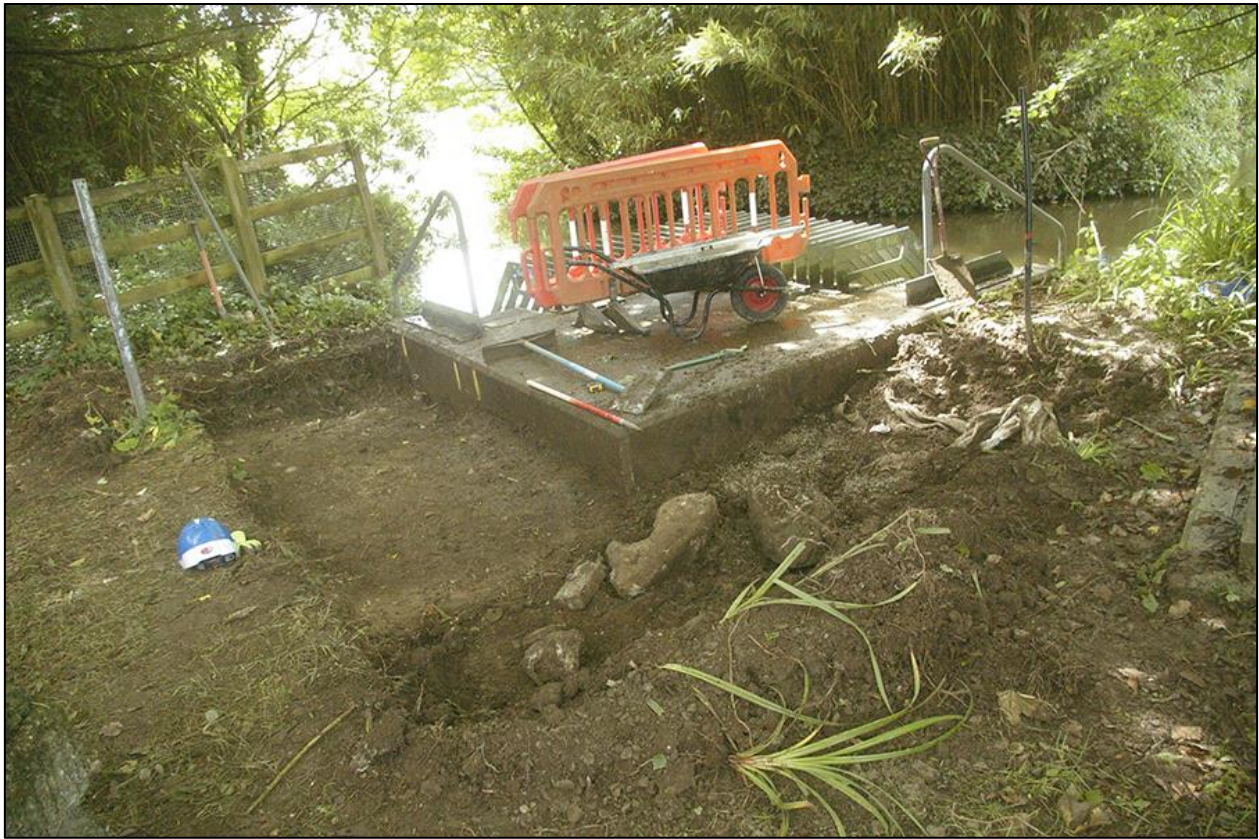
FIGURE 3: DITCHES [103] AND [105] SECTION; FROM THE NORTH-EAST (2M SCALE).
