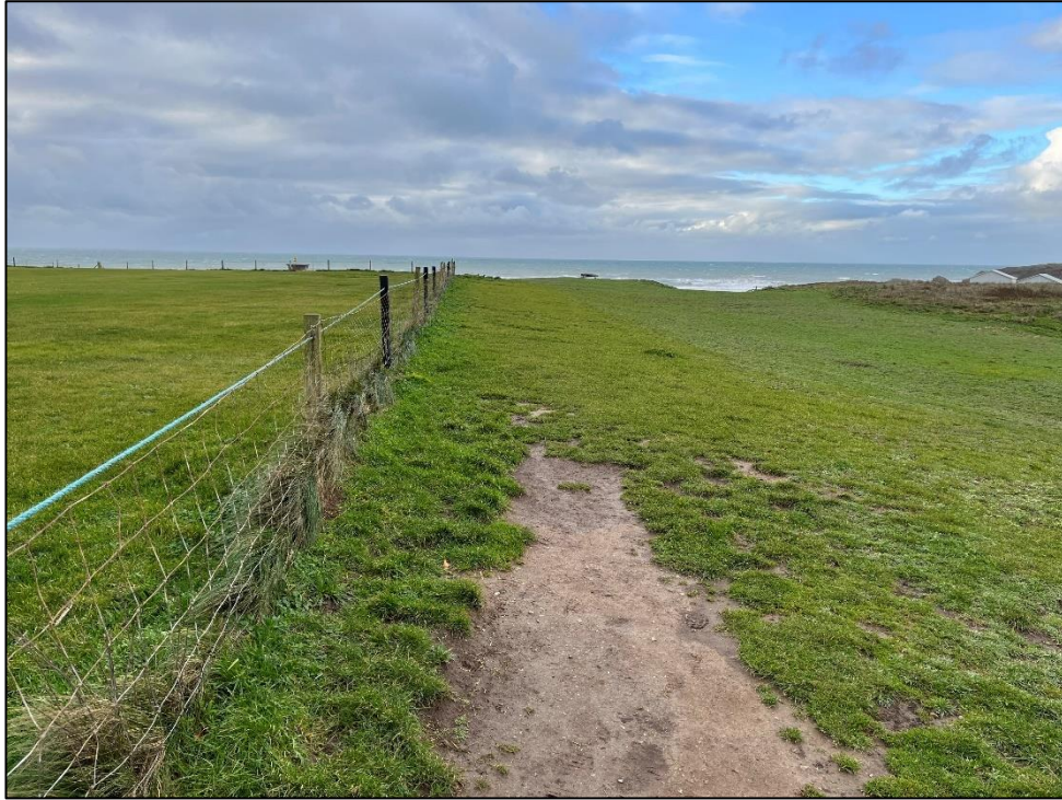
5. EROSION ALONG FENCE.
