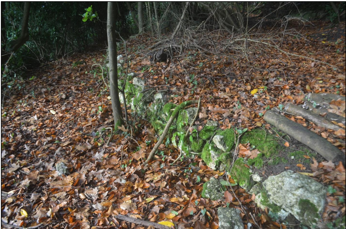
37. FURTHER EVIDENCE OF ALTERNATION OF STONE AND QUARTZ AS A WALL BUILDING MATERIAL, PATH IMMEDIATELY BEHIND ROBOROUGH HOUSE (FROM THE EAST)
