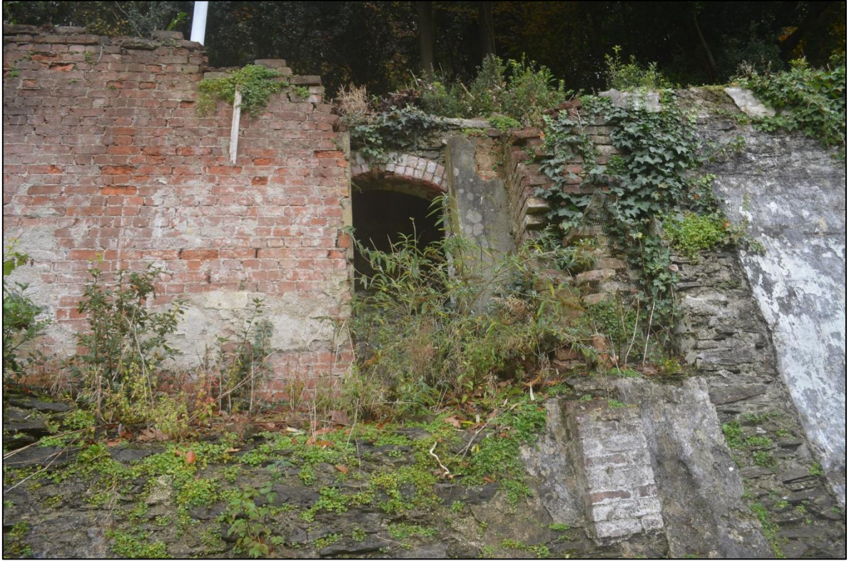
FIGURE 24: LIMITED EVIDENCE FOR PHASING WITH BRICK WALLS BUILT IN FRONT OF STONE AND BRICK ARCH (FROM THE SOUTH)
