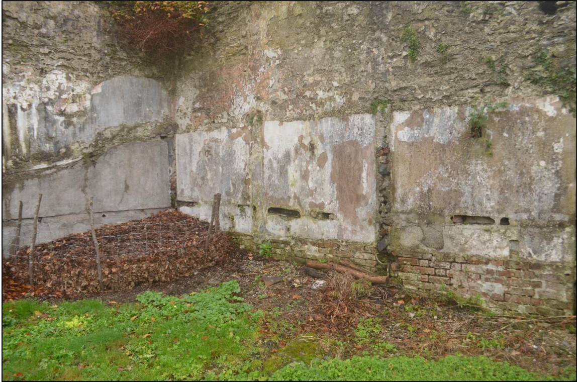
7. PART OF SURVIVING EASTERN WALL OF ROBOROUGH HOUSE SHOWING DIVISION OF THIS SPACE INTO COMPARTMENTS, POSSIBLY STABLING (FROM THE SOUTH WEST)
