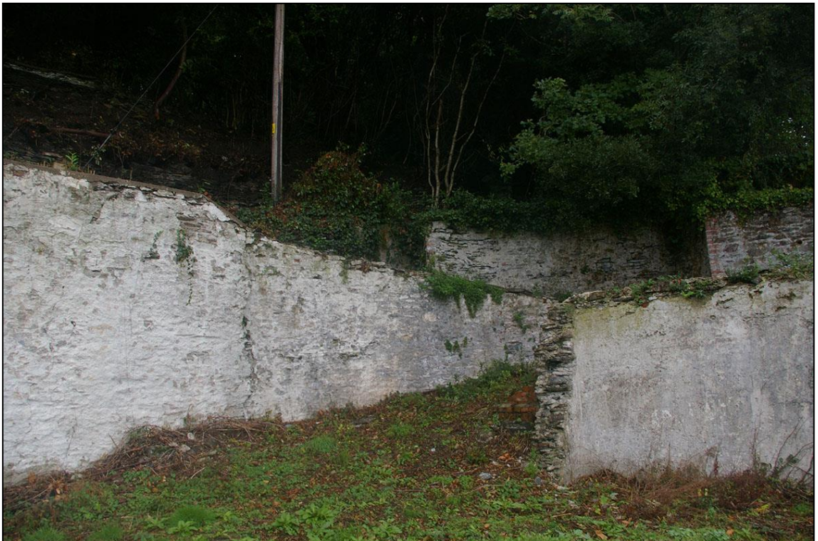
10. THE TERRACE WALLS TO THE NORTH-EAST SHOWING A CURVING SET OF STEPS RUNNING UP TOWARDS THE KITCHEN GARDENS; FROM THE WEST.
