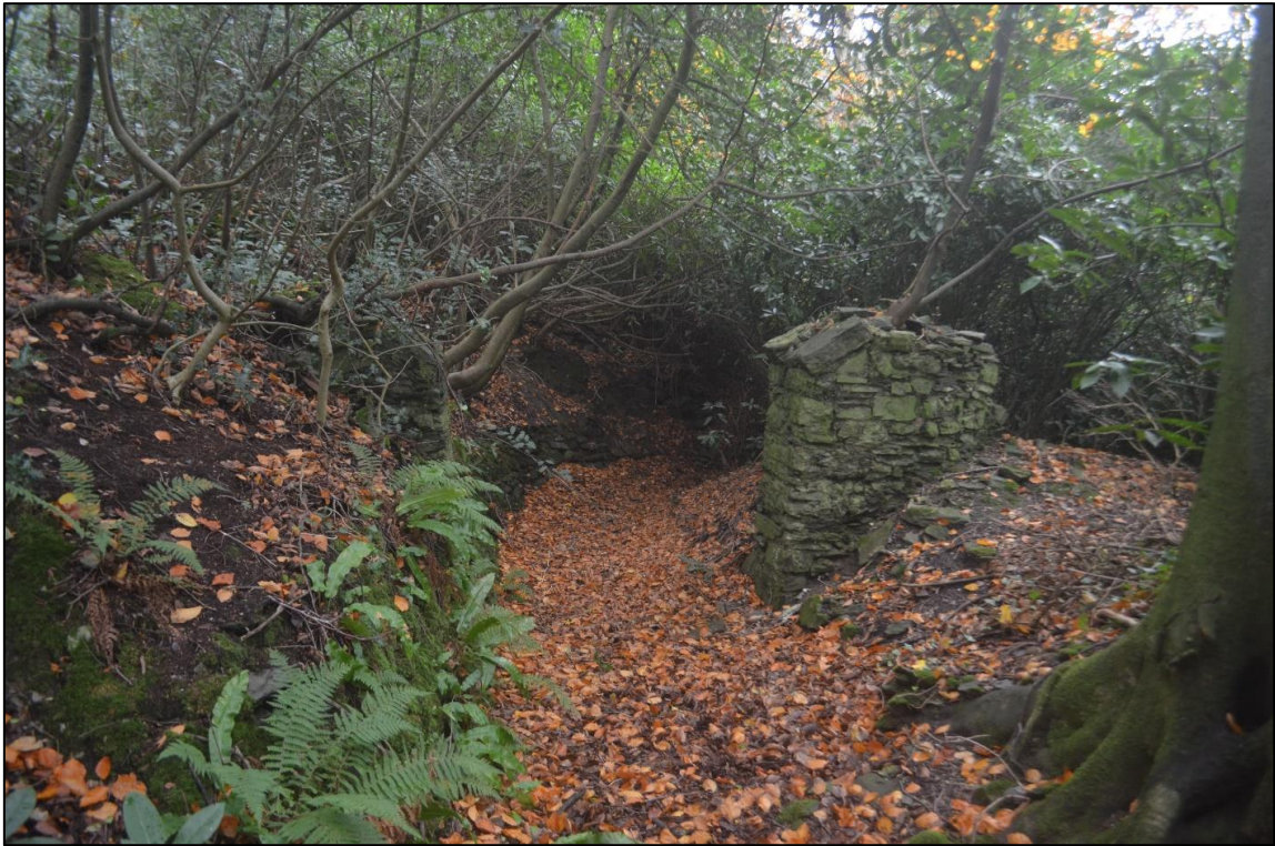
22. ENTRANCE PATH INTO WOODLAND GARDENS FROM STONE STEPS TO THE WEST OF THE HOUSE. EXTANT STONE ENTRANCE PIERS IN NEED OF VEGETATION MANAGEMENT (FROM THE NORTH WEST)
