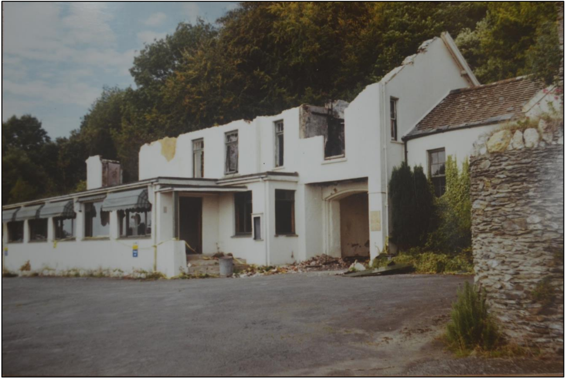
FIGURE 5: PHOTOGRAPH TAKEN AFTER THE FIRE IN THE 1990s (NDRO B513-1/126/1-5)
