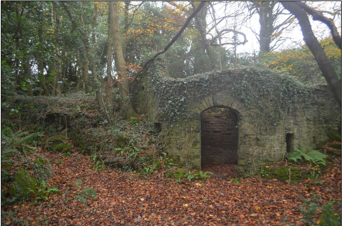
FIGURE 34: VIEW OF THE TERRACE ON WHICH THE SUMMERHOUSE WAS LOCATED, ITSELF A RUINED FOLLY FORM (FROM THE WEST)
