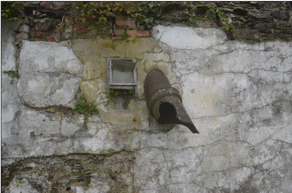
8. FITTINGS IN REAR (NORTH) WALL OF ROBOROUGH HOUSE SUGGESTING A BOILER OR RANGE IN THIS LOCATION (FROM THE SOUTH)
