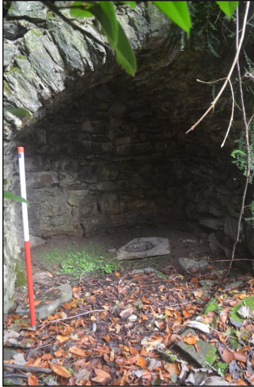
38. STONE BUILT ARCHED STRUCTURE UNDER A PATH JUST NORTH OF THE HOUSE. MAY HAVE BEEN CONSTRUCTED AT A SPRING LOCATION SHOWN ON AN EARLY 20 TH CENTURY MAP (FROM THE SOUTH)
