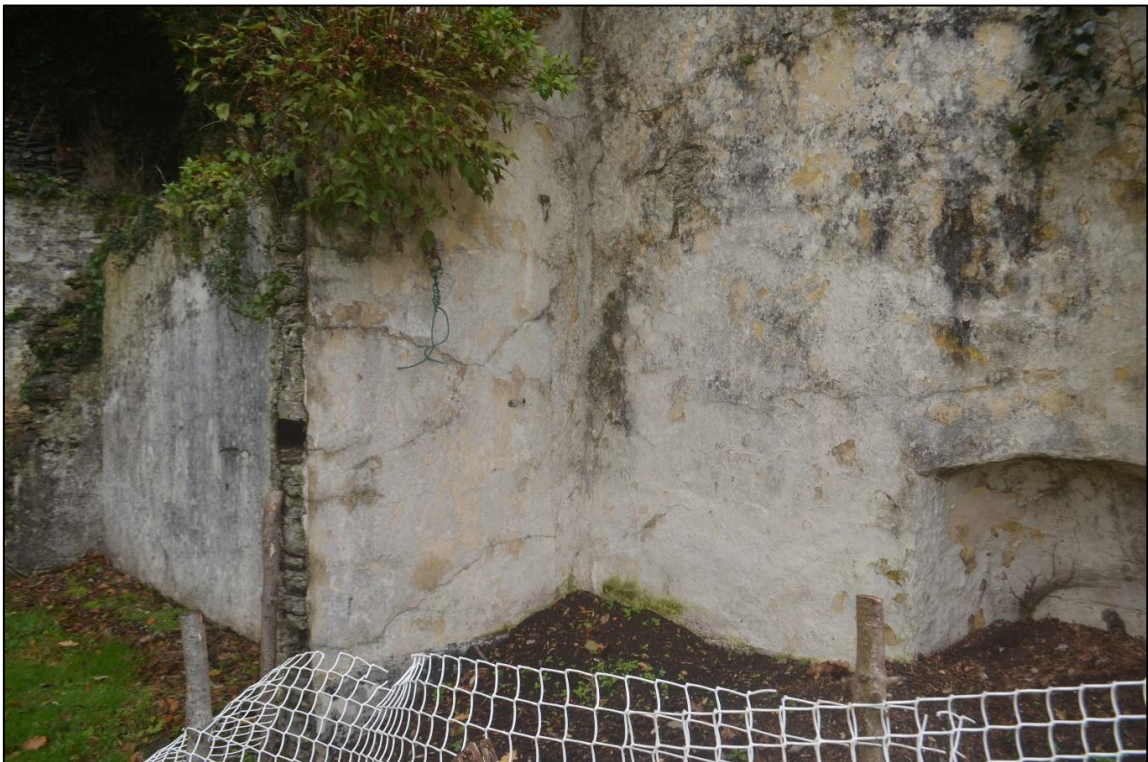
6. SURVIVING EASTERN WALL OF ROBOROUGH HOUSE; THIS AREA WAS PART OF THE MID TO LATER 19 TH CENTURY EXTENSION TO THE BUILDING AND APPEARS TO HAVE HAD A SERVICE FUNCTION WITH IRON FITTINGS STILL LOCATED IN THE WALLS (FROM THE SOUTH WEST)
