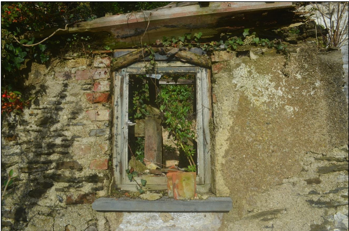
17. EVIDENCE OF ATTEMPTS TO 'RUSTICATE' THE SMALLER OF THE TWO SURVIVING GARDEN BUILDINGS IN THE FIRST GARDEN COMPARTMENT (FROM THE SOUTH)
