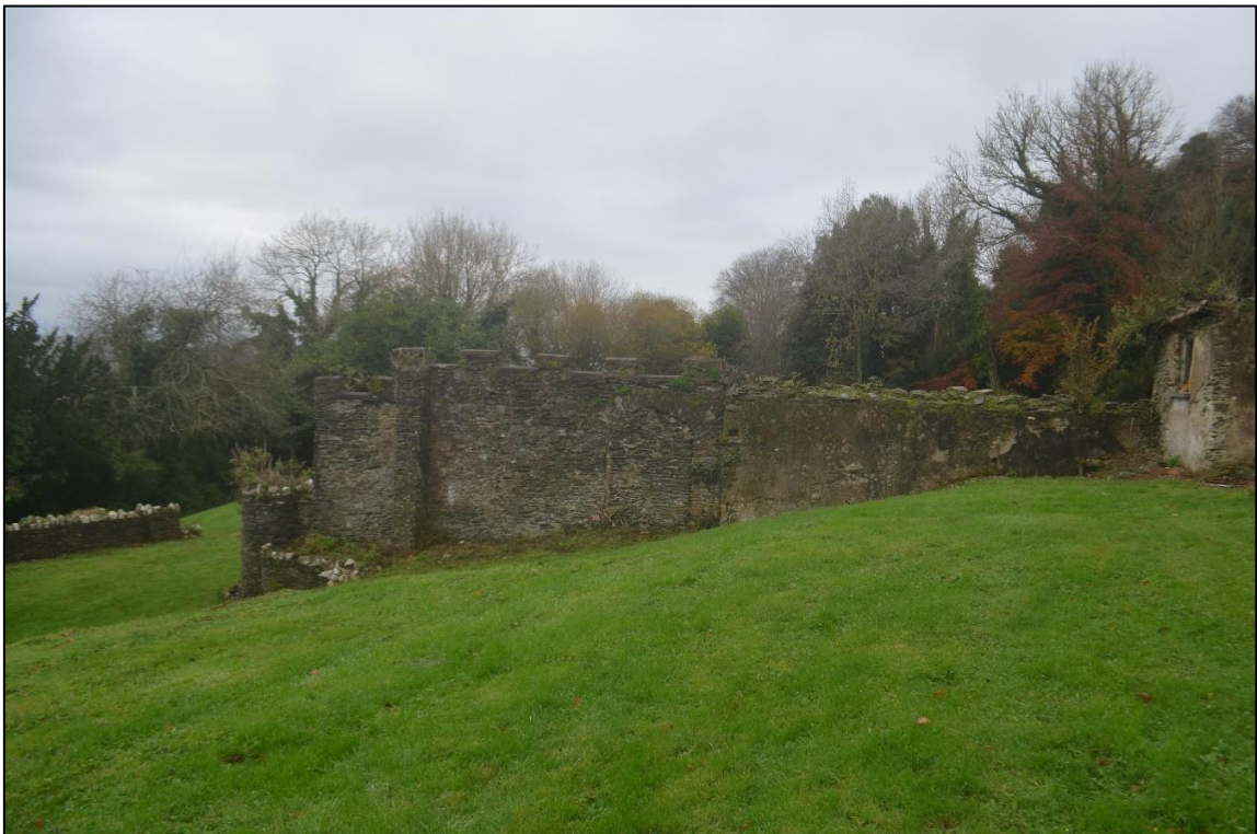
19. VIEW FROM FIRST GARDEN COMPARTMENT TOWARDS ROBOROUGH HOUSE SITE WITH CRENELATED GARDEN WALL SHOWN WITH BLOCKED ARCHED DOORWAY AND ROUND TURRET DETAILING AT TERMINUS; A COKE HOUSE WAS LABELLED ON HISTORIC MAPPING IN THIS AREA. THIS WALL IS PROPOSED FOR DEMOLITION TO ACCOMMODATE A LARGER BUILDING FOOTPRINT (FROM THE EAST)
