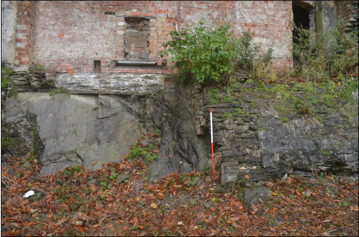
9. REAR (NORTH) WALL OF ROBOROUGH HOUSE SHOWING BRICK BUILT ONTO BEDROCK. FIREPLACE SHOWING TWO PHASES OF BLOCKING (FROM THE SOUTH)
