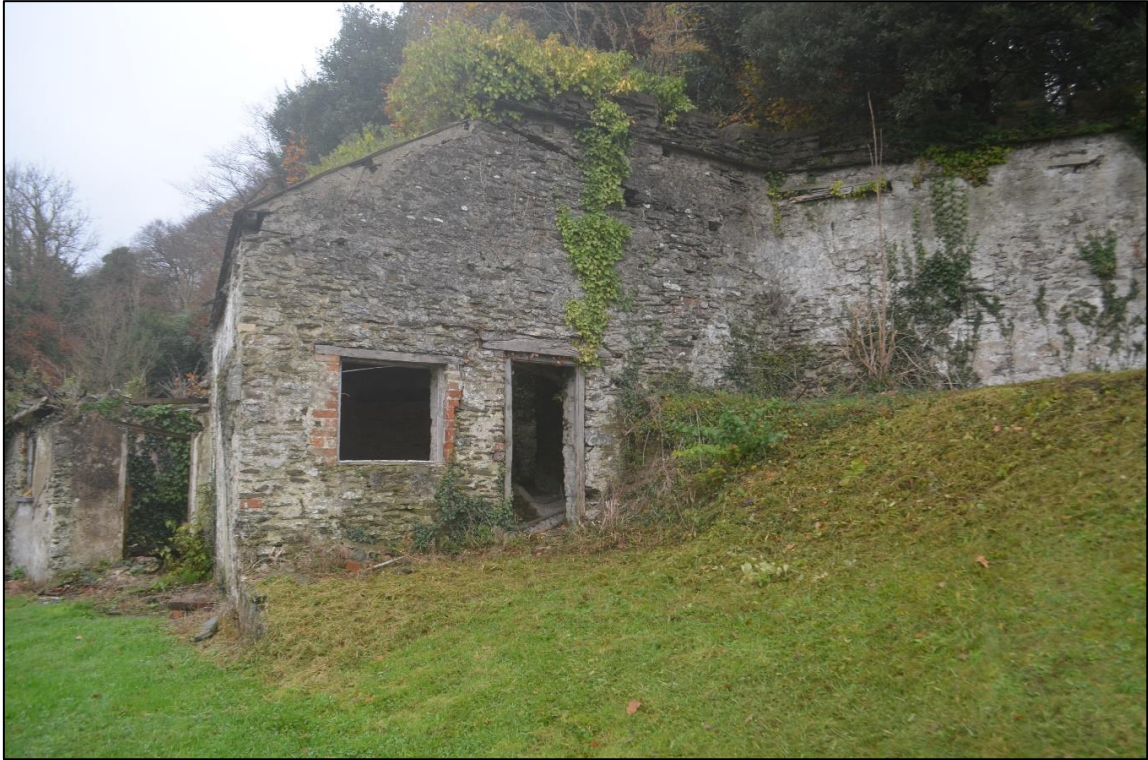
16. CRENELATED GARDEN WALL TERMINATING OVER THE ROOF OF THE LARGER SURVIVING GARDEN BUILDING (FROM THE EAST)
