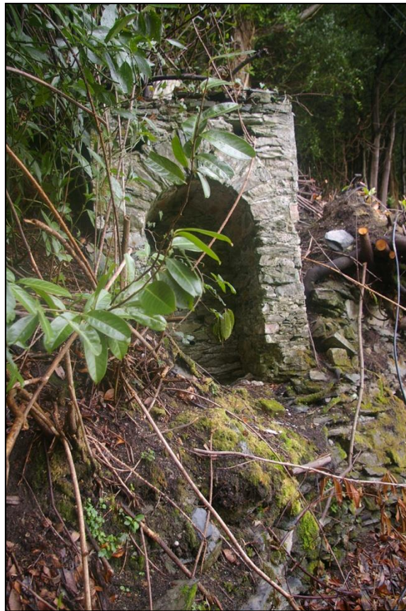
21. SMALL ARCHED WELL-HEAD TYPE STRUCTURE OVER PIPEWORK FOR WATER FEATURE AND POND BELOW, ON THE UPPER REAR TERRACE, NORTH-WEST OF THE FORMER HOUSE; FROM THE SOUTH-WEST.
