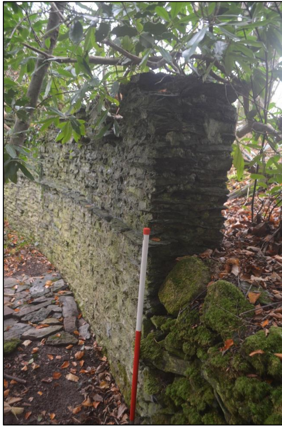
FIGURE 32: CONSTRUCTION OF THE CRENELATED WALL OF THE FOLLY (FROM THE EAST; 1M SCALE).
