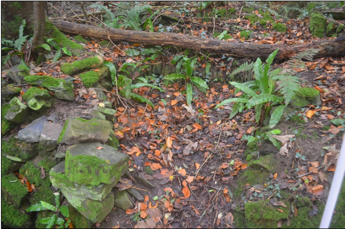
26. CIRCULAR NICHE CREATED IN STONE ALONG PATH BETWEEN SUMMERHOUSE AND FOLLY, FORMED FROM VERTICALLY SET STONE (FROM WEST)
