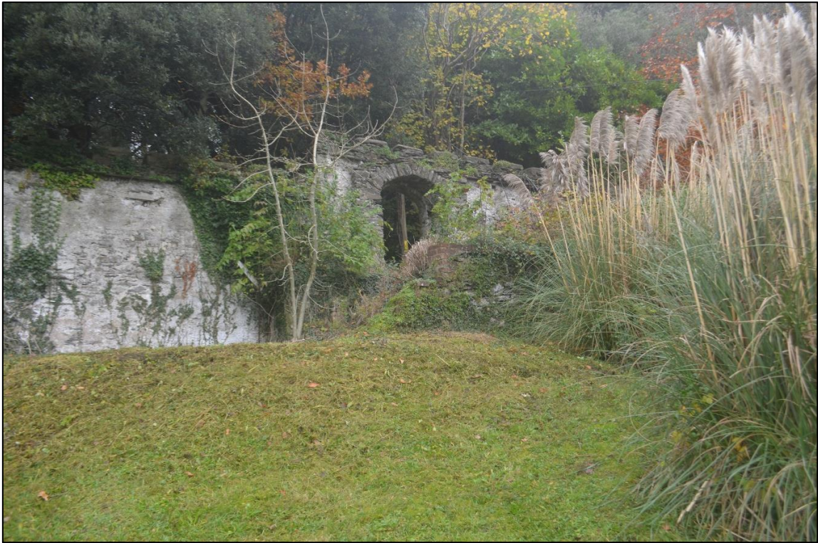
18. ARCHED DOORWAY PROVIDING ONE OF TWO ENTRANCE/EXIT POINTS TO THE GARDENS (FROM THE SOUTH)
