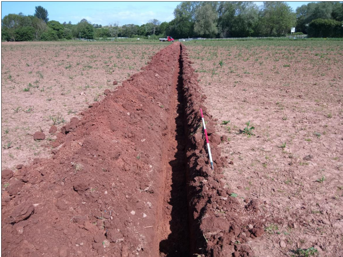
FIGURE 3: POST-EXCAVATION PLAN OF TRENCH; VIEWED FROM THE SOUTH (2M SCALE).
