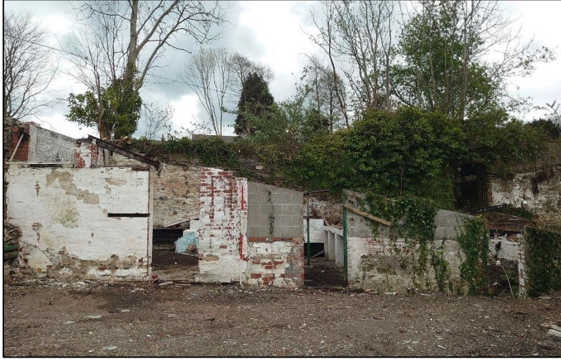
FIGURE 27: B5 FROM THE WEST, 1 x 2M SCALE.
