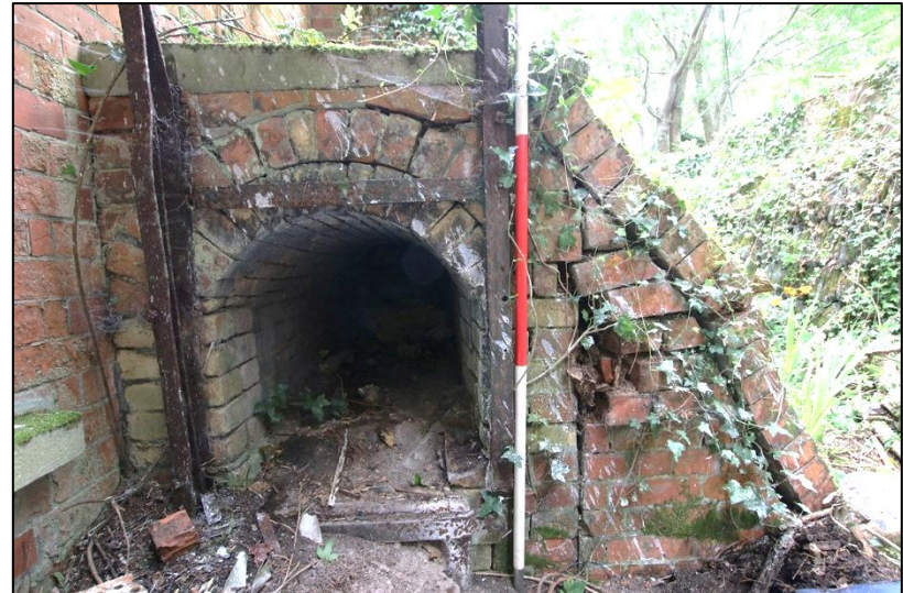
FIGURE 39: VIEW INTO THE TUBULAR EXTENSION TO THE INCINERATOR, SHOWING IN SITU SLIDING TRAY FITMENTS AND IRON DOOR.
