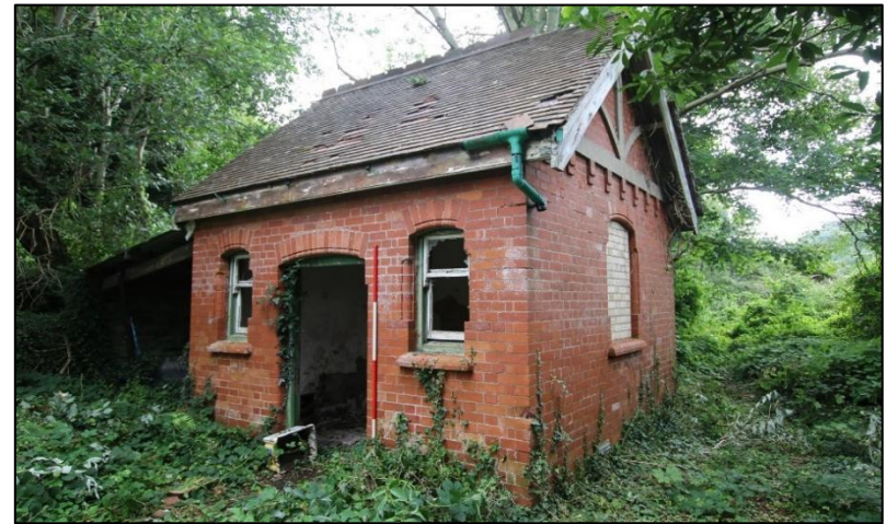
FIGURE 14: BUILDING 2, NORTH ELEVATION; FROM THE NORTH (2M SCALE).
