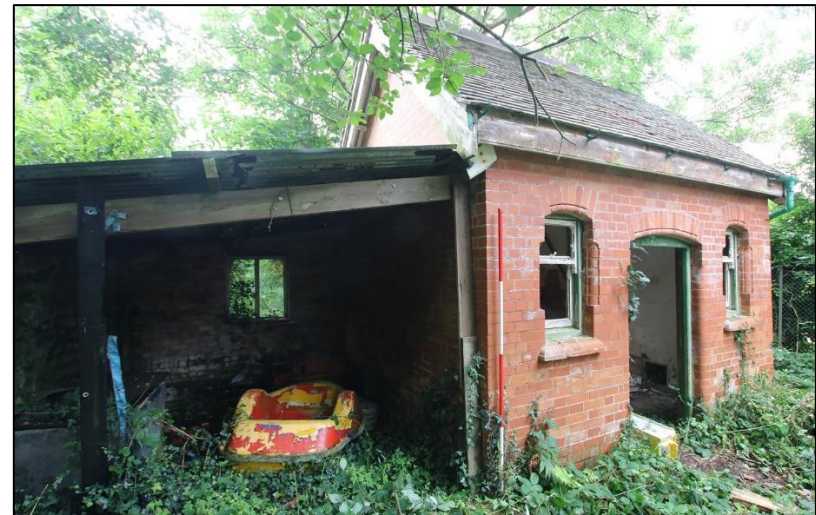
FIGURE 15: B2, AND LEAN-TO B2A, FROM THE NORTH-EAST (2M SCALE).
