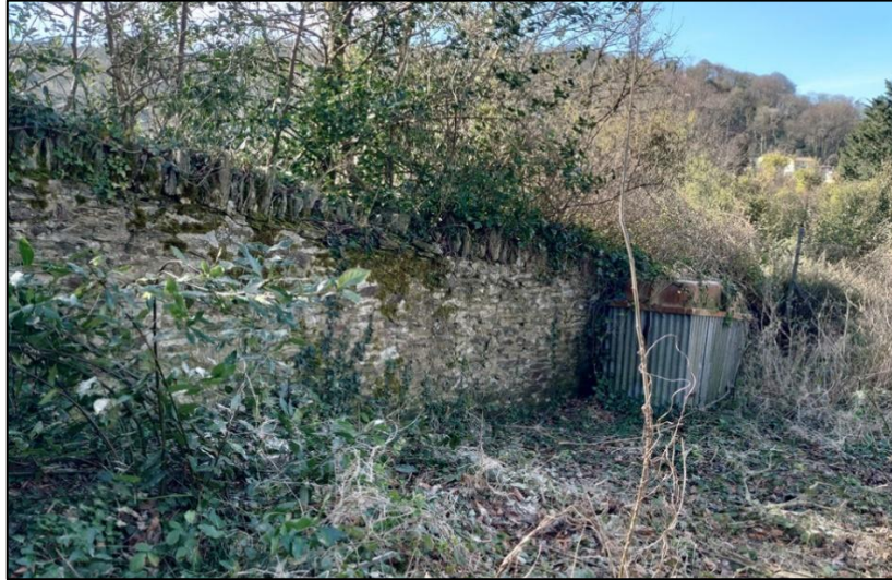
FIGURE 35: THE SOUTH GARDEN WALL; FROM THE NORTH-EAST.
