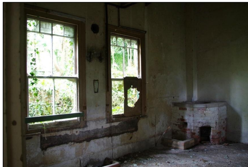
FIGURE 9: THE LAUNDRY ROOM WITH COPPER IN SITU; FROM THE NORTH-WEST.
