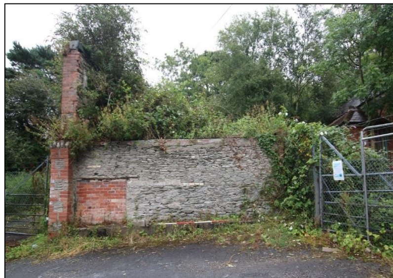
FIGURE 30: THE GARDEN WALL TO THE NORTH OF THE SITE, WHERE AN OPENING HAS BEEN FORCED FOR THE ADJACENT CARE HOME SITE (2M SCALE) FROM THE EAST.
