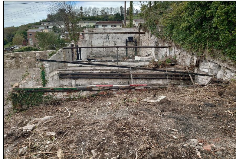
FIGURE 26: THE ROOFLESS AND STRIPPED OUT B5, OF THREE UNITS, 1 x 2M SCALE.
