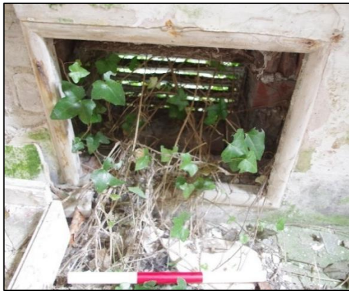
FIGURE 13: LARGE AIR VENTS IN BUILDING 2 (0.3M SCALE).
