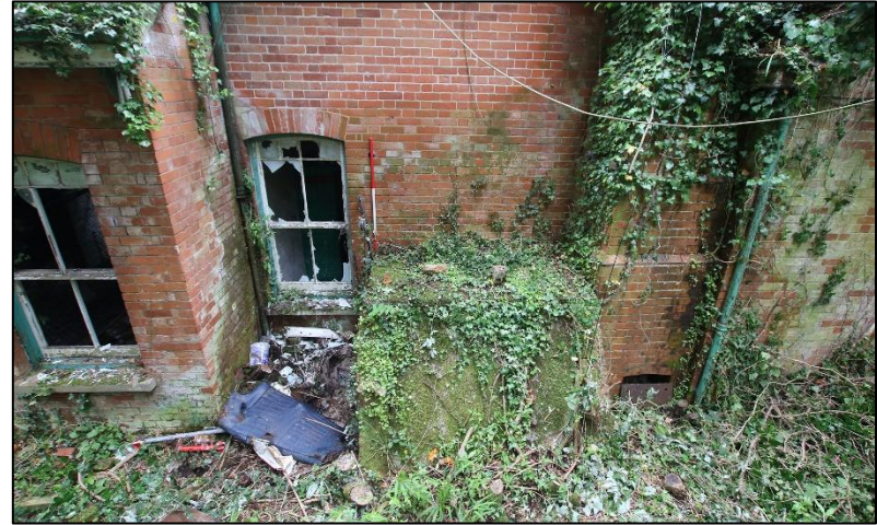
FIGURE 38: THE EXTENSION TO THE INCINERATOR WHICH APPEARS TO HAVE BEEN ADDED ONTO THE CHIMNEY, THE INTERIOR OPENING FOR LAUNDRY BEING BLOCKED, 2M SCALE.
