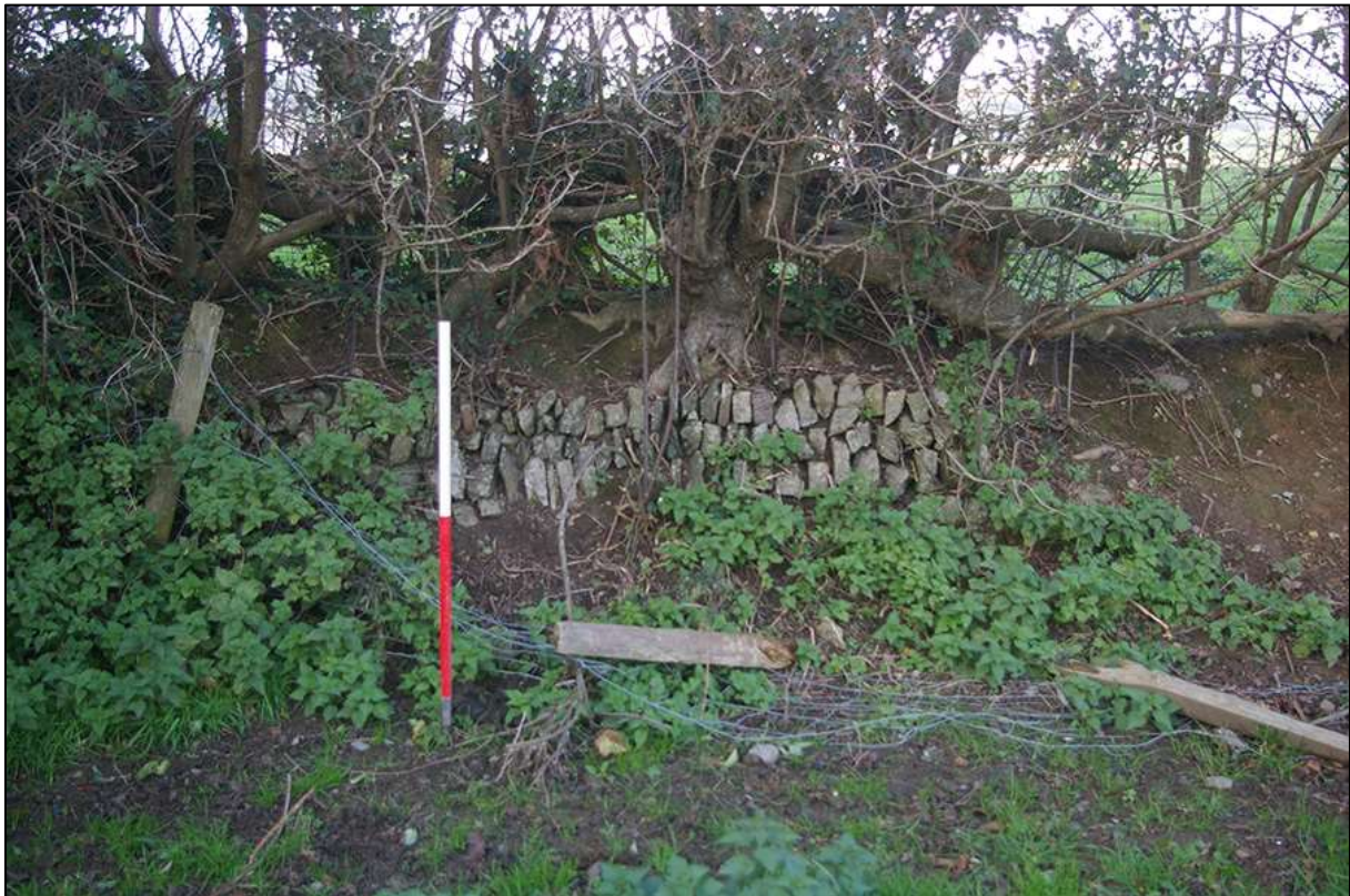
16. DETAIL OF THE NORTHERN STONE-FACED HEDGEBANK BOUNDARY TO F2; VIEWED FROM THE SOUTH (1M SCALE).
