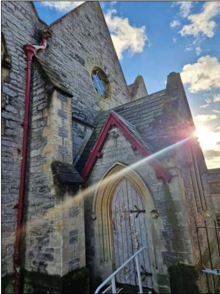
3. PORCH TO WEST OF CHURCH, WITH ROSE WINDOW ABOVE.
