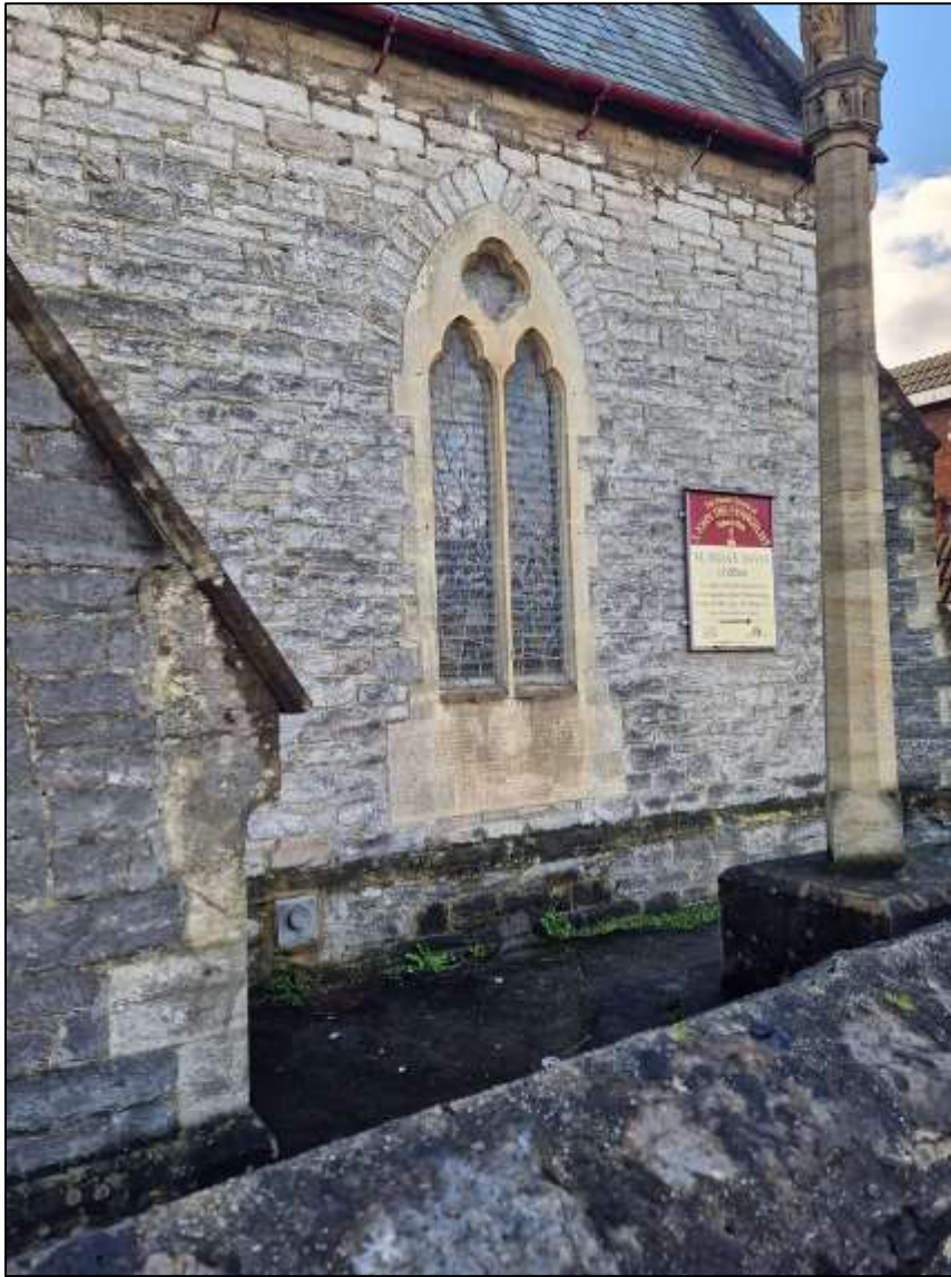
4. WAR MEMORIAL WINDOW OF C.1920 IN NORTH ELEVATION.
