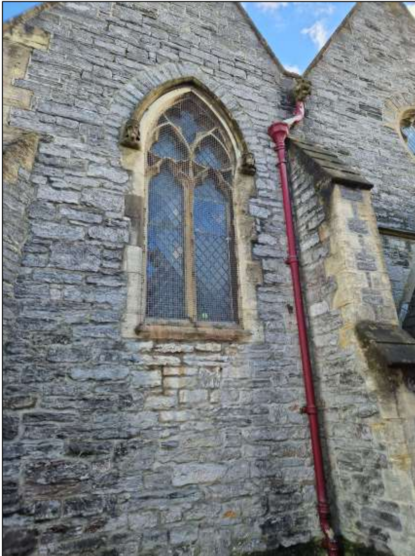
2. WINDOW WITH GROTESQUES TO WEST ELEVATION OF CHURCH.
