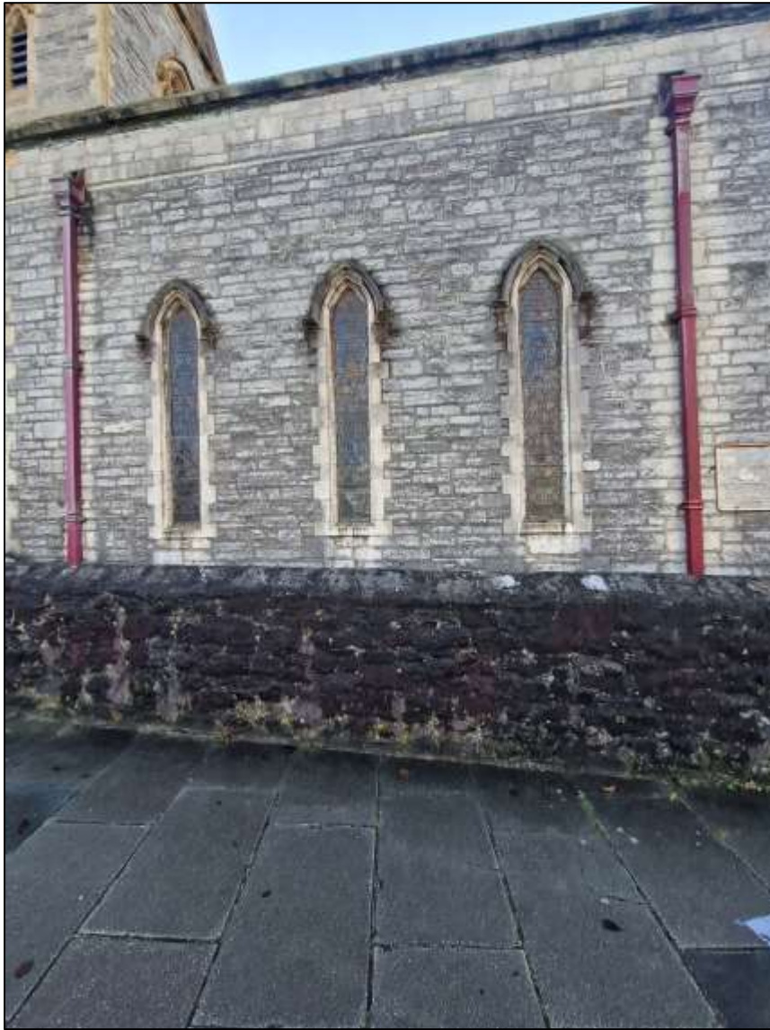
6. REPLACEMENT LANCET WINDOWS TO LADY CHAPEL, FROM THE NORTH.
