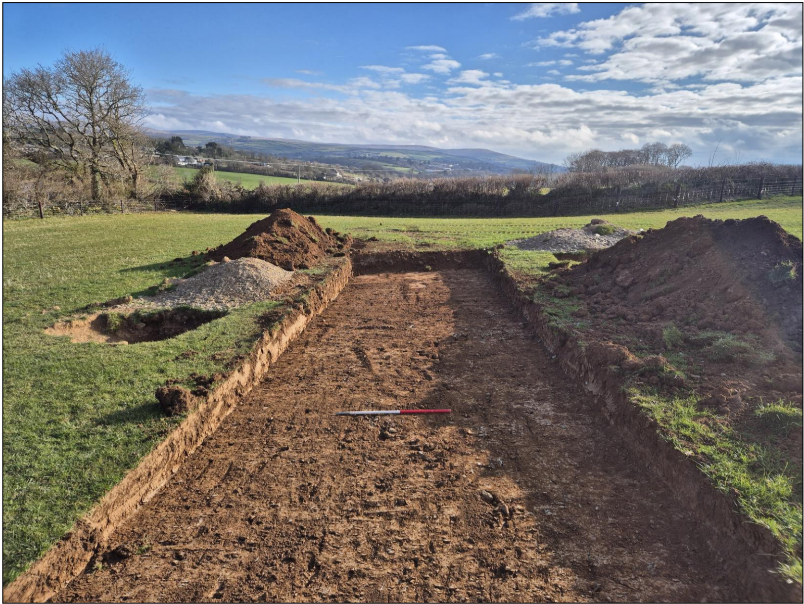
FIGURE 2: PROPOSED DRAINAGE AREA, POST-EXCAVATION; VIEWED FROM THE WEST (1M SCALE).
