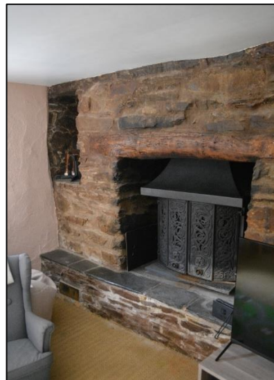
7. MAIN HOUSE PLAYROOM. DETAIL OF FIREPLACE AND ALCOVE. FROM NORTH EAST
