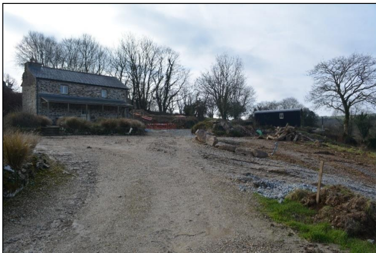
36. NORTHERN ELEVATION OF COTTAGE SHOWN IN ITS SETTING WITH APPROACH FROM WEST
