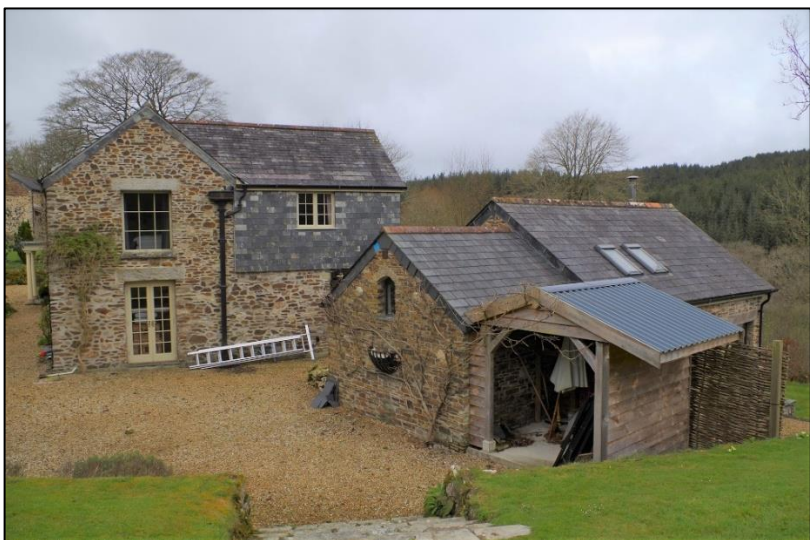
22. EAST ELEVATION OF MAIN HOUSE AND MILL BUILDING
