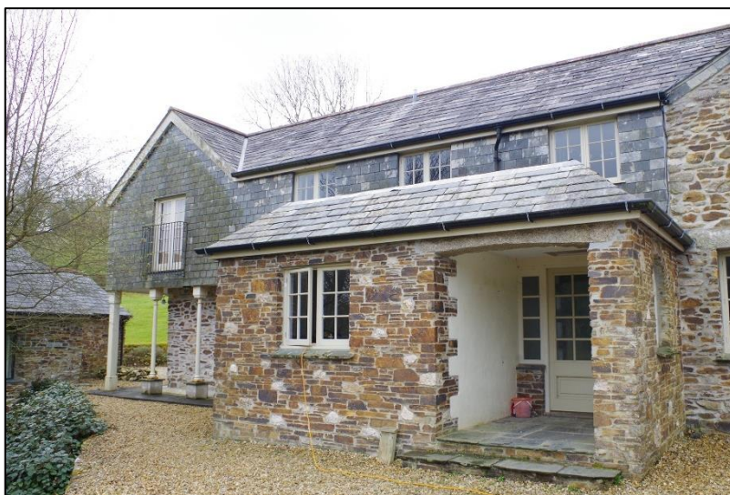
18. MAIN HOUSE NORTHERN ELEVATION WITH PORCH AND 21 ST C JETTIED EXTENSION
