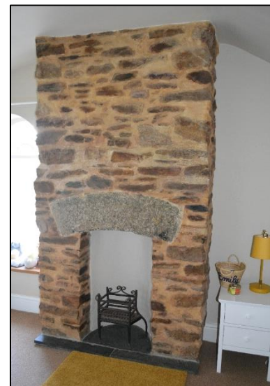
11. MAIN HOUSE, DETAIL OF FIREPLACE IN UPSTAIRS BEDROOM, ABOVE LOUNGE, WITH ROUNDED BACK TO HEARTH AND SHAPED LINTEL.
