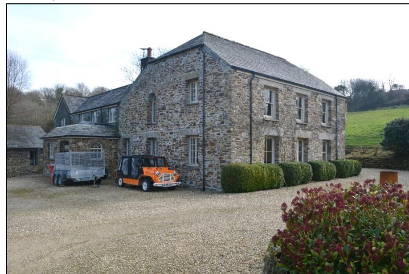
16. MAIN HOUSE, WEST AND NORTH ELEVATIONS. FROM THE SOUTH EAST.
