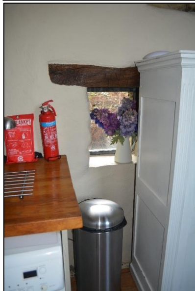
26. ONE OF OPENINGS IN W ELEVATION OF MILL FOR MACHINERY
