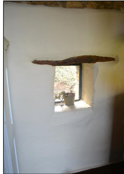
27. SECOND OPENING IN W ELEVATION OF MILL FOR MACHINERY.
