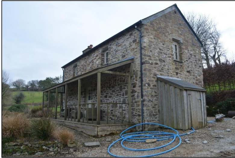
32. NORTHERN AND WESTERN ELEVATIONS OF COTTAGE SHOWING VERANDA
