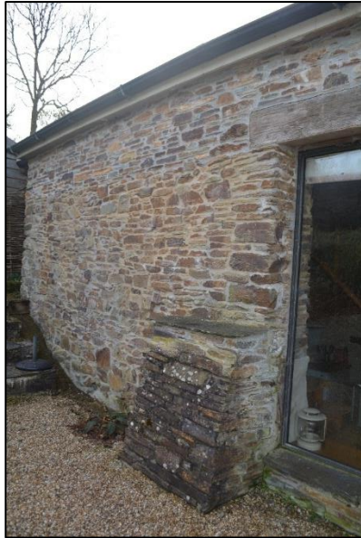
25. MILL BUILDING SHOWING RAISE WITH CLEAR BUILD LINE, FROM THE EAST
