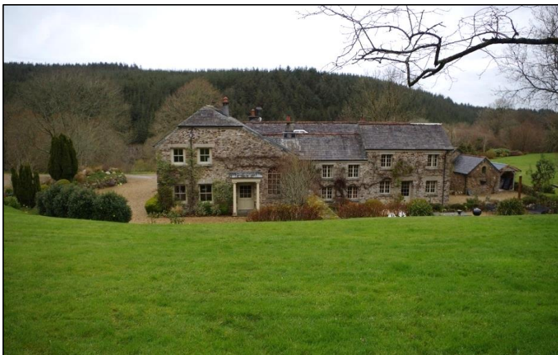
21. SETTING OF MAIN HOUSE VIEWED FROM THE SOUTH WITH MILL BUILDING ON RIGHT.
