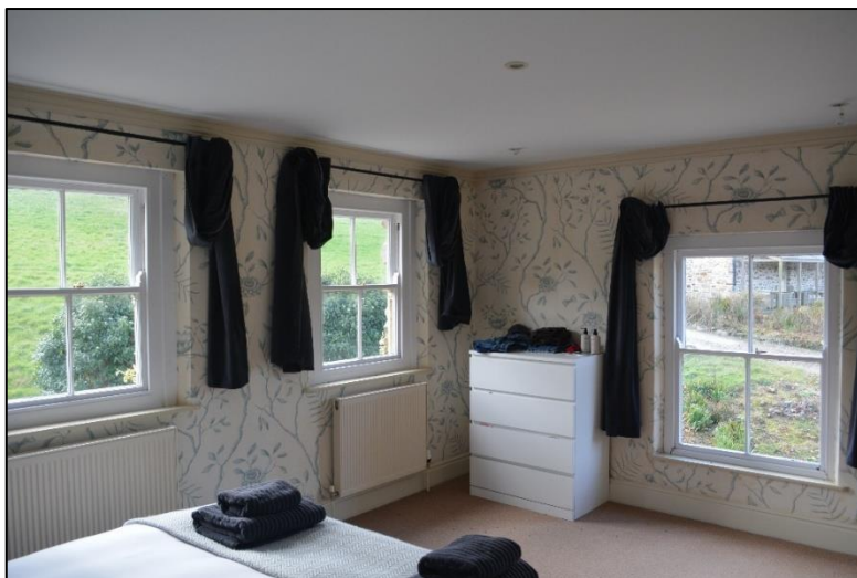
9. MAIN HOUSE, BEDROOM TO WEST OF STAIRCASE. FROM SOUTH EAST.
