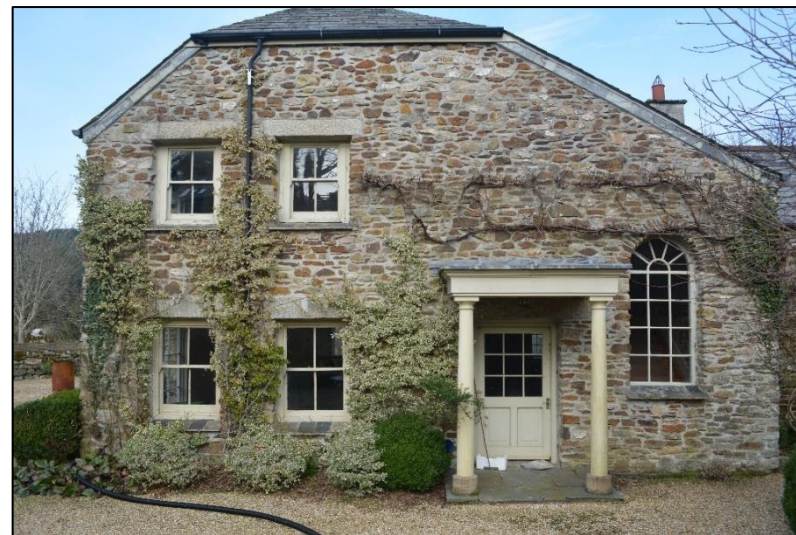
19. WESTERN END OF SOUTH ELEVATION SHOWING PORCH WITH DOOR TO LOUNGE
