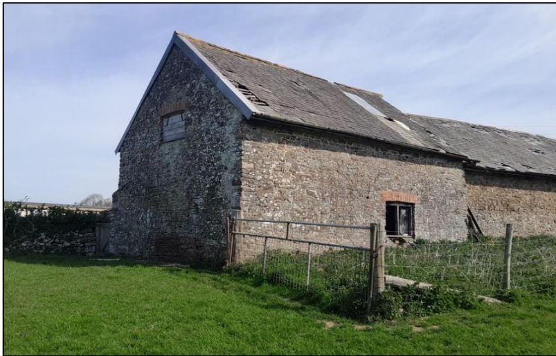
FIGURE 10: THE WEST AND SOUTH ELEVATION OF B1; FROM THE SOUTH-WEST.
