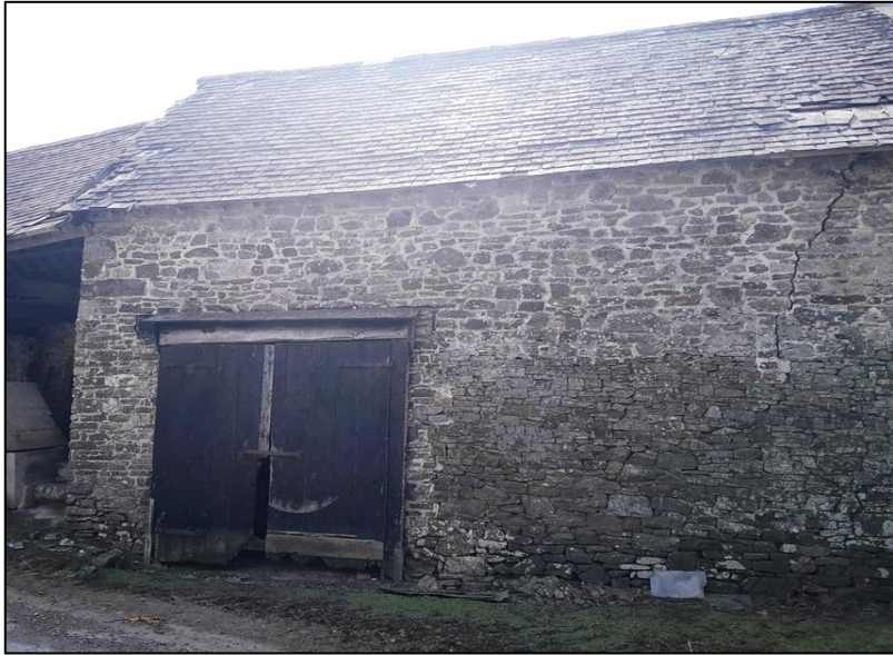
FIGURE 9: THE NORTH WALL OF B1; FROM THE NORTH-WEST.
