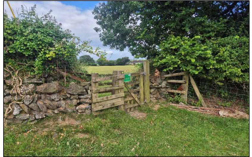
FIGURE 17: THE GATE IN THE WESTERN END OF THE SOUTHERN BOUNDARY; VIEWED FROM THE NORTH-EAST (NO SCALE).
