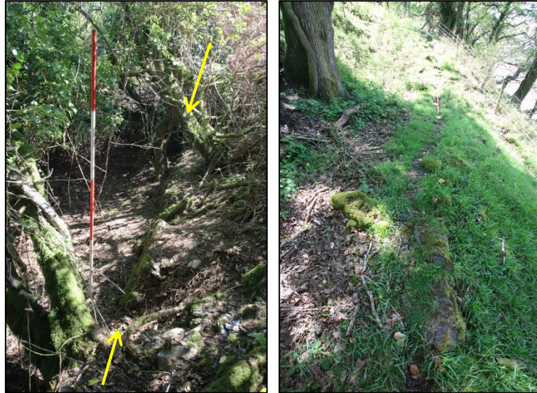
LEFT FIGURE 58: THE WALL EAST OF THE CRUSHER HOUSE; FROM THE WNW (SCALE 2M).
