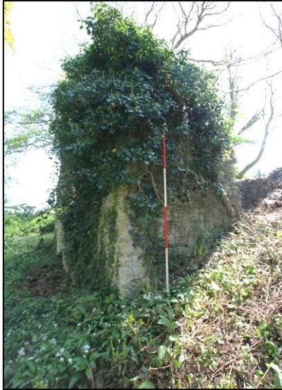
FIGURE 34: THE NORTH-WEST CORNER; FROM THE NORTH-WEST (SCALE 2M).
