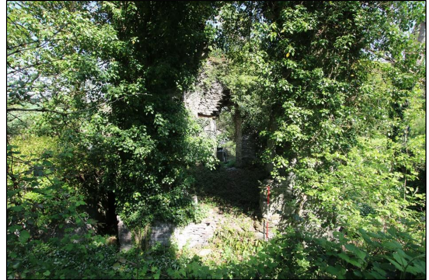
FIGURE 16: THE SOUTH-WEST ELEVATION (CYLINDER DOOR); FROM THE SOUTH-WEST (SCALE 2M).
