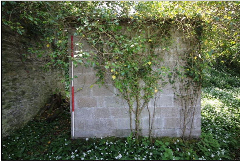
FIGURE 42: NORTH-EAST ELEVATION; FROM THE NORTH-EAST (SCALE 2M).
