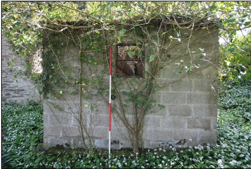
FIGURE 43: NORTH-WEST ELEVATION; FROM THE NORTH-WEST (SCALE 2M).
