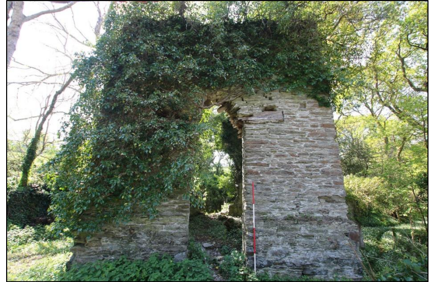
FIGURE 14: THE NORTH-EAST ELEVATION (BOB WALL); FROM THE NORTH-EAST (SCALE 2M).
