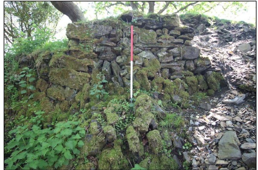
FIGURE 57: AS ABOVE, SHOWING DETAIL OF THE RAISE; FROM THE NORTH (SCALE 1M).
