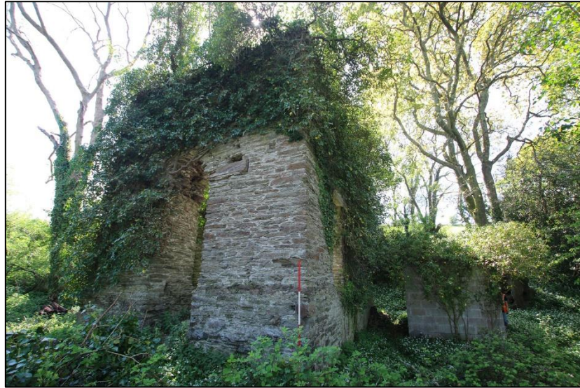
FIGURE 22: NORTH-WEST AND NORTH-ELEVATIONS; FROM THE NNE (SCALE 2M).
