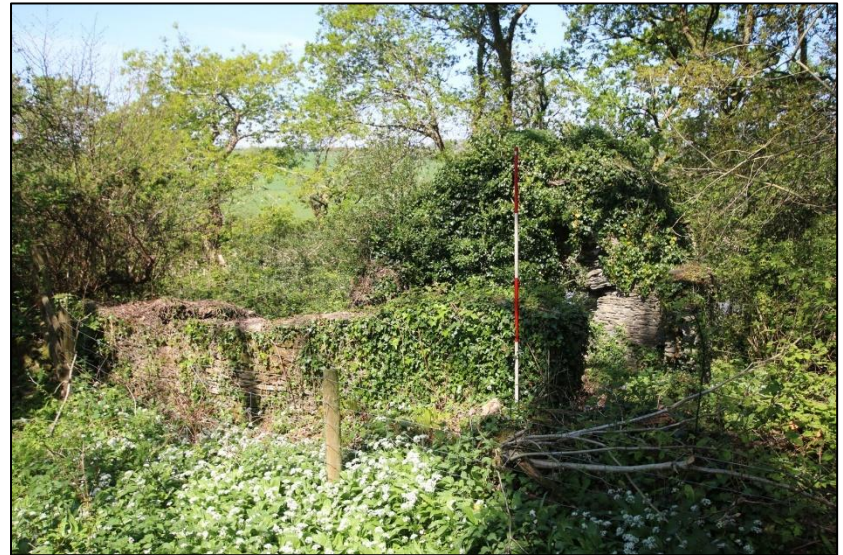
FIGURE 37: THE SOUTH-EAST CORNER; FROM THE SSE (SCALE 2M).
