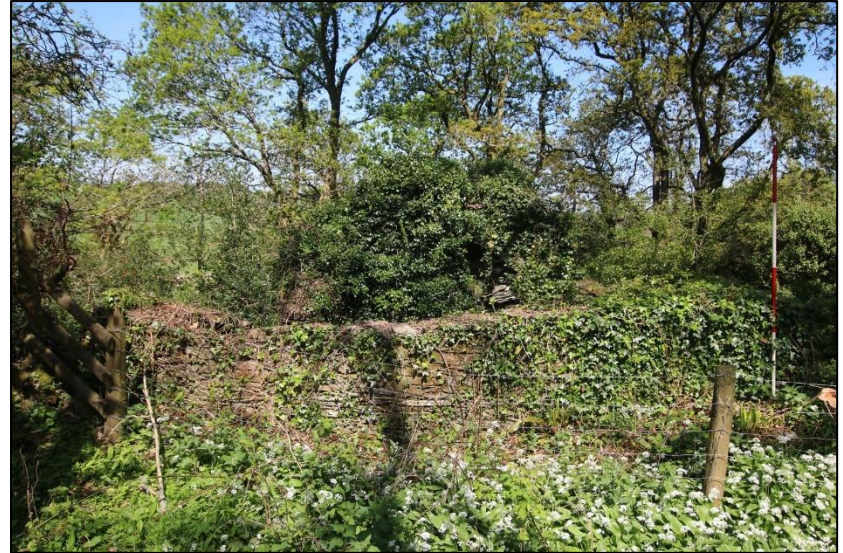
FIGURE 36: THE SOUTH GABLE WALL; FROM THE SOUTH (SCALE 2M).
