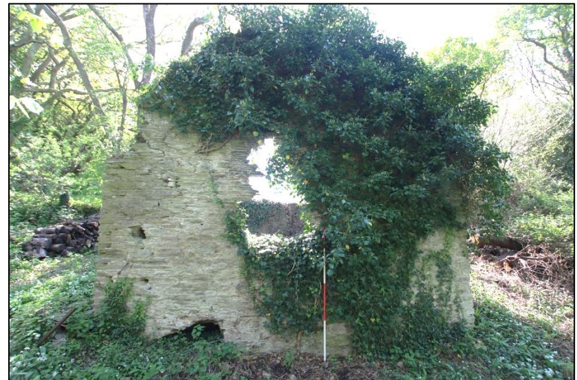
FIGURE 33: THE NORTH GABLE; FROM THE NORTH (SCALE 2M).
