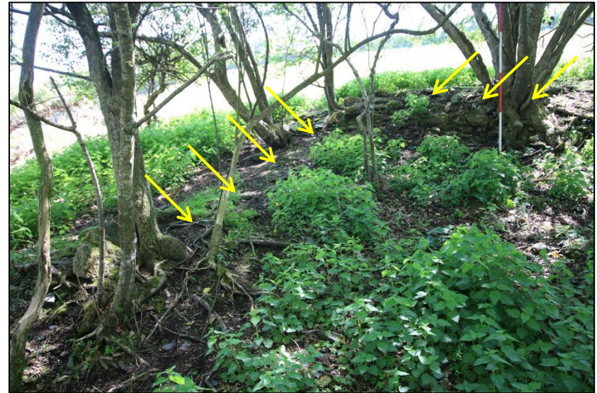
FIGURE 53: THE EAST SIDE OF THE TERRACE, INDICATING THE WALLS; FROM THE NORTH-WEST (SCALE 2M).
