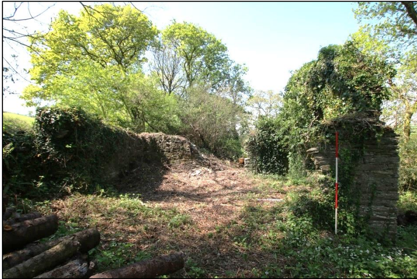
FIGURE 31: THE SMITHY; FROM THE EAST (SCALE 2M).
