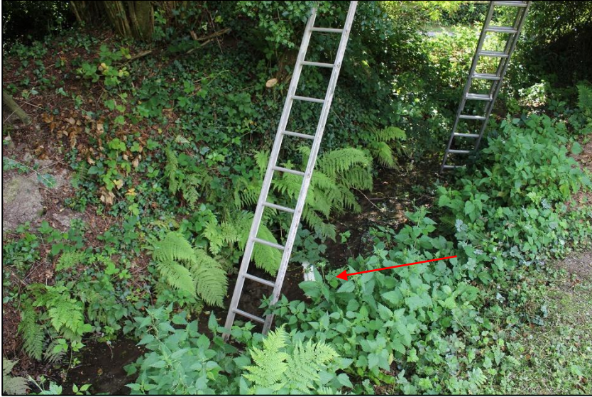
65. PLASTIC PIPE IN DRAIN/STREAM IN THE SOUTH-WEST CORNER OF THE SITE, ASSOCIATED WITH ON-SITE DRAINAGE; VIEWED FROM THE NORTH-EAST (NO SCALE).
