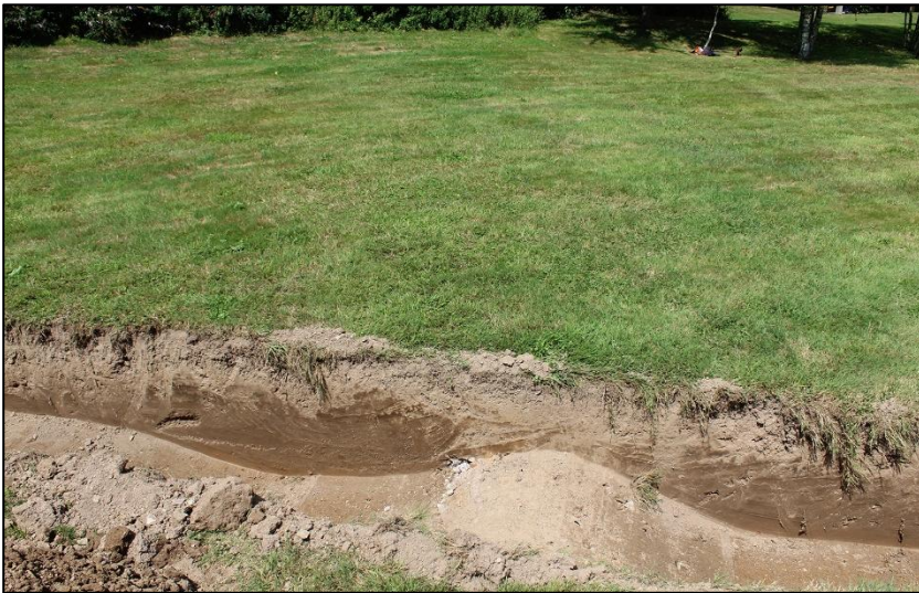
18. PLASTIC DRAIN IN TRENCH #3; VIEWED FROM THE SOUTH-WEST (NO SCALE).
