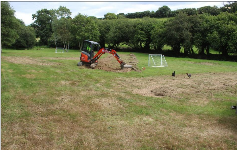
66. SOUTHERN AREA DURING BACK-FILLING; VIEWED FROM THE NORTH-WEST (NO SCALE).
