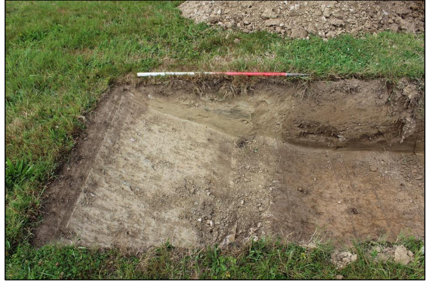
39. CUT FOR PLASTIC PIPE IN TRENCH #5; VIEWED FROM THE SOUTH-SOUTH-EAST (1M SCALE).
