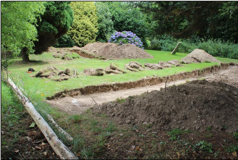
50. VIEW OF TRENCHES #7 AND #8; VIEWED FROM THE NORTH-WEST (NO SCALE).
