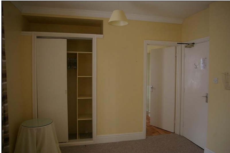
FIGURE 20: BEDROOM 32A, WITH SOME SURVIVING SKIRTING BOARDS AND PLASTER CORNICE, AS WELL AS REMAINS OF TRUNCATED WEST GABLE END STACK; FROM THE SOUTH-EAST.
