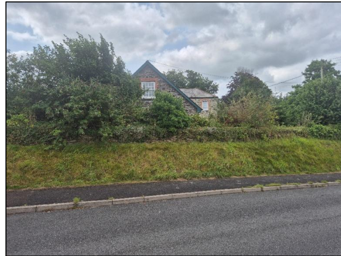
16. TREVANION HOUSE, FROM THE CULVERY; FROM THE NORTH.
