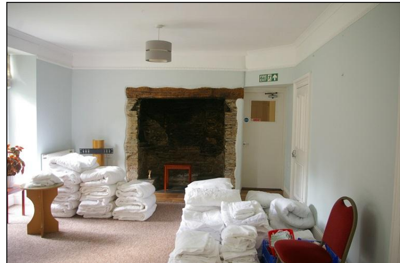
FIGURE 15: THE MAIN FORMAL LIVING SPACE IN THE MAIN RANGE, R3, WITH HISTORIC FIREPLACE; FROM THE EAST.
