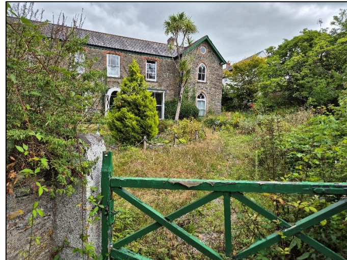
8. VIEW FROM THE GATE ACROSS THE GARDEN TO TREVANION HOUSE, THIS IS THE PROPOSED DRIVEWAY ENTRANCE; FROM THE SOUTH-WEST.
