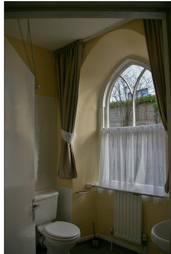
FIGURE 19: THE GOTHIC WINDOWS IN THE CROSS-WING; FROM THE SOUTH-WEST.
