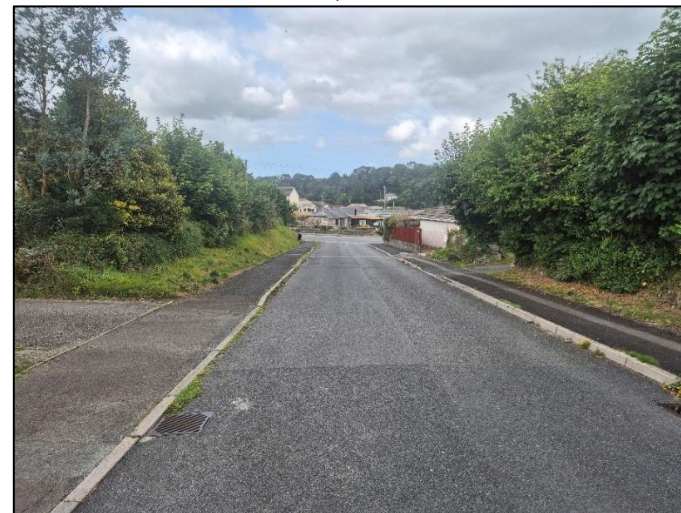
12. VIEW DOWN THE CULVERT TO THE CONVERTED TREVANION BARTON; FROM THE EAST.
