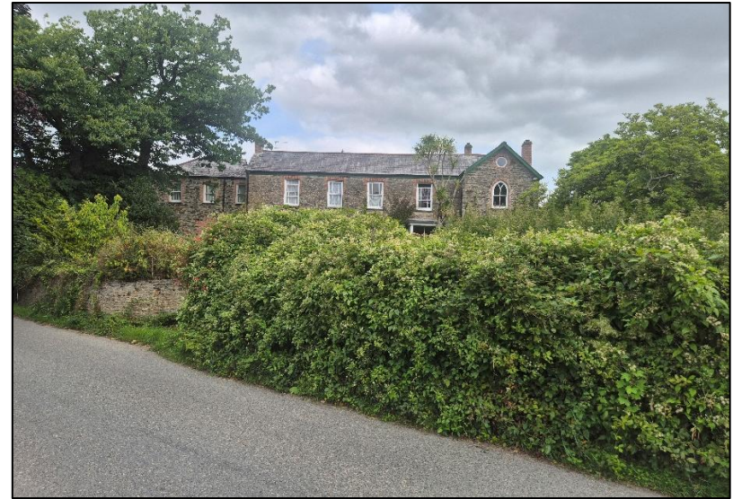
FIGURE 11: VIEW TOWARDS TREVANION HOUSE, ACROSS THE FRONT GARDEN PROPOSED FOR DEVELOPMENT.
