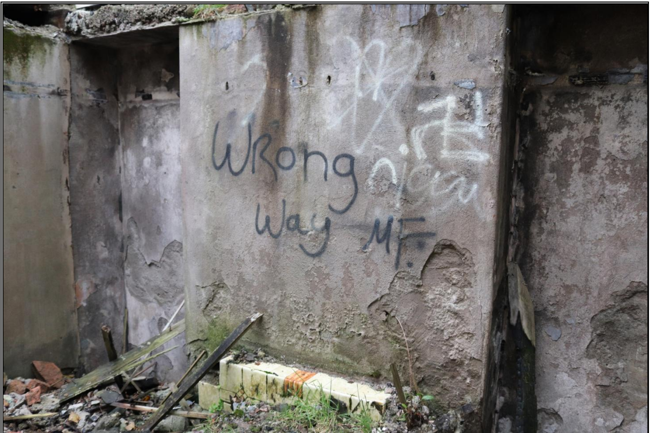
47. STACK TO R2, FROM THE NW.
