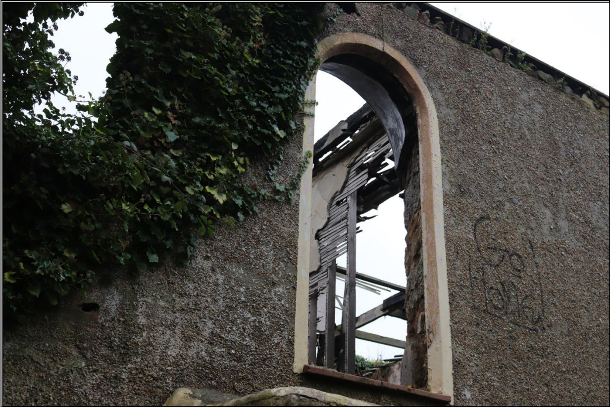
12. THE STAIR WINDOW ABOVE PORCH.
