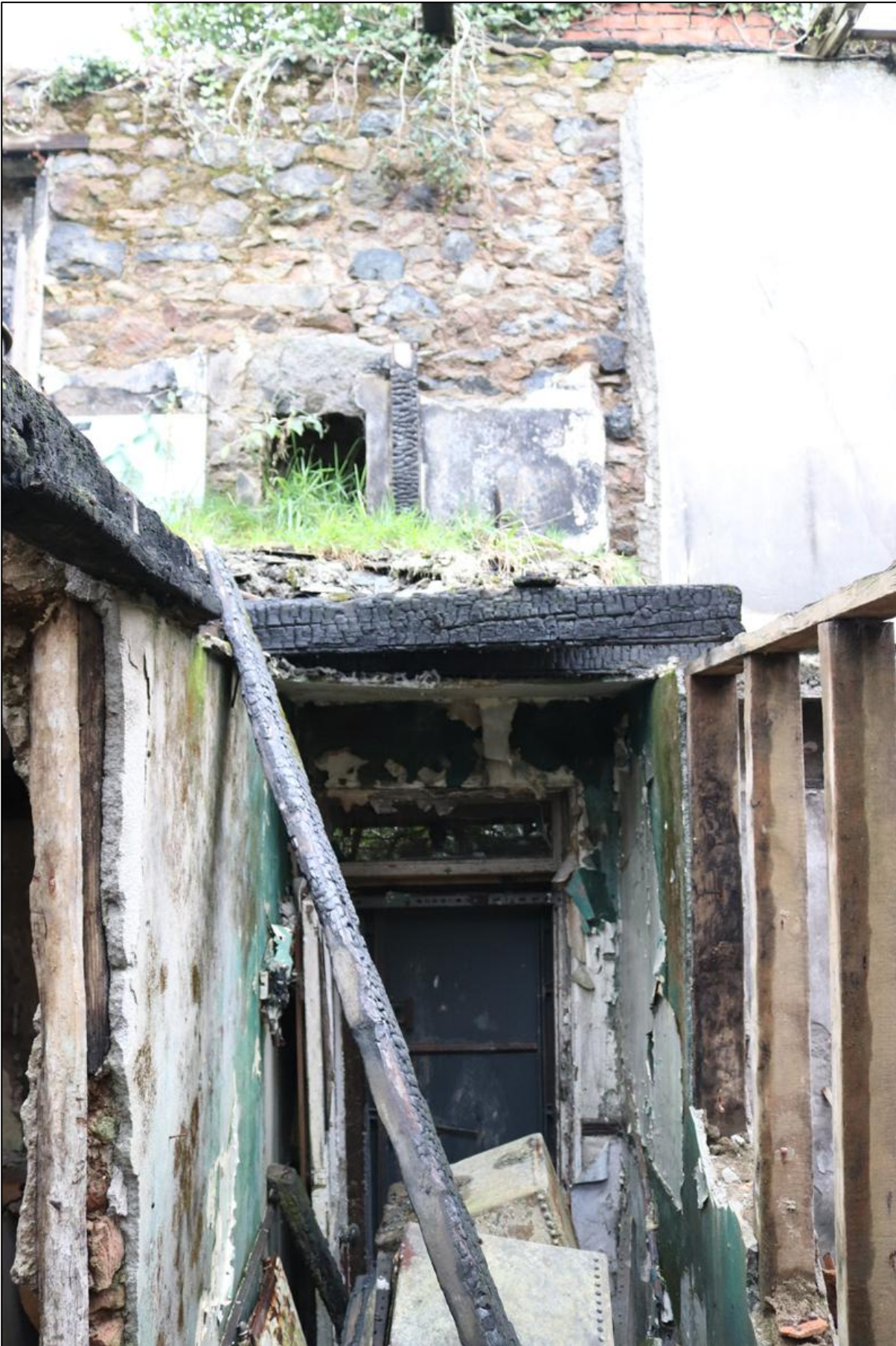
52. LOOKING TO FORMER FORMAL ACCESS FROM STAIR HALL TO NORTH.
