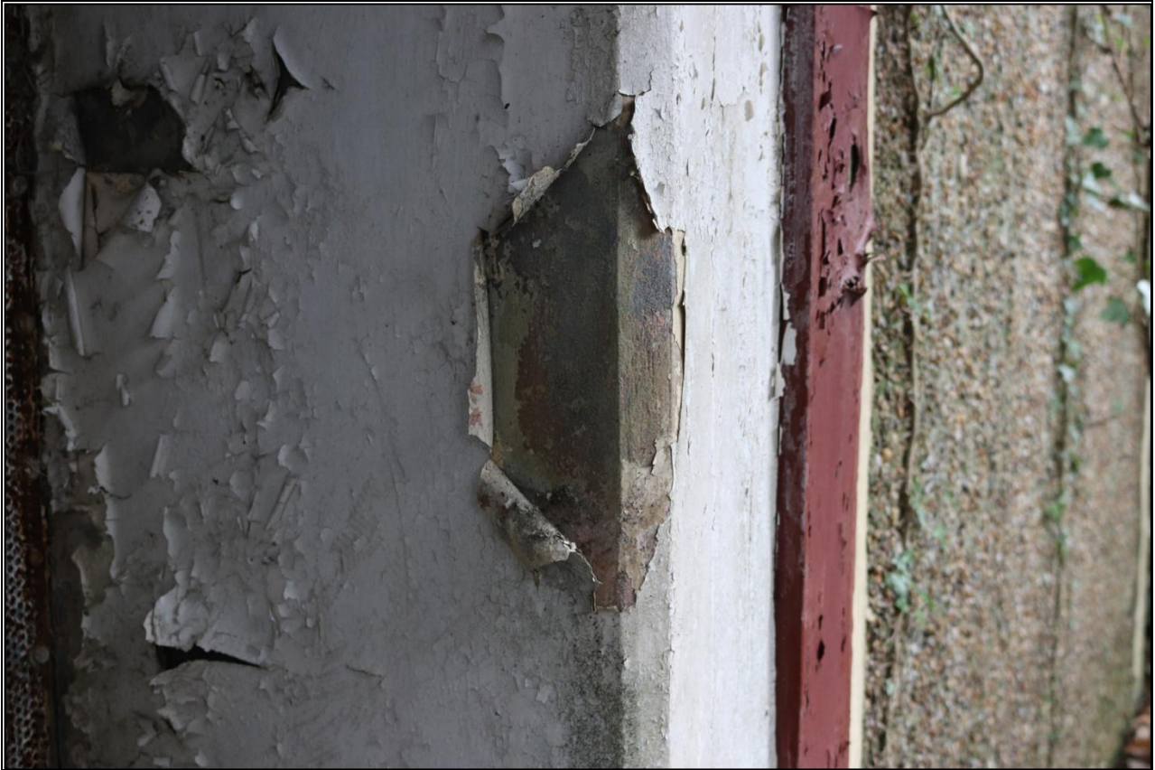
19. CHAMFERED STUCCO SURROUND WITH LOST PAINT LAYERS, MAY INFORM ON FORMER EXTERNAL FINISH.
