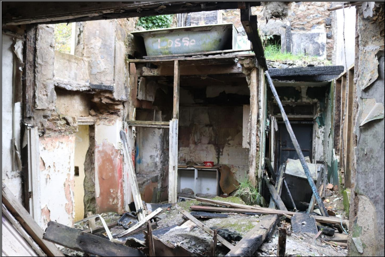
32. LOOKING BACK TO STAIR HALL AND FORMER KITCHEN, FROM THE NORTH.
