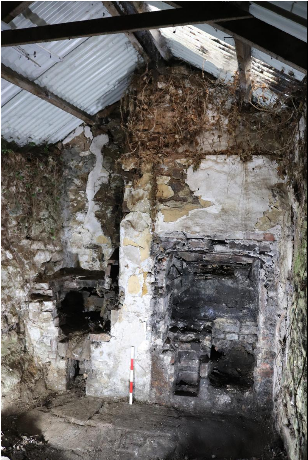
FIGURE 15: B1A LOOKING AT THE SOUTHERN GABLE, WITH ADDED SERVICE STACK AND LATER BRICK BUILT COPPER. GRANITE PAVERS ADDRESS STACK, FROM THE NORTH WITH 0.5M SCALE.
