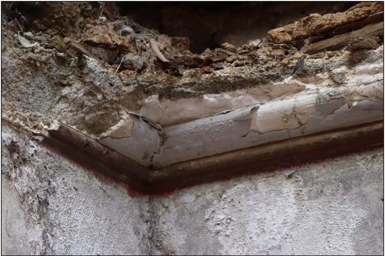
FIGURE 31: DETAIL OF CORNICE FOUND TO R3 INCLUDING EARLIER PAINT SCHEMES OVER A REFINED LIME PLASTER.
