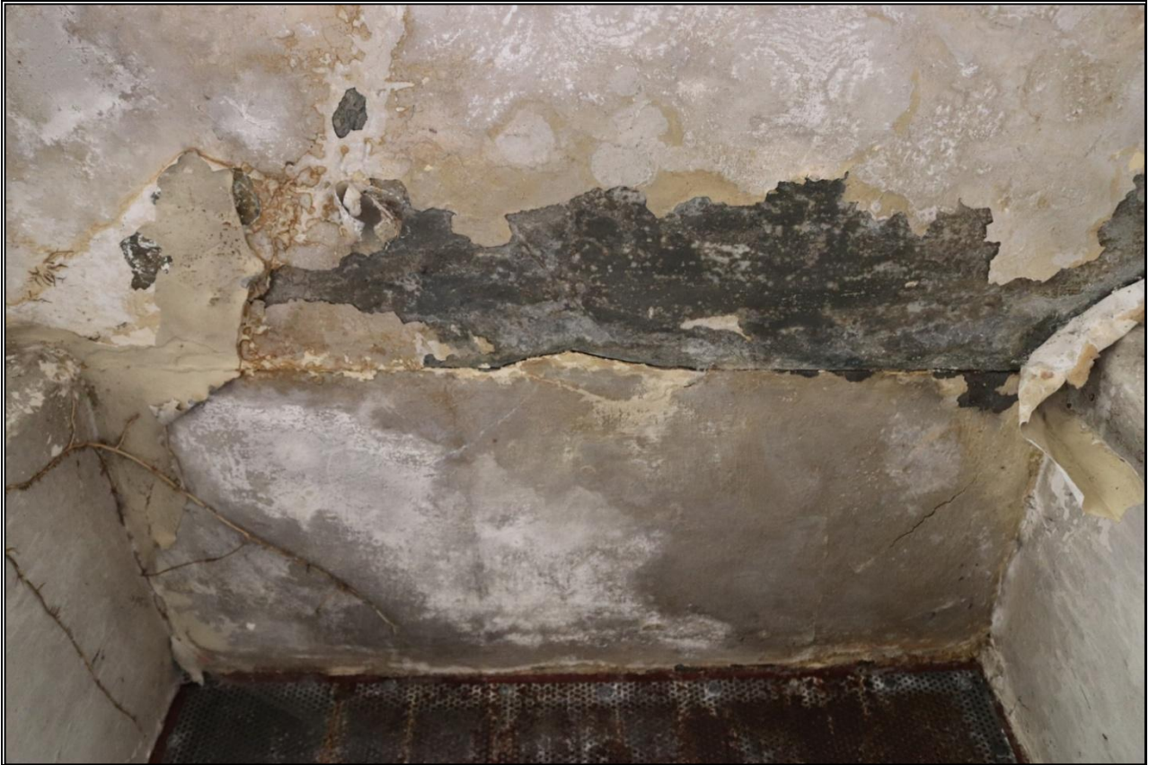
17. HEAVY SLATE SLAB CANOPY.
