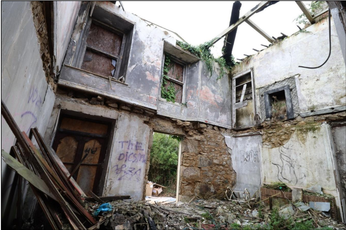
FIGURE 9: R3 RECEPTION ROOM AND FF ROOM ABOVE, FROM THE SOUTH-EAST WITH WIDE-ANGLED LENS.
