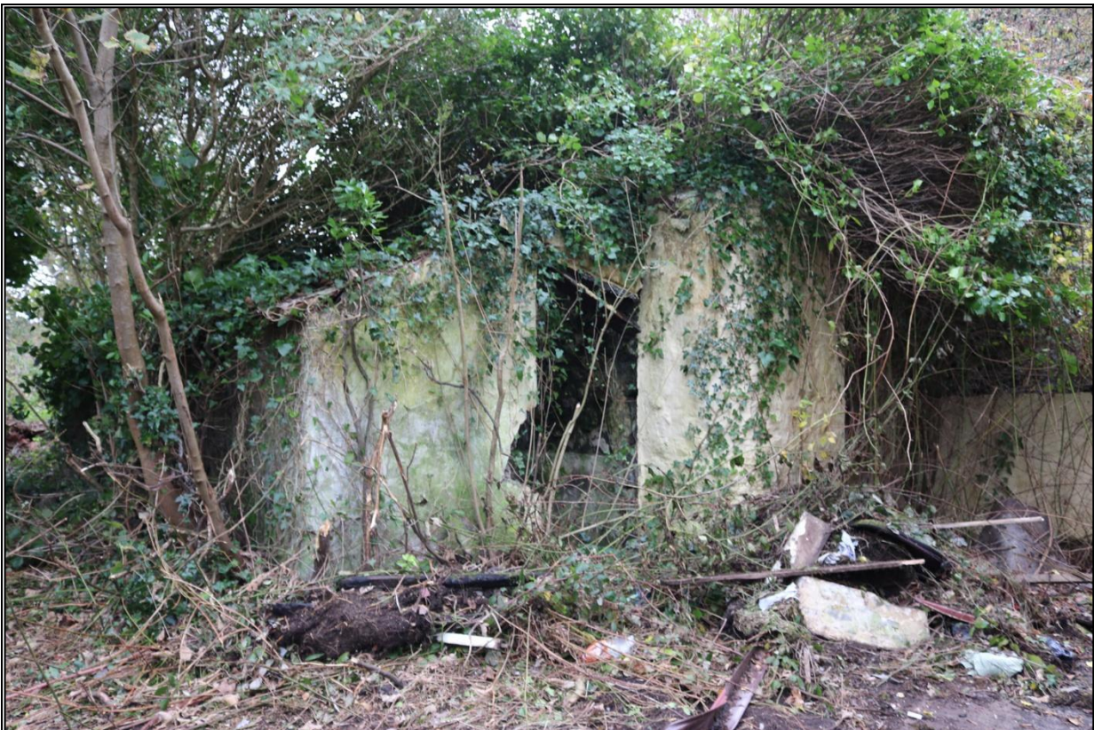
4. INACCESSIBLE OUTBUILDING TO THE NE OF THE HOUSE.
