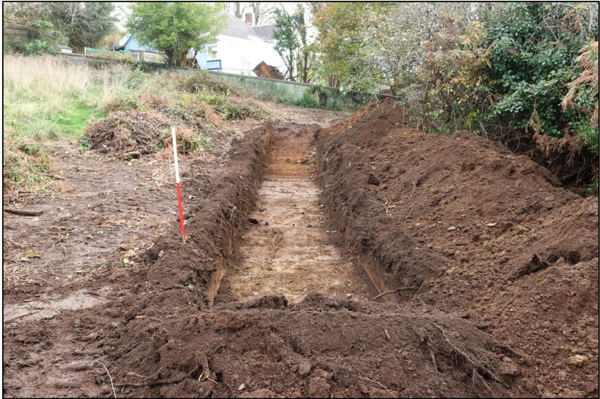
FIGURE 50: TRENCH 7 FROM NW (1M SCALE)
