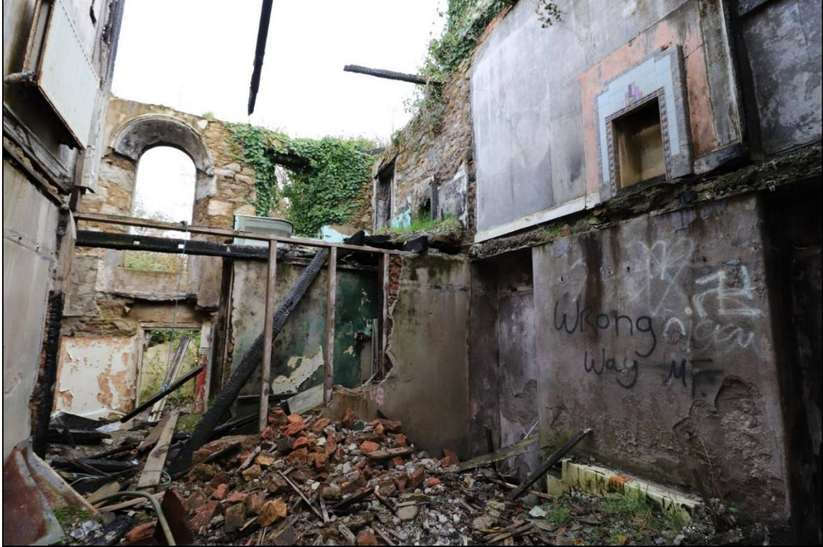
FIGURE 8: R2 RECEPTION ROOM, FROM THE EAST, WITH WIDE-ANGLED LENS.
