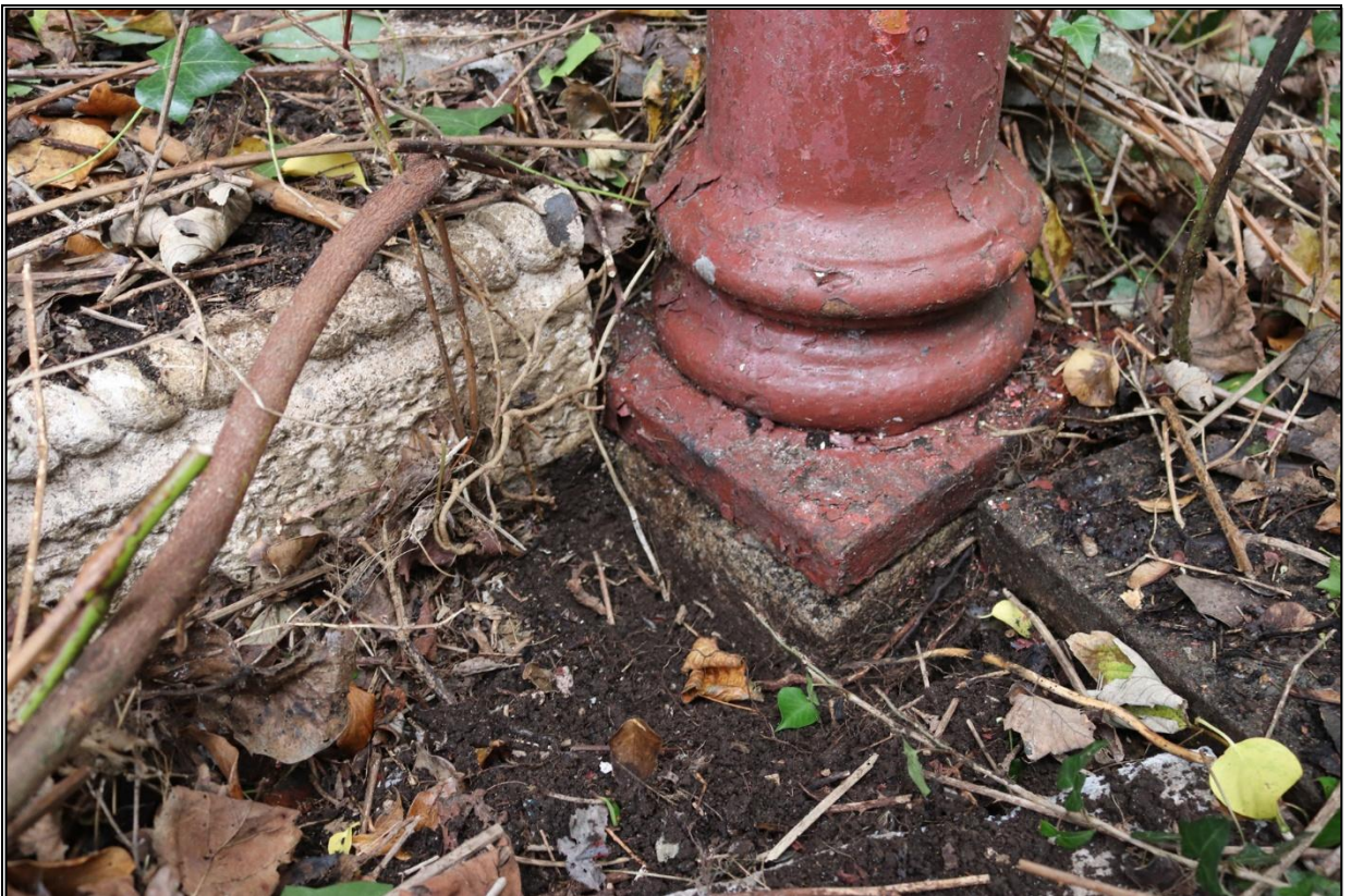
16. BASE OF THE COLUMNS SET ON TO GRANITE PADS.
