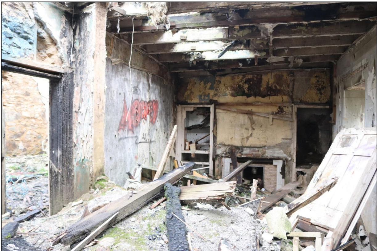
FIGURE 10: R4 FROM THE SOUTH, SHOWING CURVED PARTITION FOR R3 DOOR, TAKEN WITH WIDE-ANGLED LENS.
