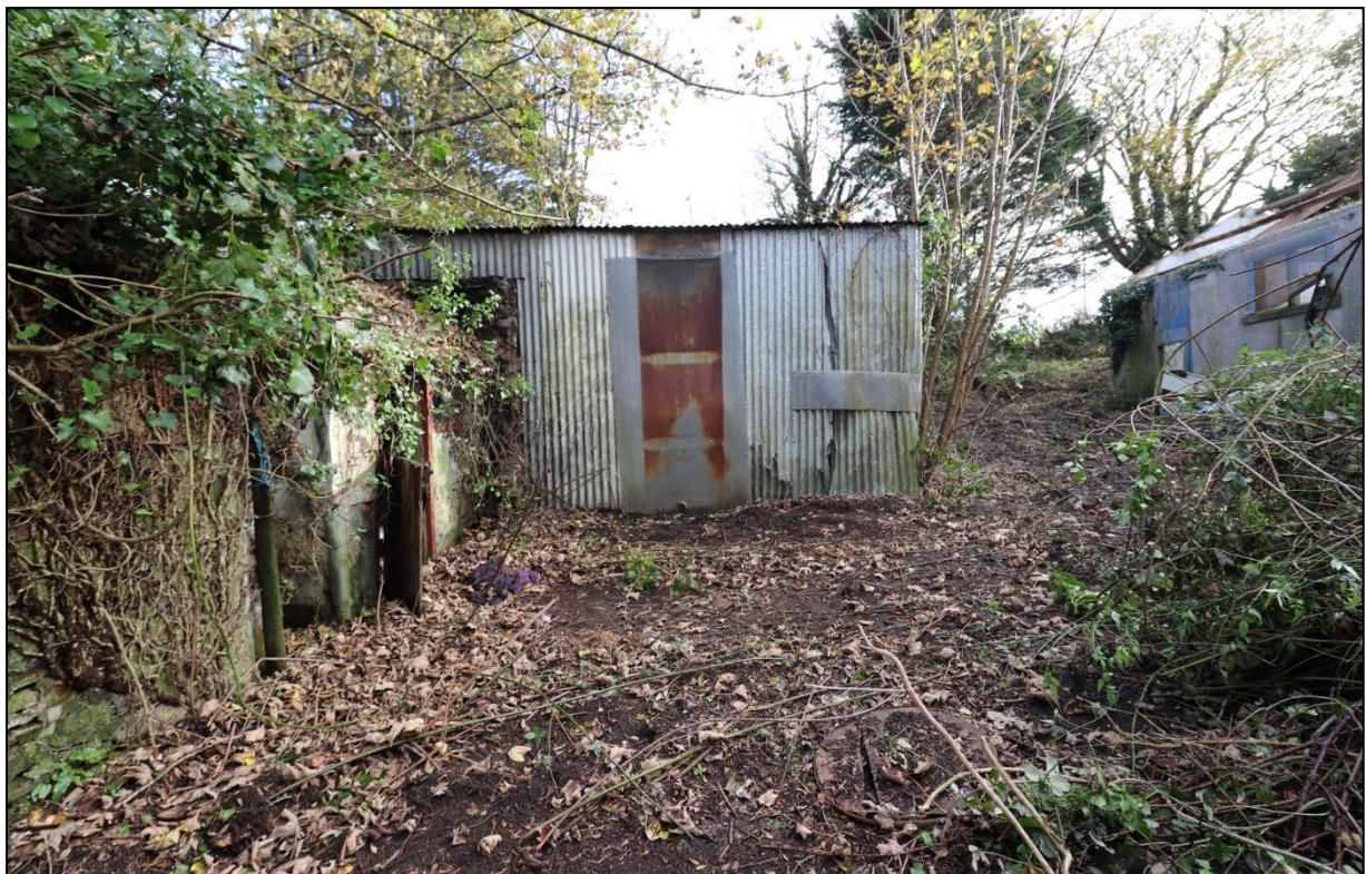
FIGURE 14: LOOKING TO B2 GARAGE, BEYOND TO SOUTH IS B3 CONCRETE BLOCK FORMER DAIRY, FROM THE NORTH – TAKEN WITH WIDE-ANGLED LENS.
