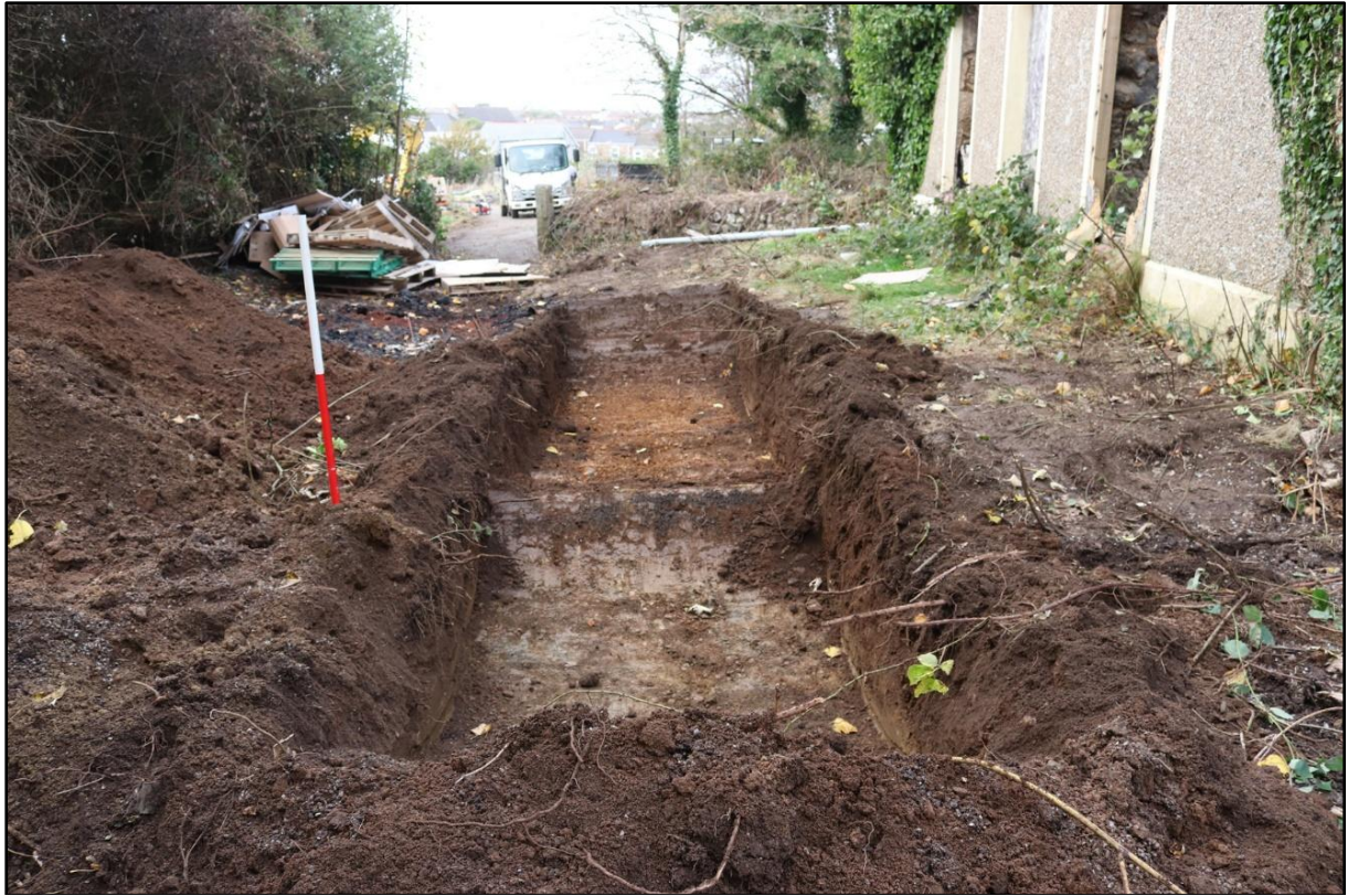
FIGURE 55: TRENCH 9 WITH GAS PIPE FROM SSE.
