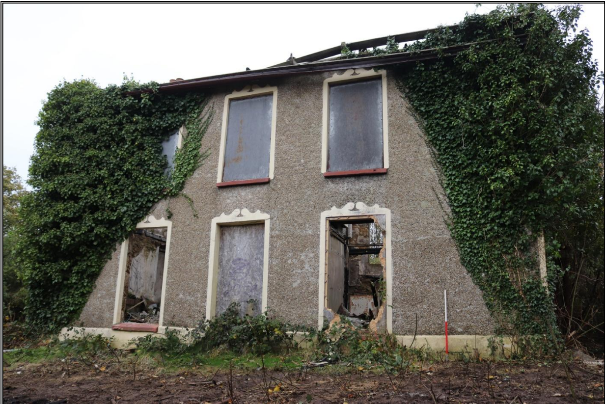
13. THE WEST FACING ELEVATION, FROM THE SW WITH 1M SCALE.
