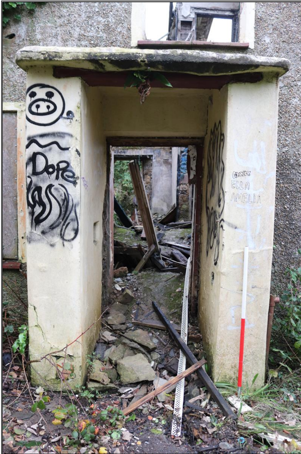
11. THE REAR PORCH, LOOKING THROUGH FORMER ACCESS, FROM EAST WITH 1M SCALE.
