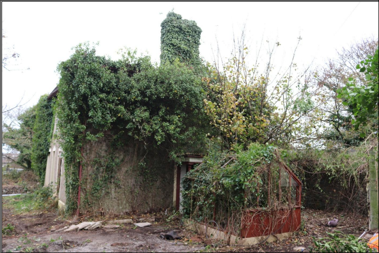
7. THE SOUTH GABLE END, LARGELY OVERGROWN, MAIN PORCH OBSCURED BY MODERN TIMBER-FRAMED GREENHOUSE, FROM THE SSW.
