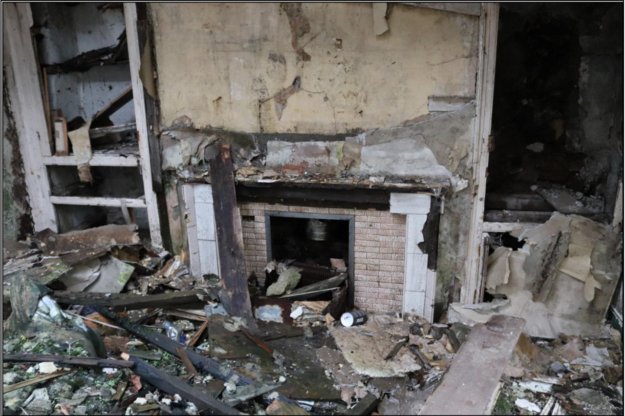
28. ALTERED FIREPLACE AND FLANKING CUPBOARDS R4 AGAINST NORTH WALL, FROM THE SE.
