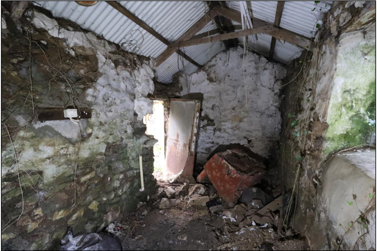
FIGURE 20: THE NORTHERN END OF B1A, FROM THE SOUTH TAKEN WITH WIDE-ANGLED LENS.
