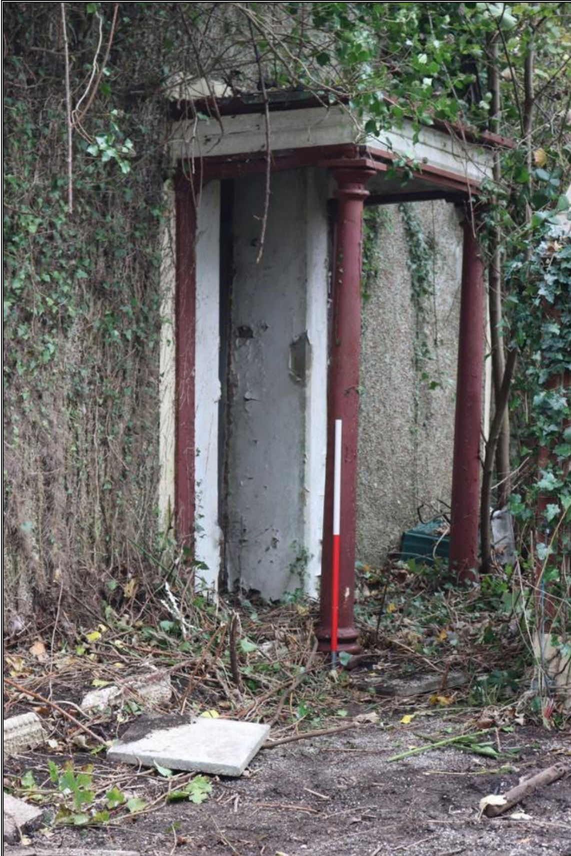
14. THE FORMER FORMAL ACCESS WITH REUSED PORCH TO THE SOUTH GABLE, FROM THE SW WITH 1M SCALE.
