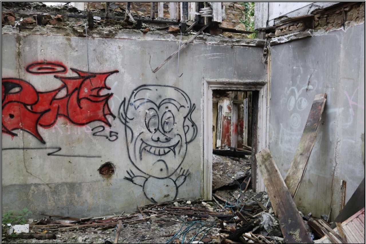
38. LOOKING TO THE SE CORNER OF R3, FROM THE NNW.
