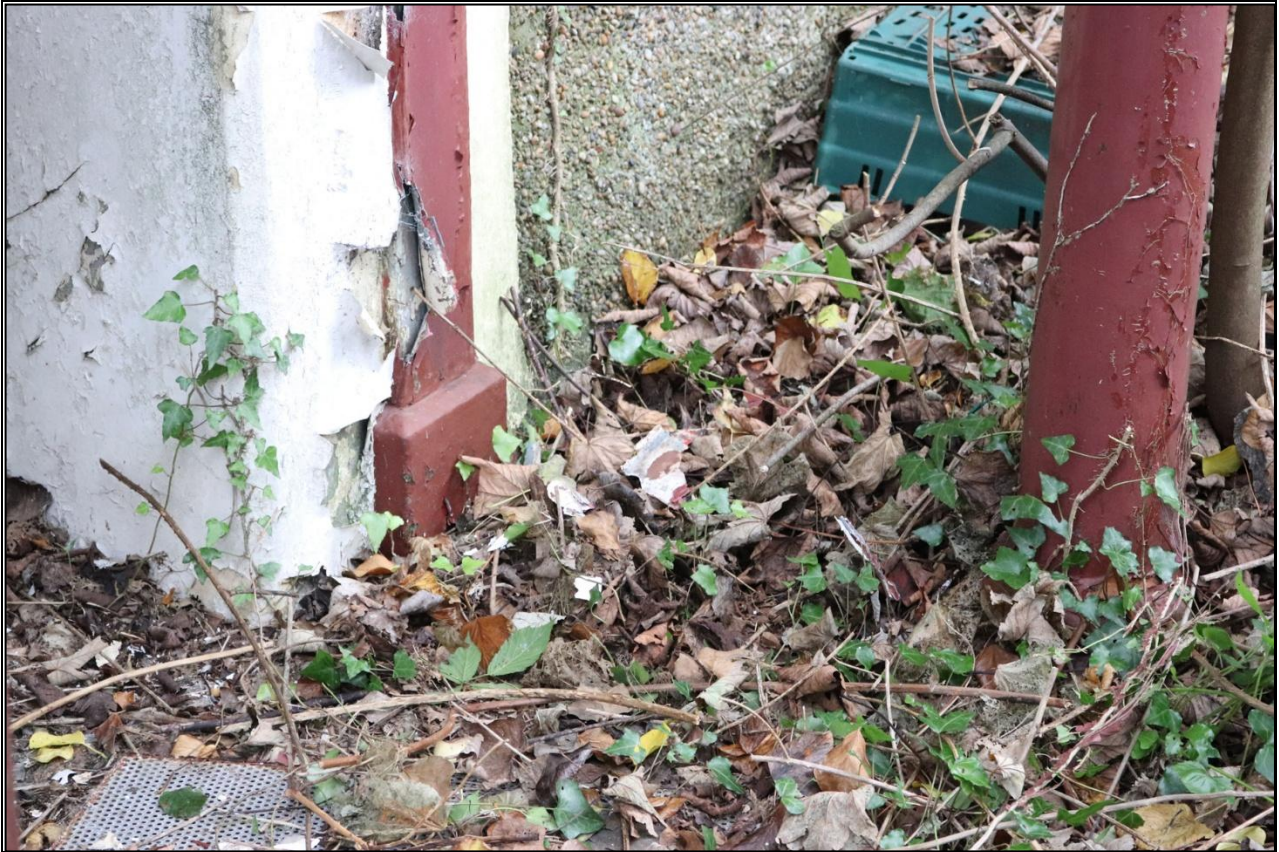
22. BASE OF OPENING AGAINST COLUMN.
