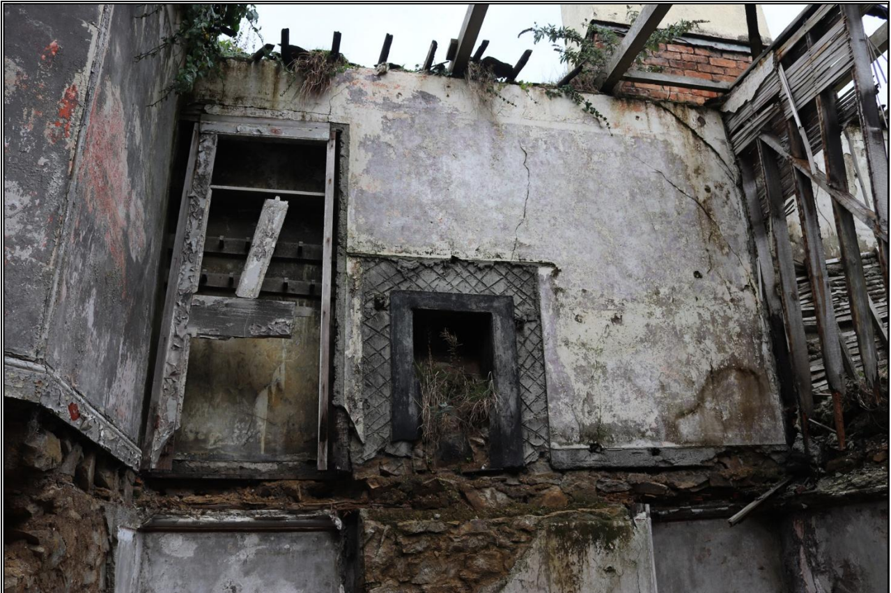
43. FF FIREPLACE OVER R3, FROM SOUTH.
