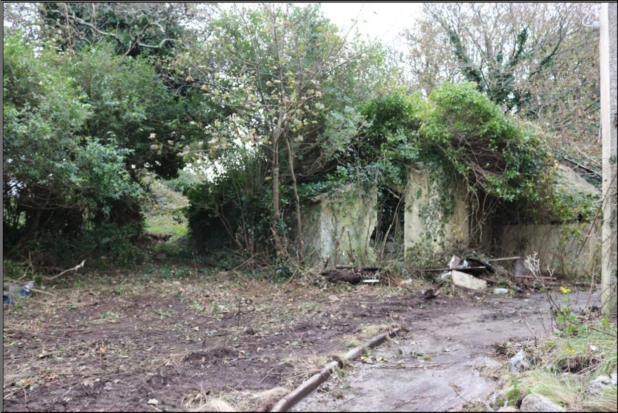
3. HOUSE LEADING AROUND FROM THE WEST, FOLLOWING A PATH THAT WRAPS NORTH ELEVATION TO DILAPIDATED OUTBUILDINGS. FROM THE WNW.
