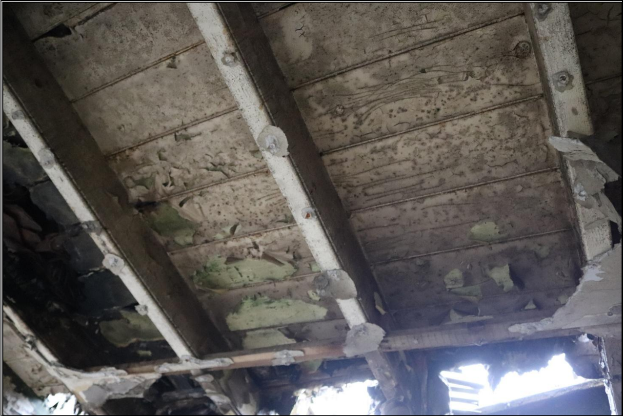
30. CEILING TO R4 LARGELY LOST THOUGH SHOWS BEADED JOISTS AND FLOORBOARDS.
