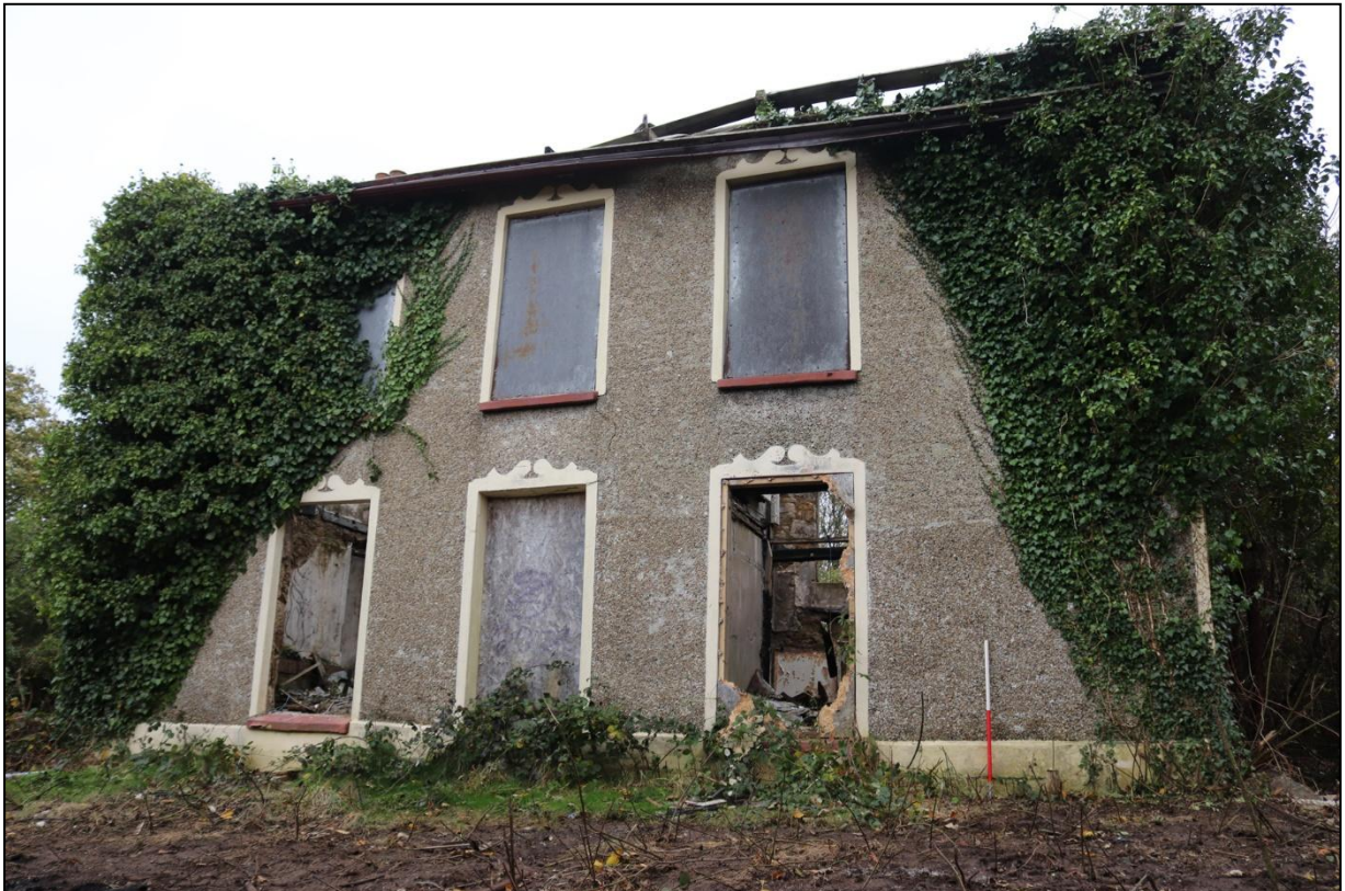
FIGURE 5: THE EAST-FACING ELEVATION, FROM THE ESE WITH 1M SCALE.
