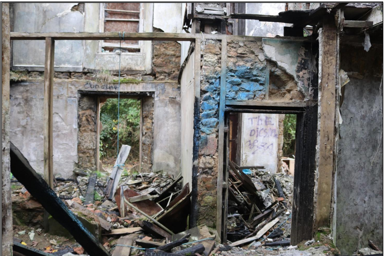
25. ENTERING THE HOUSE THROUGH REAR PORCH, FROM THE EAST.
