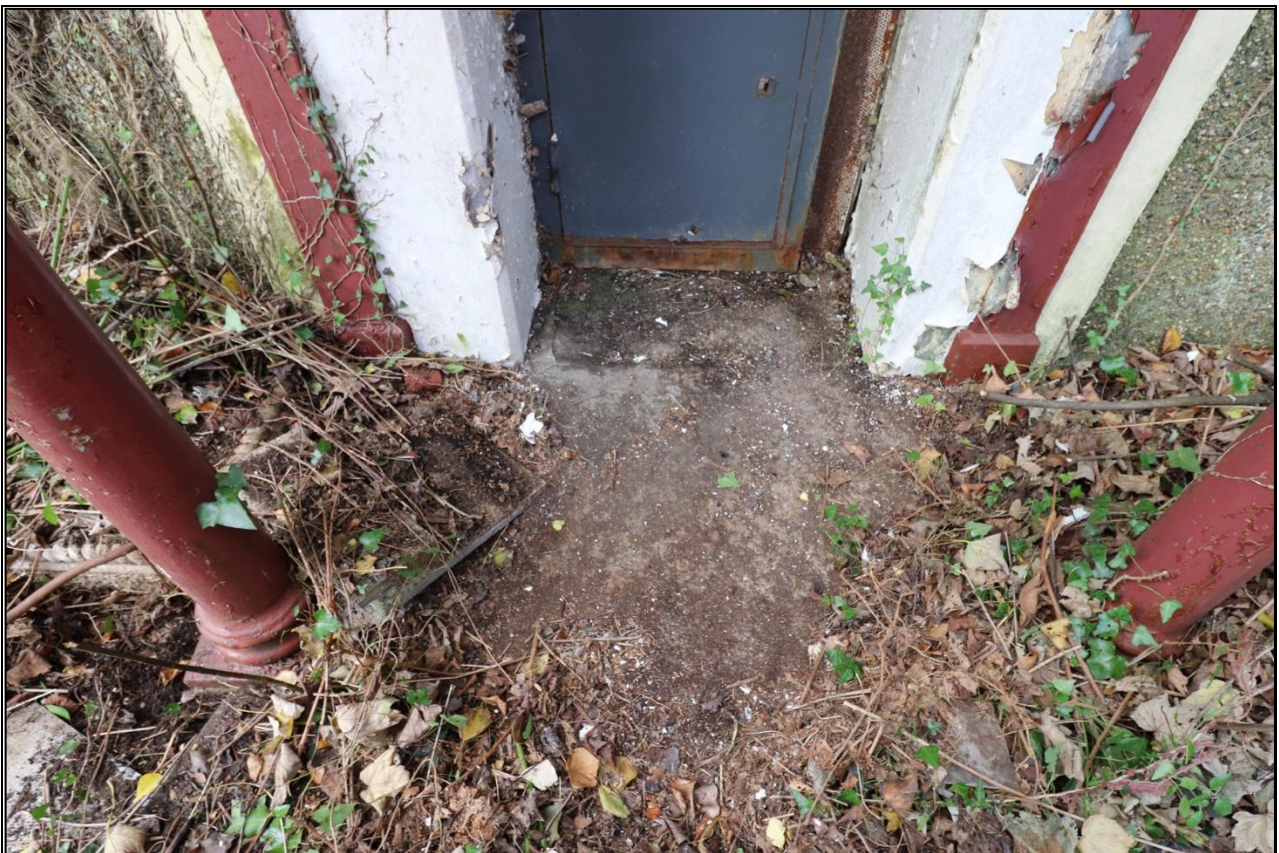
23. GRANITE THRESHOLD OF PORCH, TAKEN WITH WIDE-ANGLED LENS.
