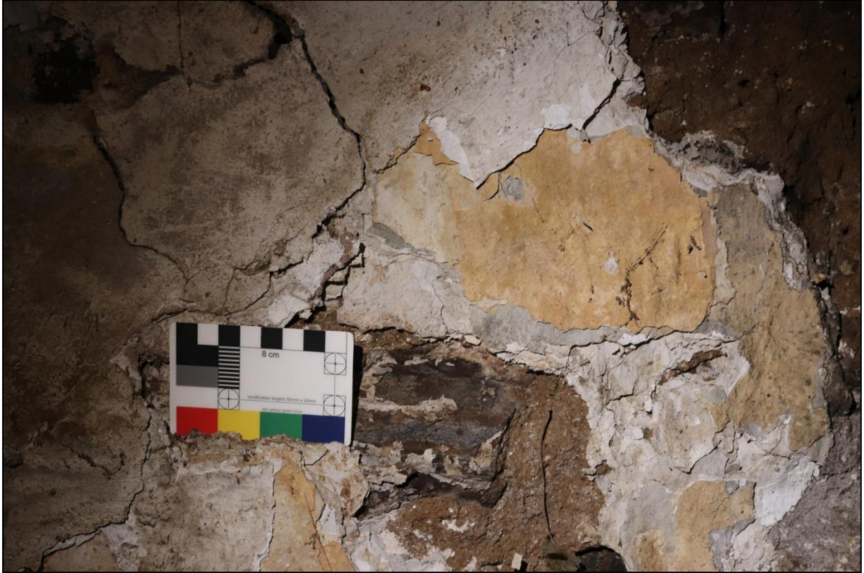
FIGURE 18: COLOUR WASHES EVIDENT AGAINST STACK AND COPPER REFLECTING DECORATIVE SCHEMES TO SECONDARY SPACES, WITH A COLOUR-CARD AND 5CM SCALE.
