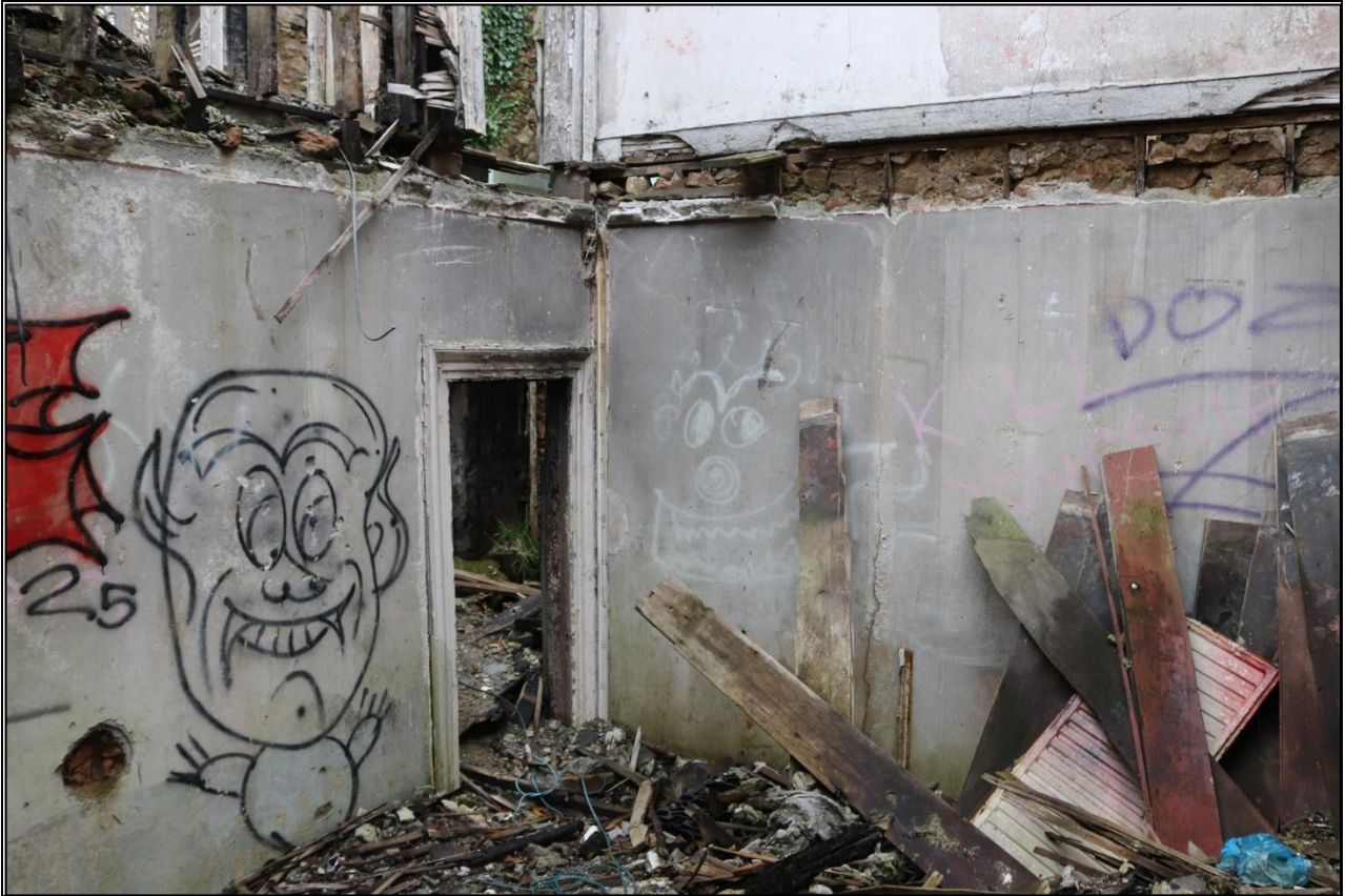
40. SW CORNER OF R3, FROM THE NW.
