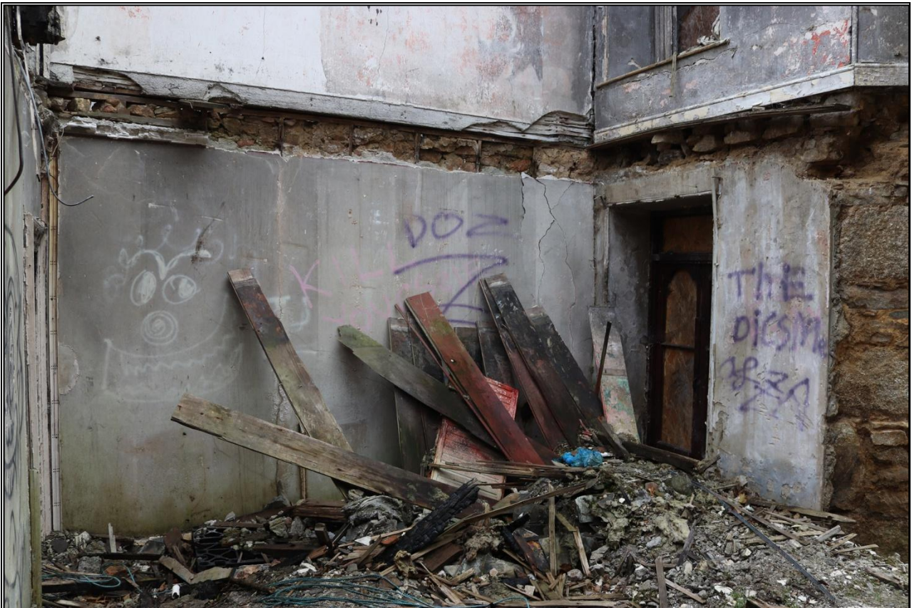
41. SOUTH WALL OF R3, FROM THE NNE.
