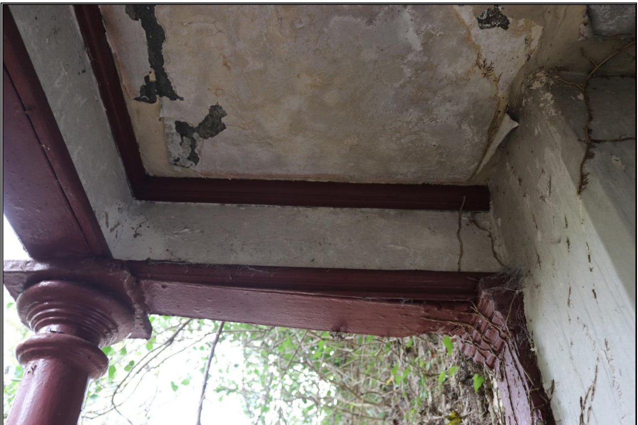
18. DETAIL BETWEEN COLUMN AND ENGAGED PILASTER.
