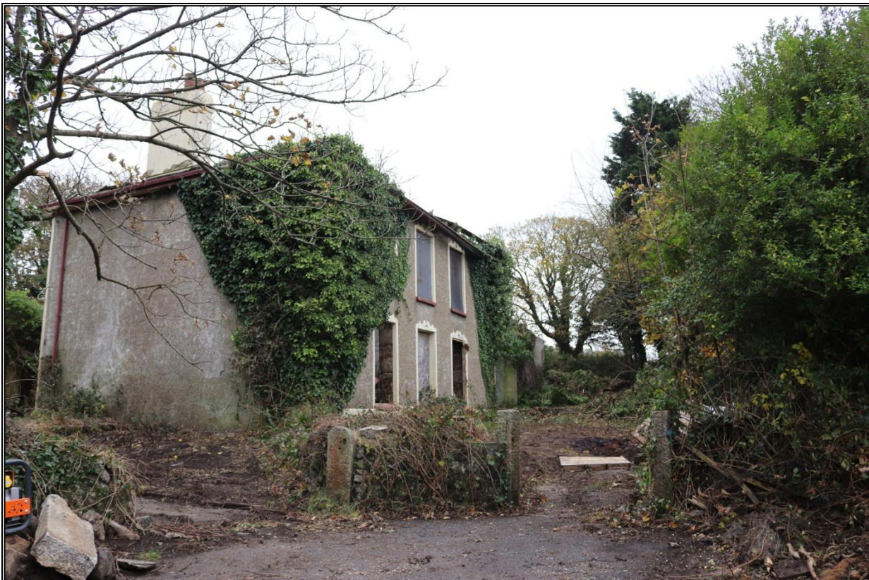
2. NORTH GABLE AND WEST ELEVATION. FROM THE NORTH-WEST.
