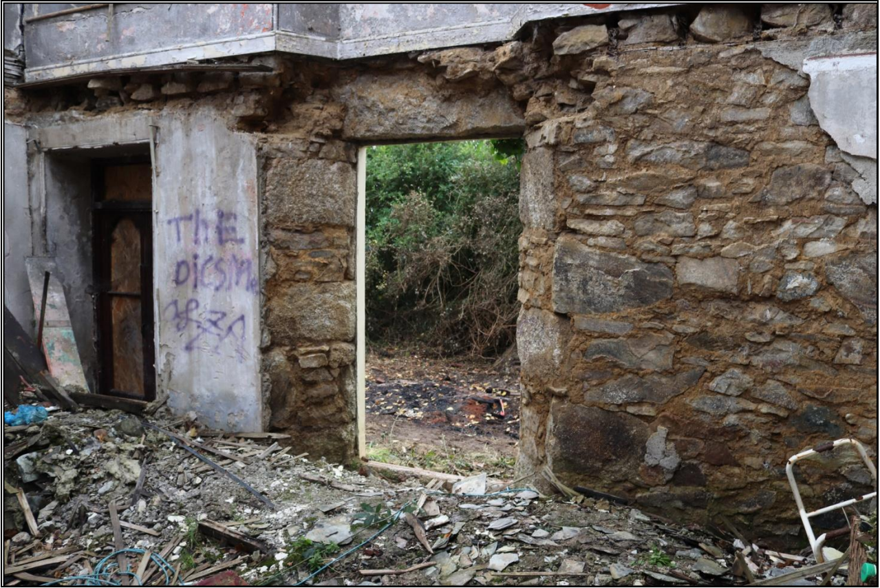
42. R3 WEST - WINDOW WITH DEEP REVEALS FLANKING ALTERED DOOR OPENING, FROM THE NE.
