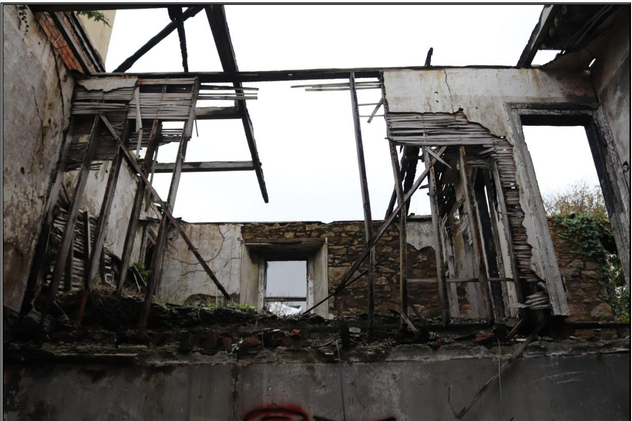
39. LOOKING TO FF ROOM ABOVE R4 SHOWING LATH AND PLASTER FF PARTITIONS OVER RUBBLE GF PARTITIONS.
