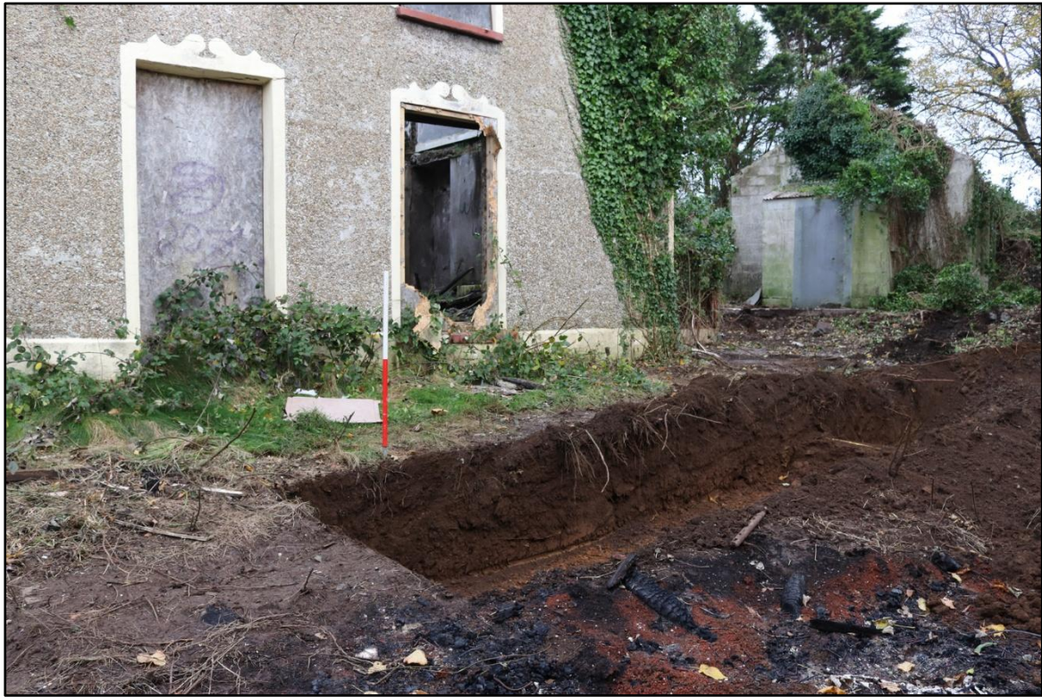
FIGURE 57: TRENCH 9 WITH GAS PIPE FROM NORTH-WEST (1M SCALE).
