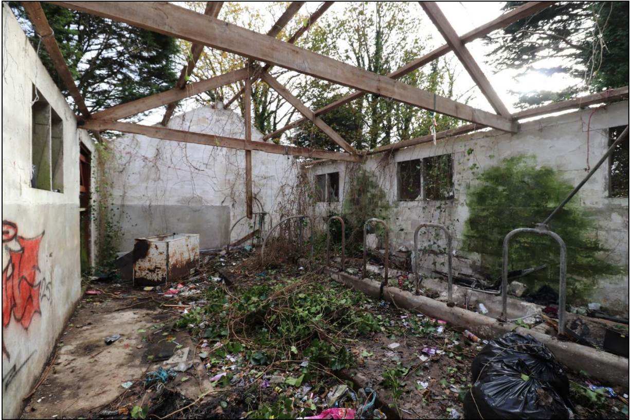
FIGURE 24: B3 CONCRETE BLOCK, MUCH LATER DAIRY WITH FEED PASSAGE ALONG THE WEST, FROM THE NE WITH WIDE-ANGLED LENS.
