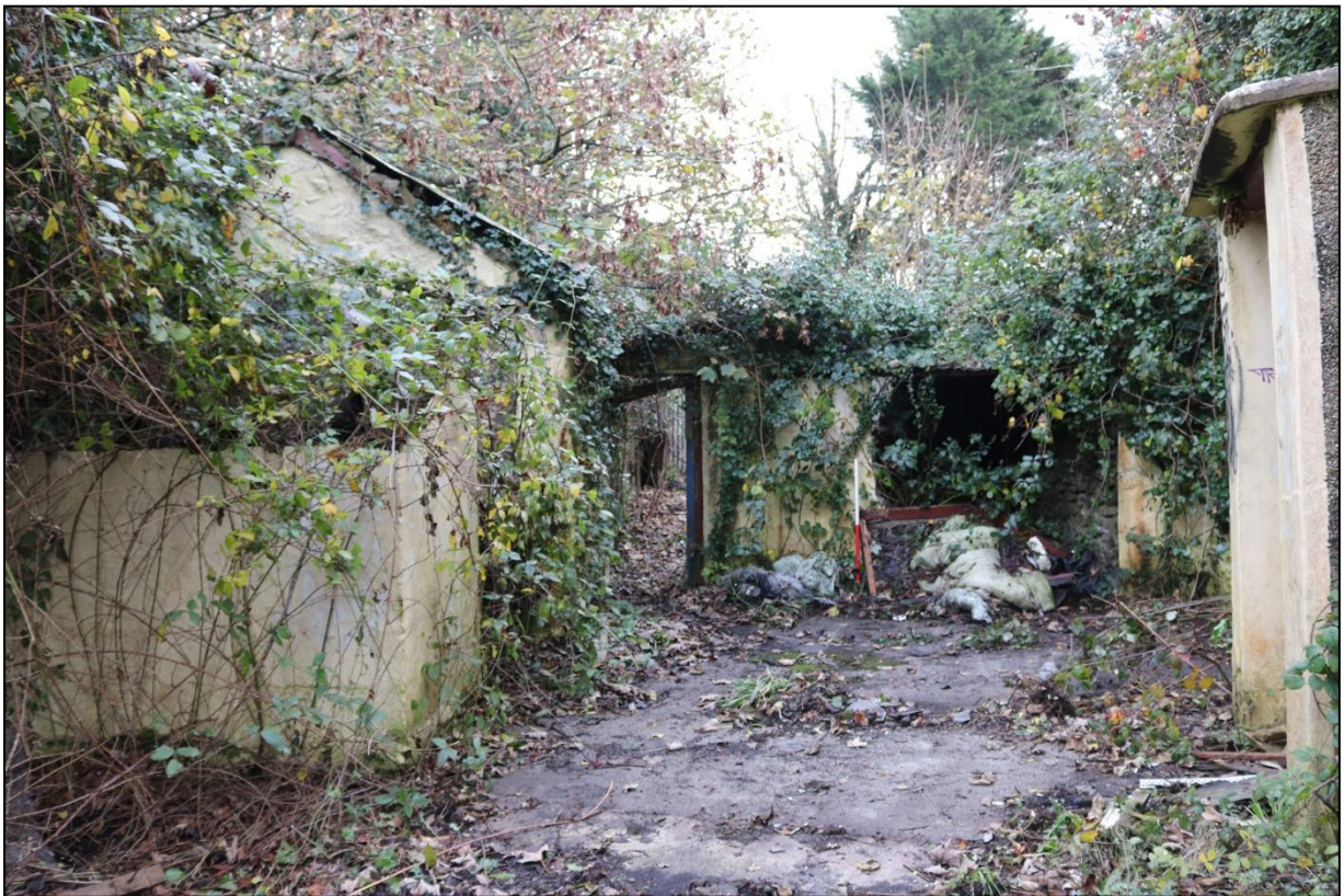
FIGURE 12: B2 LOOKING TO B1 AND HOUSE PORCH, FROM THE NORTH.
