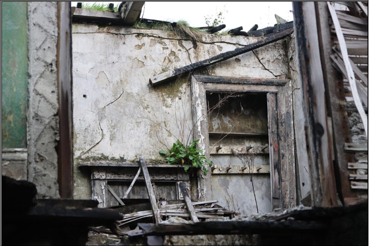
36. LOOKING THROUGH TO FF ROOM OVER R4 WITH ORIGINAL FIREPLACE IN SITU.
