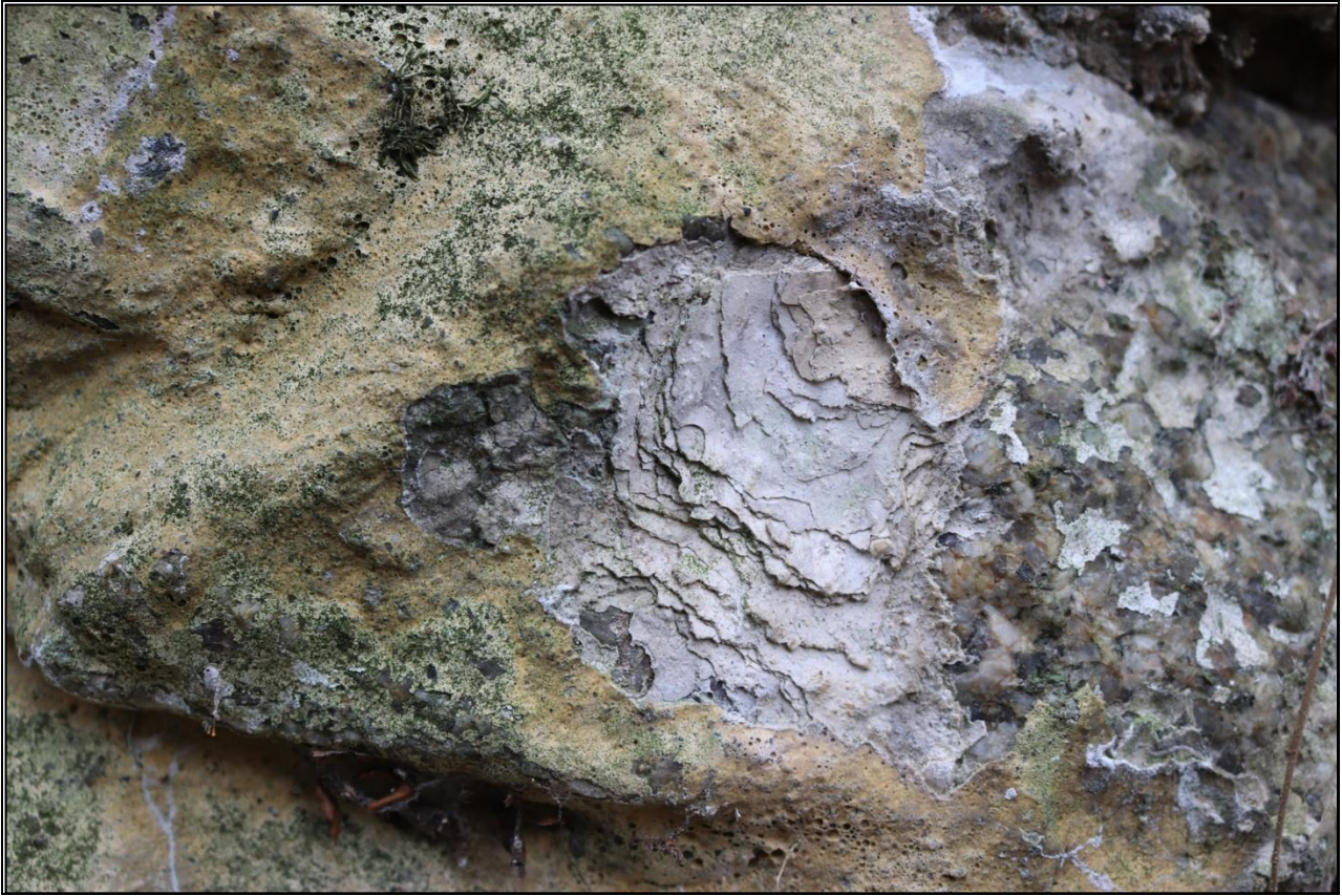
24. LIMEWASHED LAYERS SEEN TO GARDEN WALLS.
