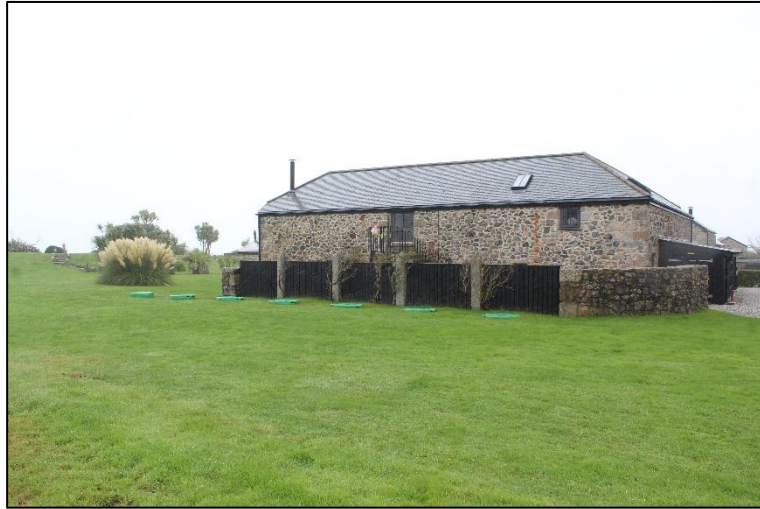
21. FIELD F3, VIEW OF GONWIN MANOR; VIEWED FROM THE SOUTH-WEST (NO SCALE).
