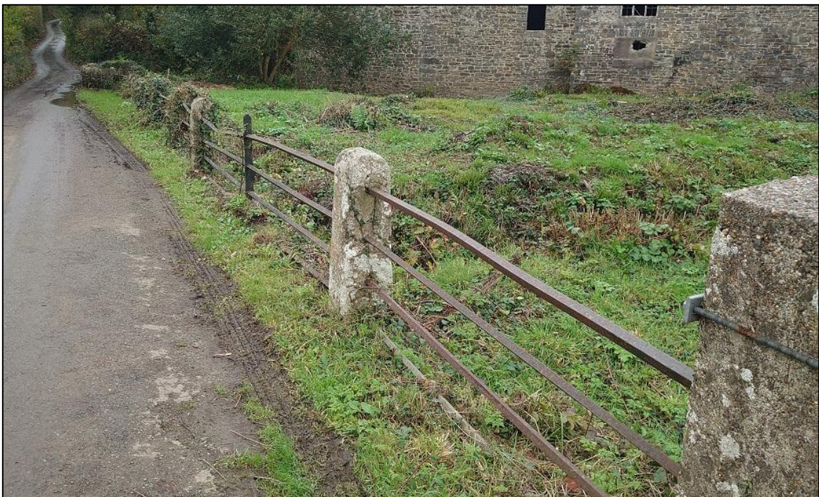
FIGURE 15: THE SMART 19 TH CENTURY FENCING TO THE ROAD, WITH GRANITE POSTS AND IRON RAILS; FROM THE WEST, SOUTH-WEST.
