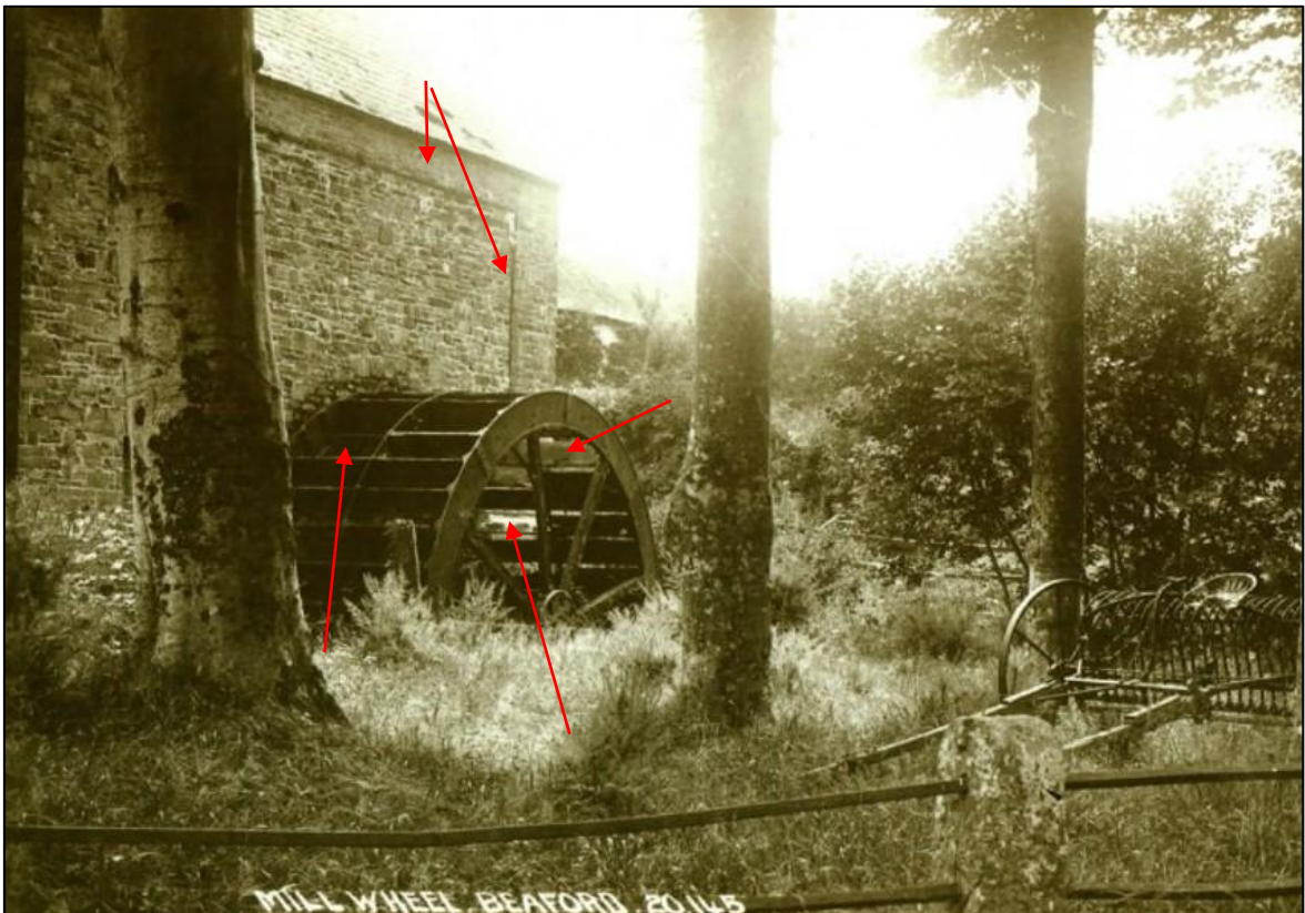
FIGURE 4: ANOTHER EARLY-MID 20 TH CENTURY PHOTOGRAPH OF THE MILL WHEEL IN SITU, THE SITE AGAIN LOOKS OVERGROWN. THE PHOTOGRAPH IS SHOWING A TYPICAL UNDERSHOT FED WHEEL USING TIMBER FLOATS AND IRON RINGS AND BARS OF DOUBLE-WIDTH FORM, SOME OF THE FLOATS CAN BE SEEN TO BE MISSING ON THE WHEEL AND THE HOUSING CHAMBER OVER THE WHEEL HAS ALREADY BEEN REMOVED, THE FLASHINGS CAN CLEARLY BE SEEN. (PROVIDED BY CLIENT).
