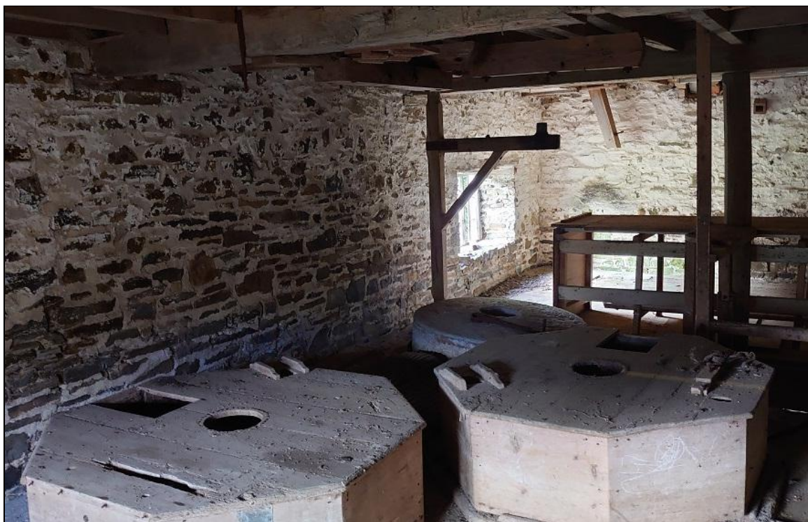
FIGURE 13: FIRST FLOOR OF THE REAR BLOCK OF THE MILL, WITH ENCASED MILLSTONES IN SITU; FROM THE EAST-NORTH-EAST.
