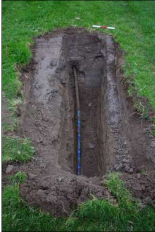
FIGURE 6. PIT 1 DUG TO FULL DEPTH WITH THE DRAINAGE PIPE INSTALLED.
