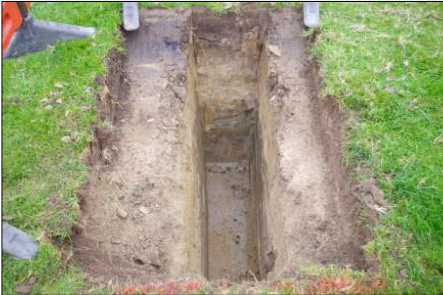
FIGURE 4. PIT 2. DUG TO FULL DEPTH (1.00M).
