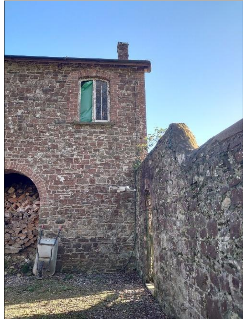
FIGURE 17: THE COURTYARD WALL AND SOUTH END OF THE BUILDING.
