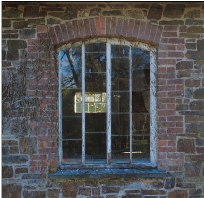
FIGURE 19: ONE OF THE WINDOWS IN THE WEST ELEVATION OF THE SAWMILLS BUILDING, A STYLE COMMON IN THE 19 TH CENTURY, ALTHOUGH THESE WINDOWS APPEAR TO BE 20 TH CENTURY COPIES.
