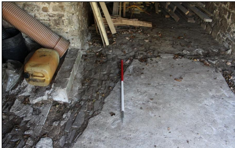
FIGURE 13: THE COBBLED FLOOR ON THE LOWER GROUND FLOOR, COVERED BY CEMENT/CONCRETE; (FROM THE WEST 1M SCALE).
