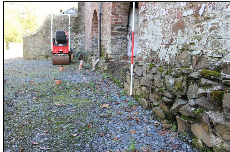
FIGURE 15: THE EXPOSED ROUGH FOUNDATIONS OF THE BUILDING (1M SCALE); FROM THE SOUTH-WEST.
