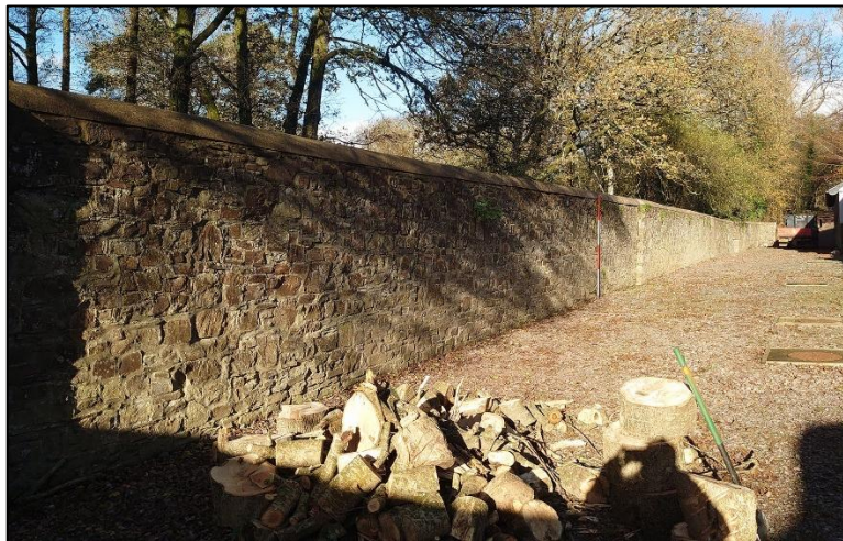
FIGURE 16: THE COURTYARD WALL WHICH ENCLOSES THE BUILDING (2M SCALE).
