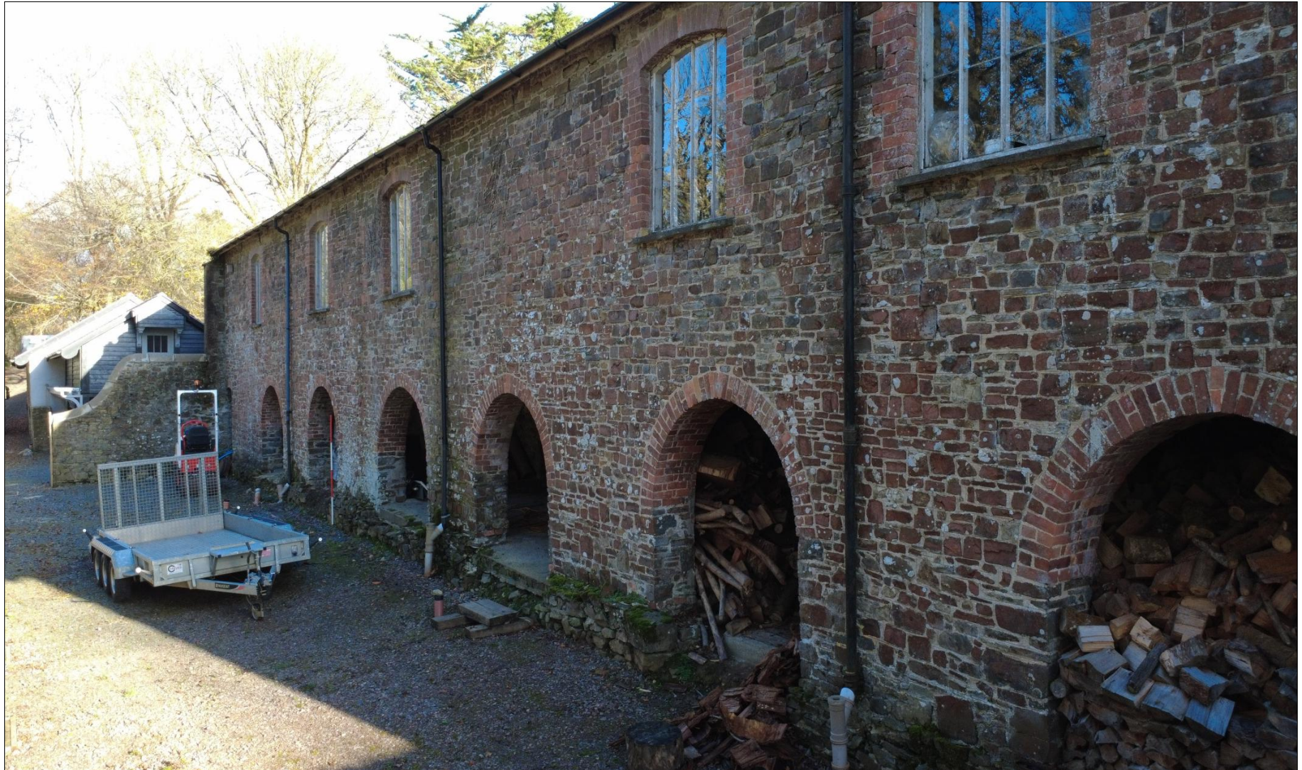
Figure 6: WIDE VIEW OF WEST ELEVATION (2M SCALE).
