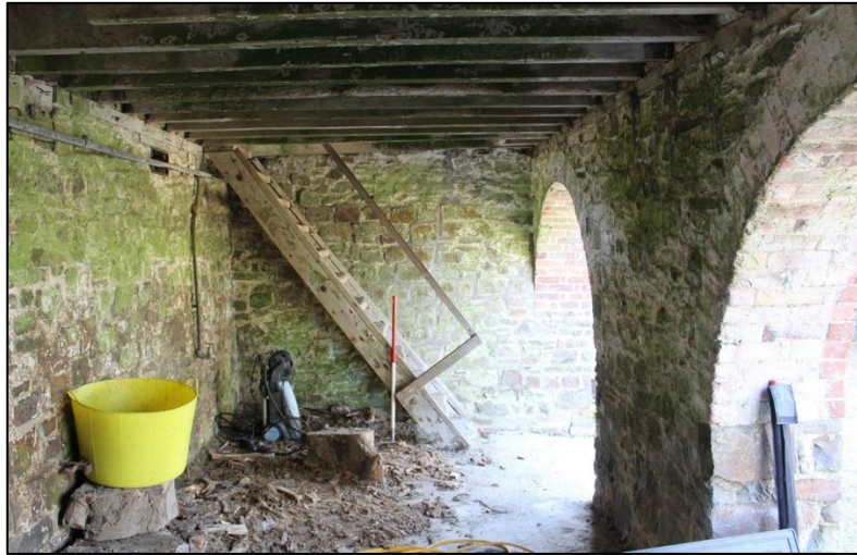
FIGURE 12: THE LADDER FROM THE LOWER TO UPPER GROUND FLOOR FORM THE NORTH (1M SCALE).
