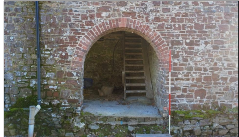
FIGURE 18: DETAILED PHOTOGRAPH OF ONE OF THE ROUND-HEADED ARCHES WHICH DEFINES THE WEST ELEVATION (2M SCALE); FROM THE WEST.
