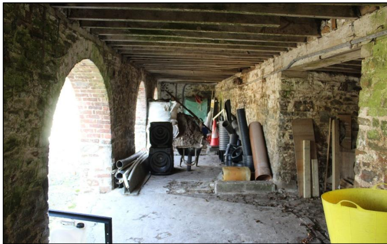
FIGURE 10: THE LOWER GROUND FLOOR, NOW USED FOR STORAGE; FORM THE SOUTH.
