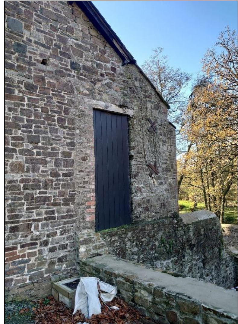
FIGURE 20: THE NORTH-WEST CORNER, THE REMAINS OF AN ADJACENT BUILDING INCORPORATED INTO THIS BUILDING.
