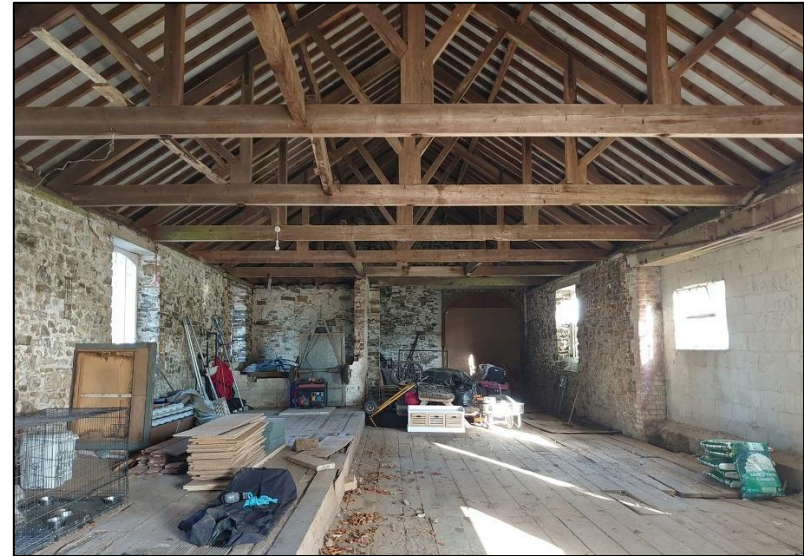
FIGURE 7: INTERIOR VIEW OF UPPER GROUND FLOOR.
