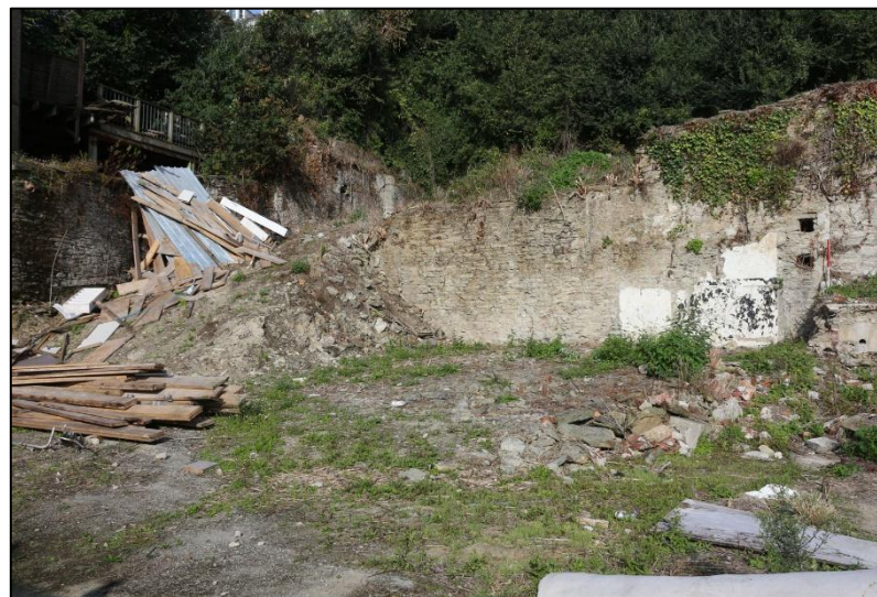
FIGURE 15: THE NW PART OF THE CAR PARK SITE IN 2024; FROM THE SE.
