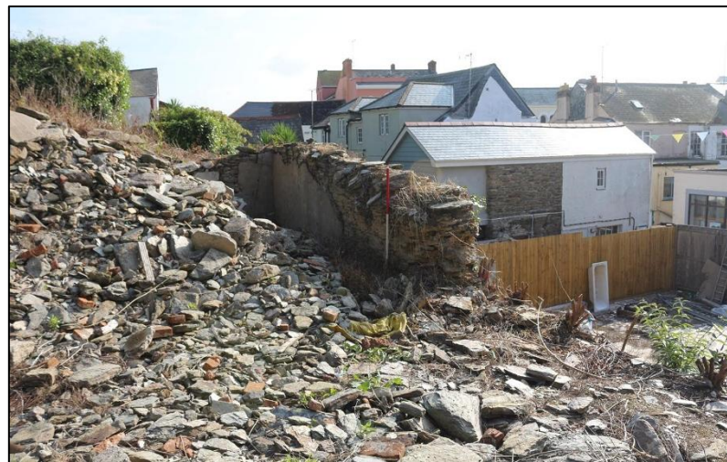
FIGURE 18: THE SURVIVING SOUTH-EAST CORNER OF THE CHAPEL IN 2024; FROM THE NW (SCALE 1).
