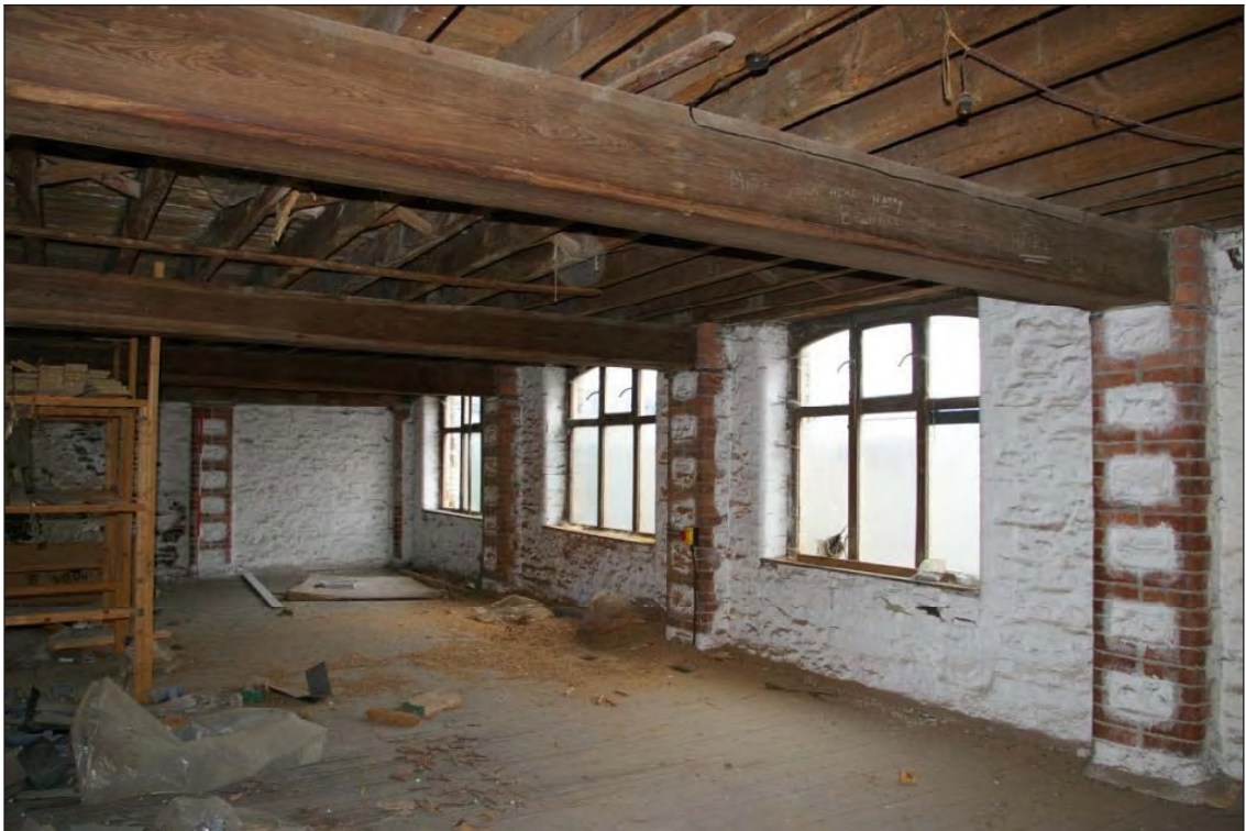
Figure 19: Room 11 viewed from the south-west (2m scale).
