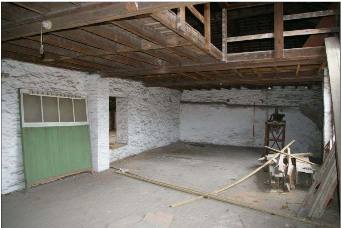
Figure 17: Room 9 viewed from the south-west (2m scale).
