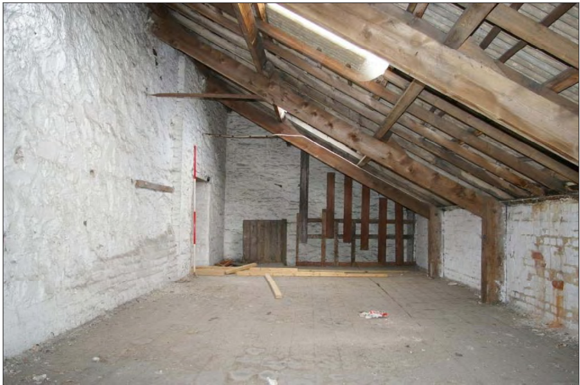
Figure 18: Room 10 viewed from the east (2m scale).
