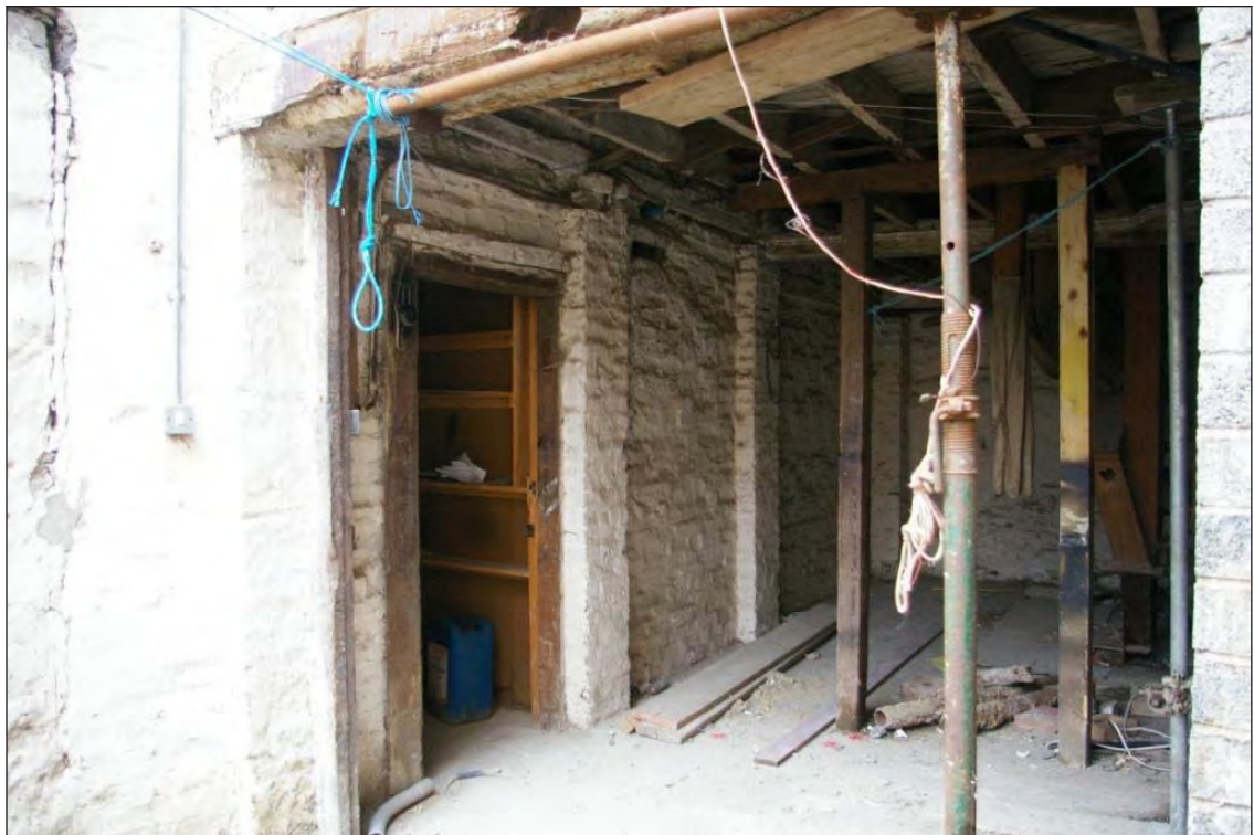
Figure 13: Room 5a and the entrance to Room 5b, viewed from the west.
