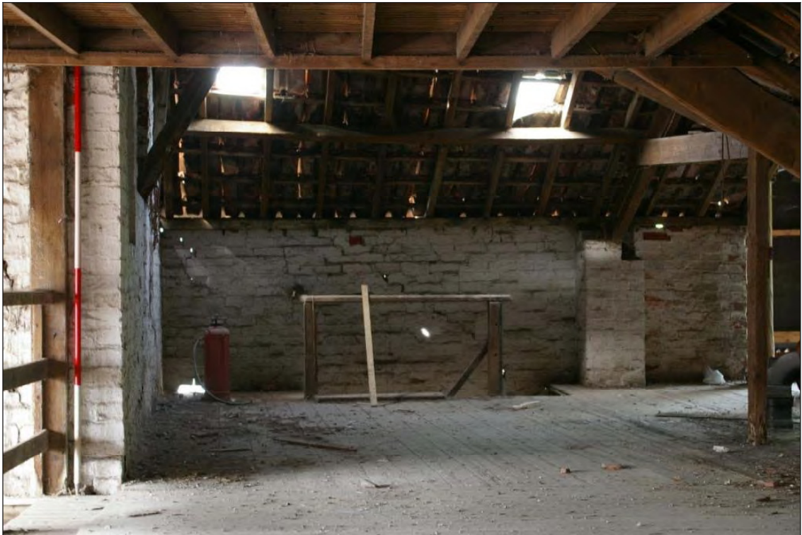
Figure 23: Room 15, viewed from the east (2m scale).
