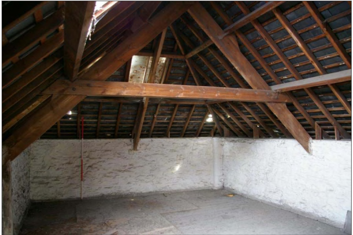
Figure 24: Room 16 viewed from the south (2m scale).
