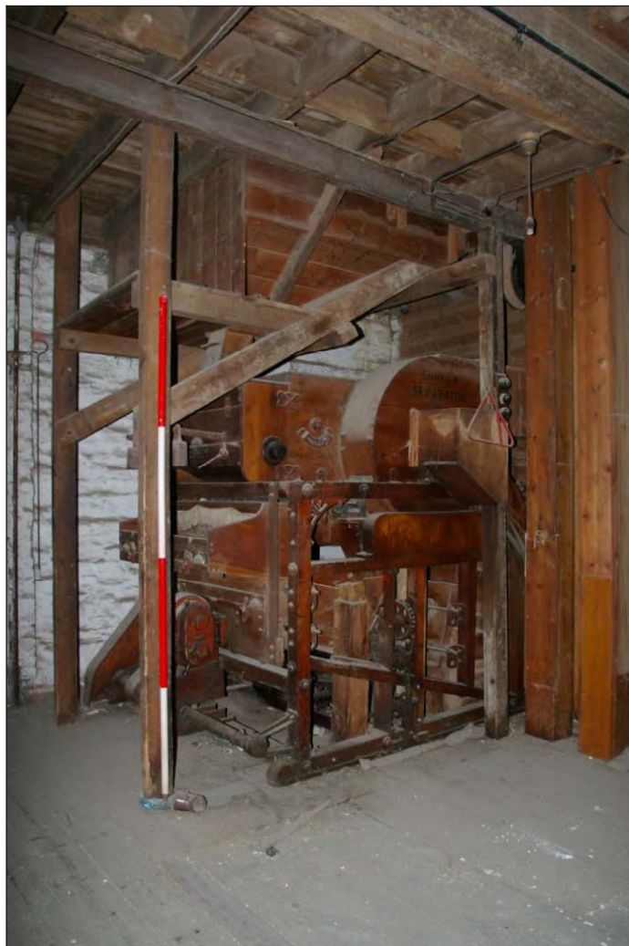
Figure 20: The Eureka Separator No.3 in wooden frame in the north east corner of Room 12, viewed from the south west (2m scale).
