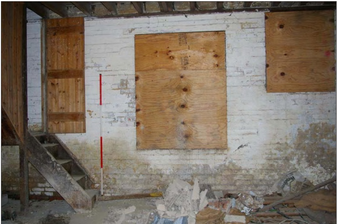
Figure 12: The northern elevation of Room 4, viewed from the south (2m scale).
