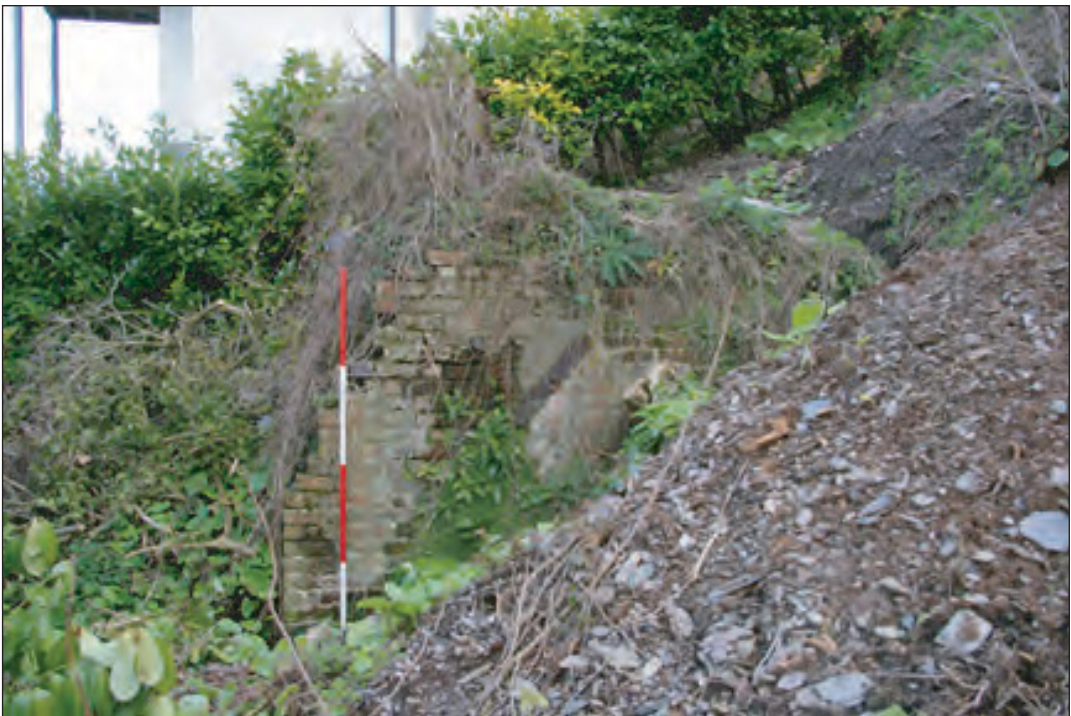
Plate 2: The water tank prior to work commencing, viewed from the west.
