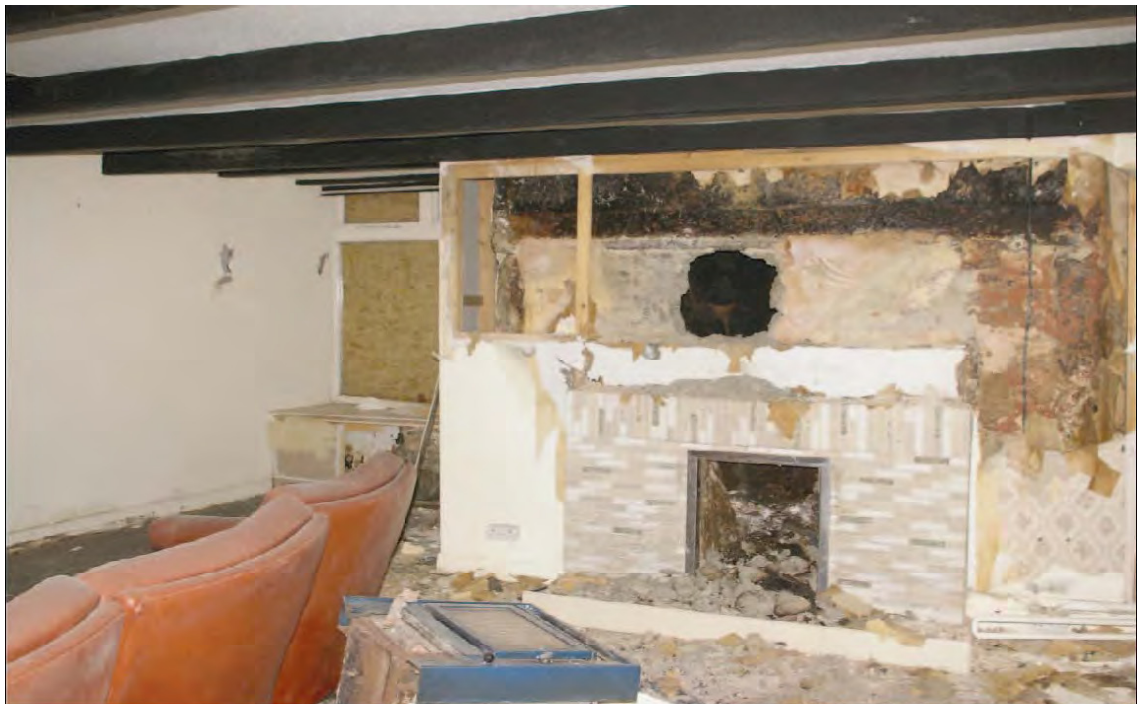
Figure 13: Room 3 viewed from the west showing, the fireplace and hall window.
