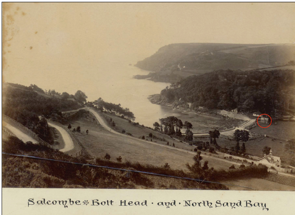
Plate 2: Salcombe, Bolt Head and North Sands bay (undated). Cable Cottage is circled in red. (P4116bd - Cookworthy Museum).
