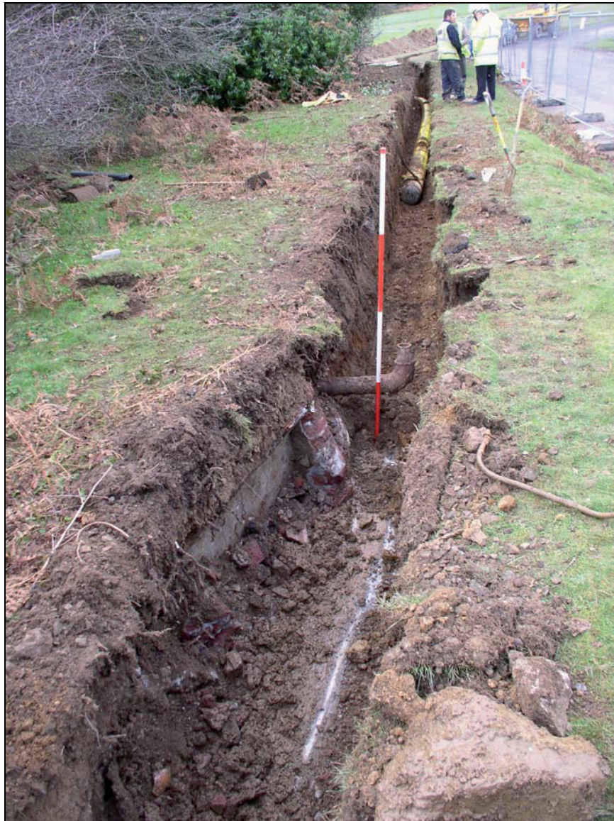
Fig. 7: Brick structure with associated pipework (Fig. 4, location C).
