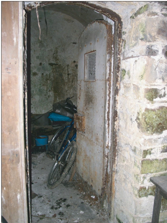
Plate 6: The doorway to cell (5) viewed from the south west.
