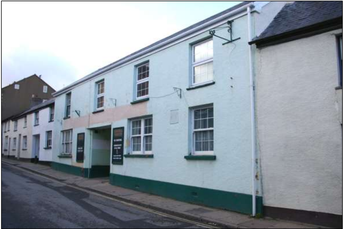
SOUTH ELEVATION, OBLIQUE; VIEWED FROM THE SOUTH-EAST.
