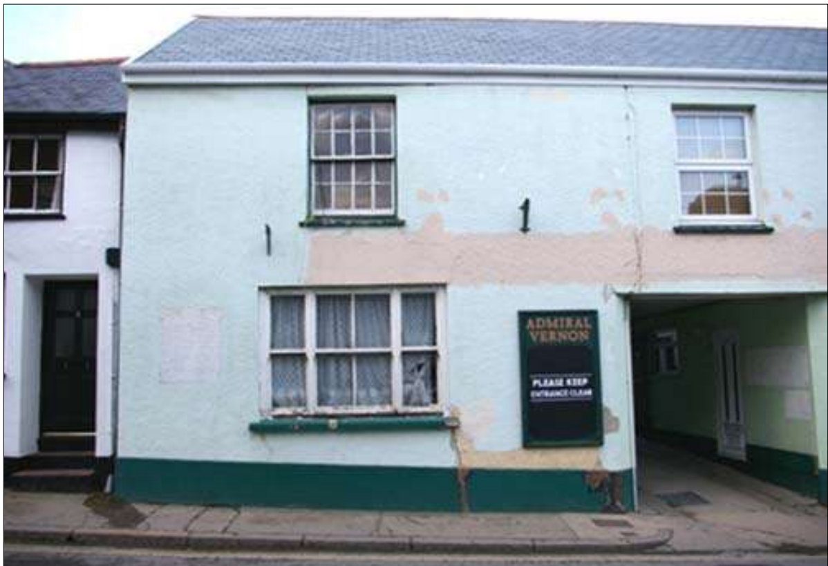
SOUTH ELEVATION, SHOWING HORNED SASH WINDOW TO GROUND FLOOR, AND HORNLESS SASH TO FIRST FLOOR; VIEWED FROM THE SOUTH.
