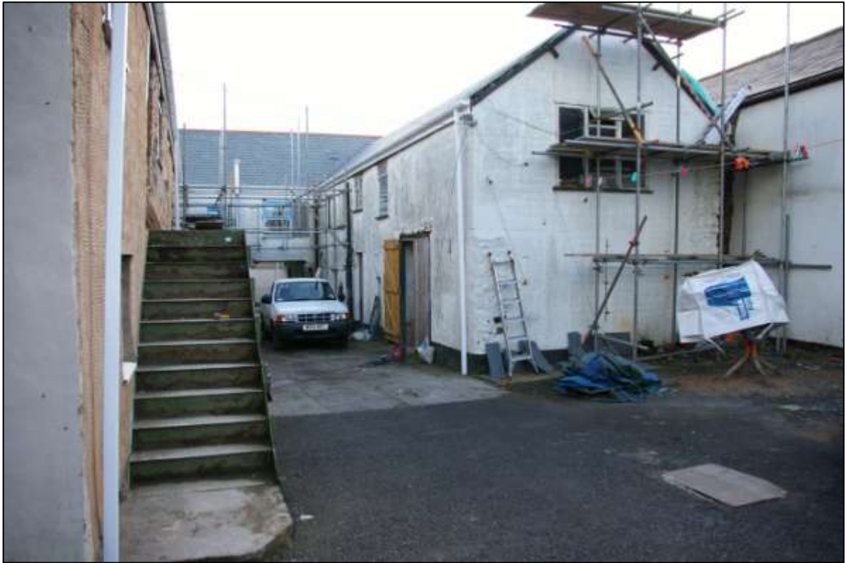
NORTH ELEVATION OF WEST WING; VIEWED FROM THE NORTH-EAST.
