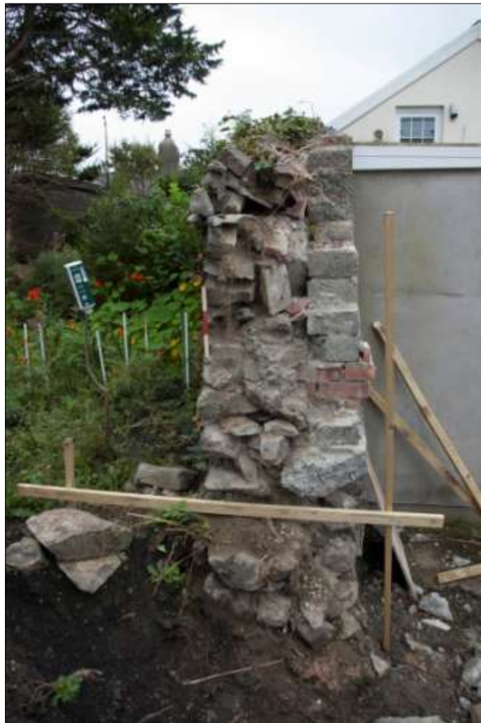
FIGURE 18: WALL {004}, NORTH FACING PROFILE WITH MODERN RETAINING/REPAIR {014}; VIEWED FROM THE NORTH (0.30M SCALE).
