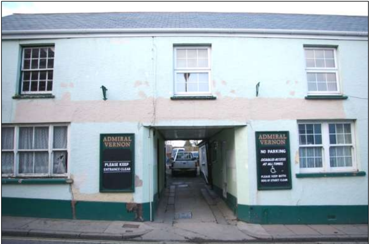
Figure 11: SOUTH ELEVATION, SHOWING THE OFF-CENTRE OPENING WITH SPLAYS TO THE ROAD; VIEWED FROM THE SOUTH.
