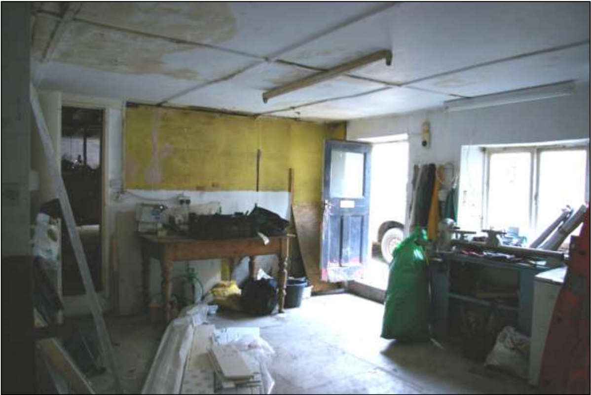
INTERNAL NORTH WALL OF GR2; VIEWED FROM THE SOUTH-WEST (NO SCALE).
