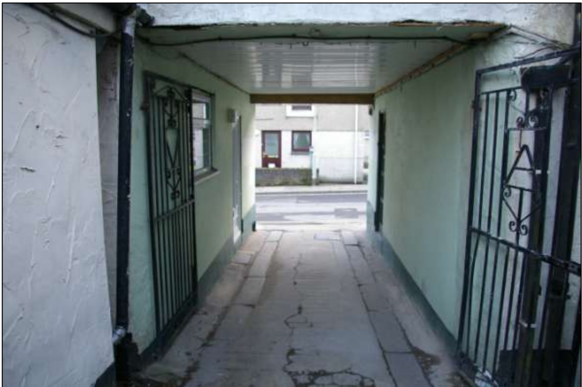
OFF CENTRE OPENING; VIEWED FROM THE NORTH.
