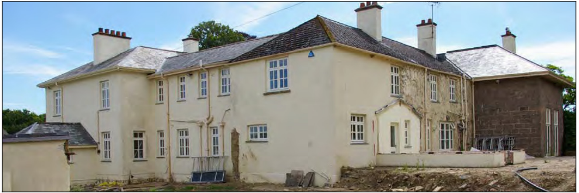
Figure 8: Fishleigh House, the north-west elevation.
