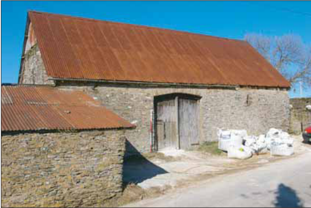
Plate 3: The Threshing Barn (1) viewed from the south.
