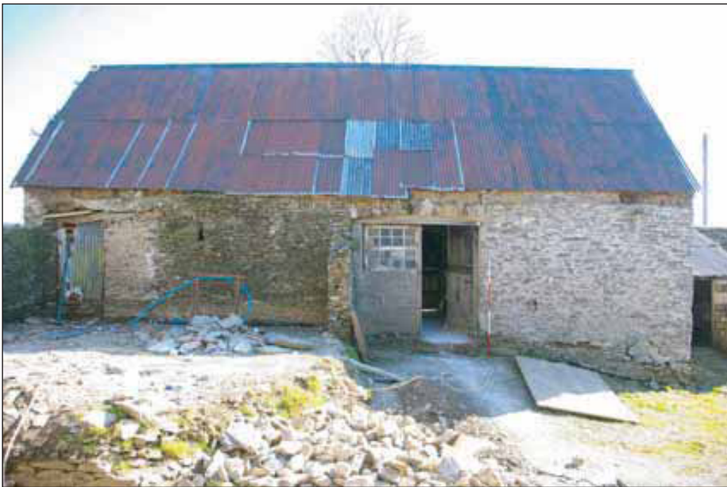
Plate 4: The Threshing Barn (1) viewed from the north.
