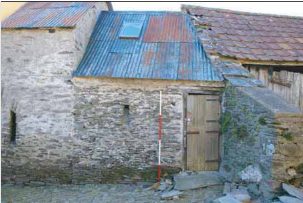
Plate 6: The Infill Building (6) viewed from the west.
