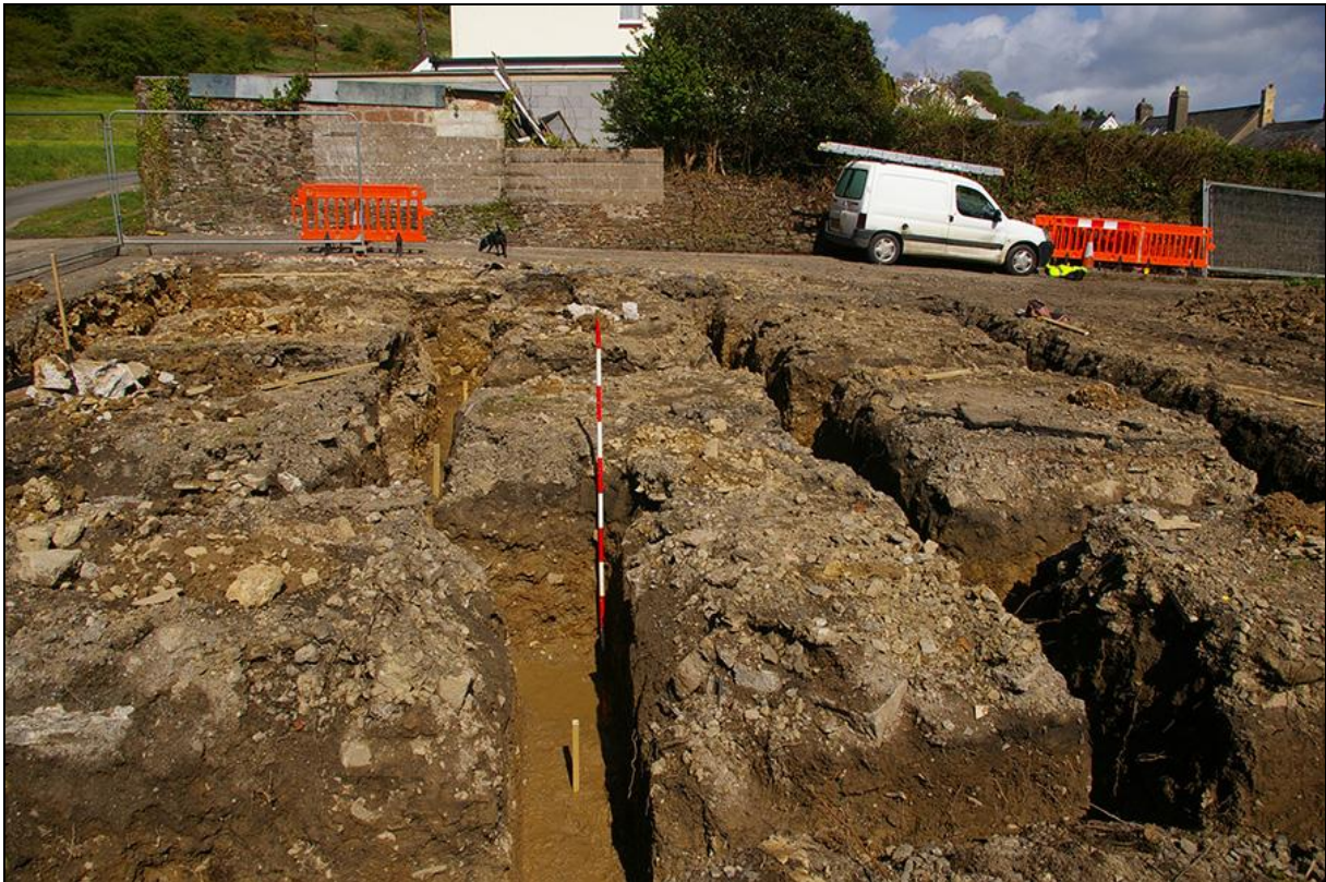
FIGURE 3: EXCAVATED FOOTING TRENCHES; VIEWED FROM THE SOUTH-WEST (2M SCALE).
