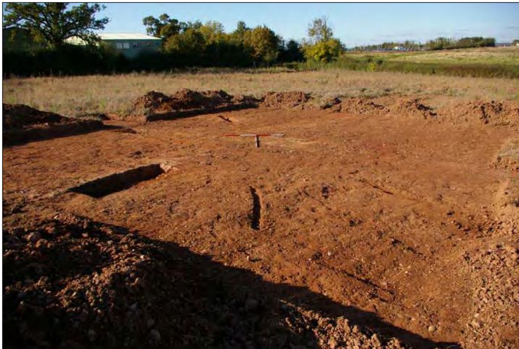
Figure 7: General area shot of Trench #4, viewed from the south east looking north west (scale 2m).
