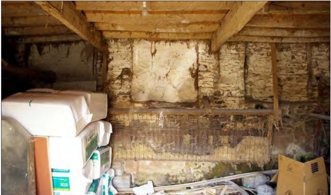
Figure 10: The interior north wall of Shippon no.1 with recessed alcoves for feeding access.
