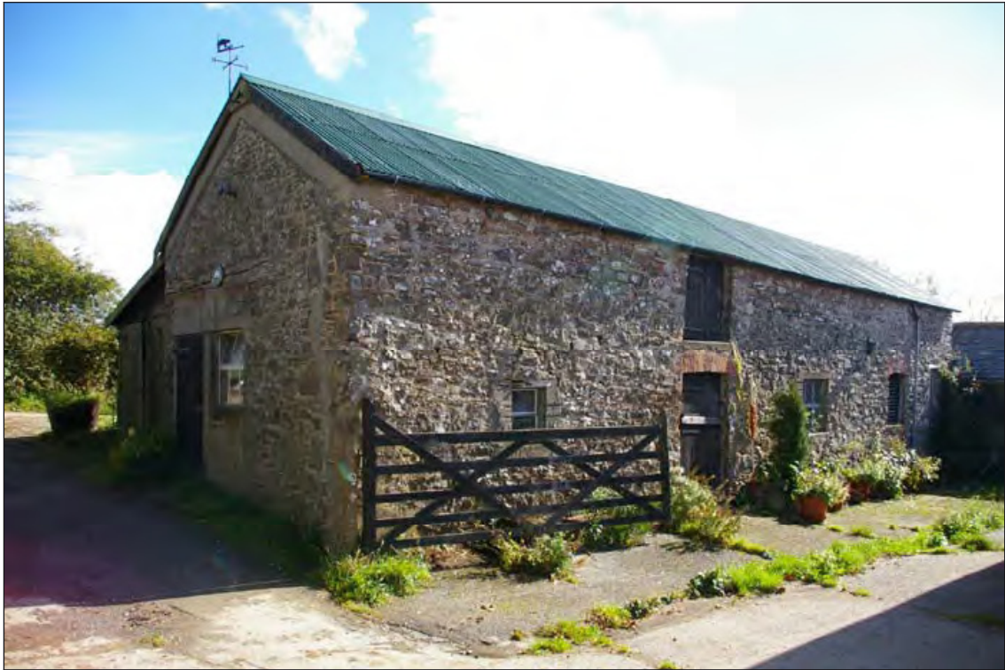
Figure 11: The north and west elevations of Shippon no.2, viewed from the north-west (2m scale).
