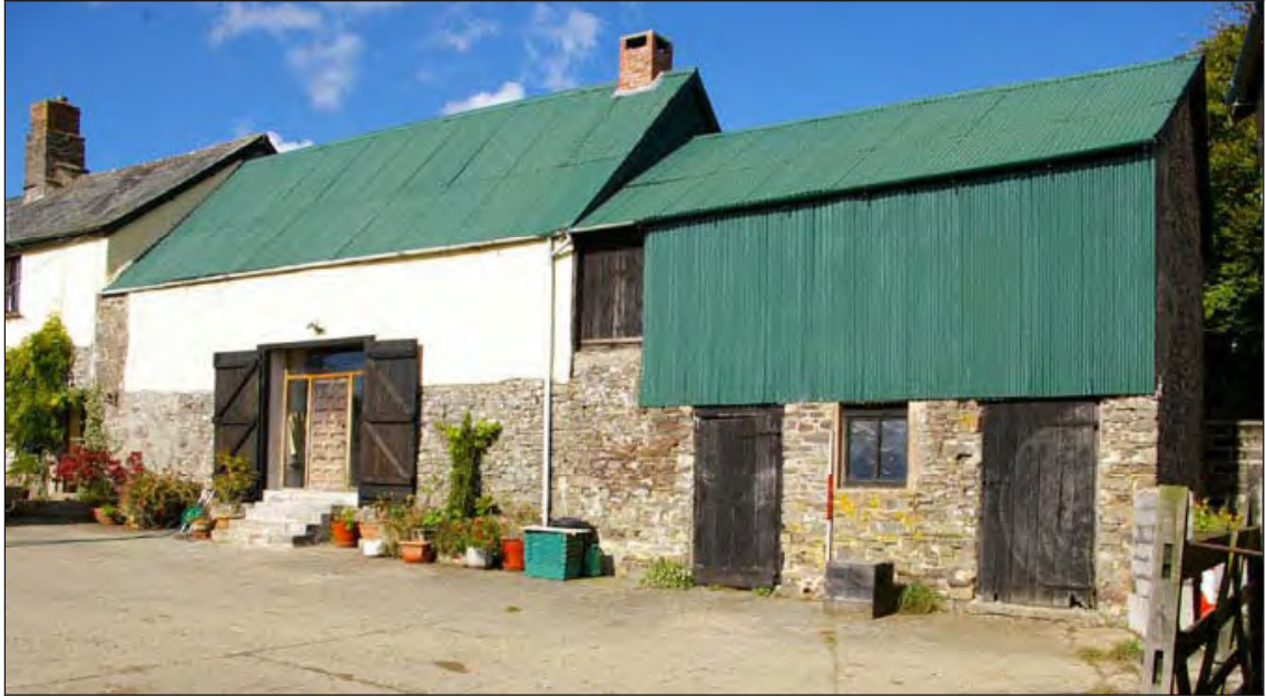
Figure 8: The south elevation of the parallel range; Threshing Barn and Shippon No. 1, viewed from the south-east (2m scale).
