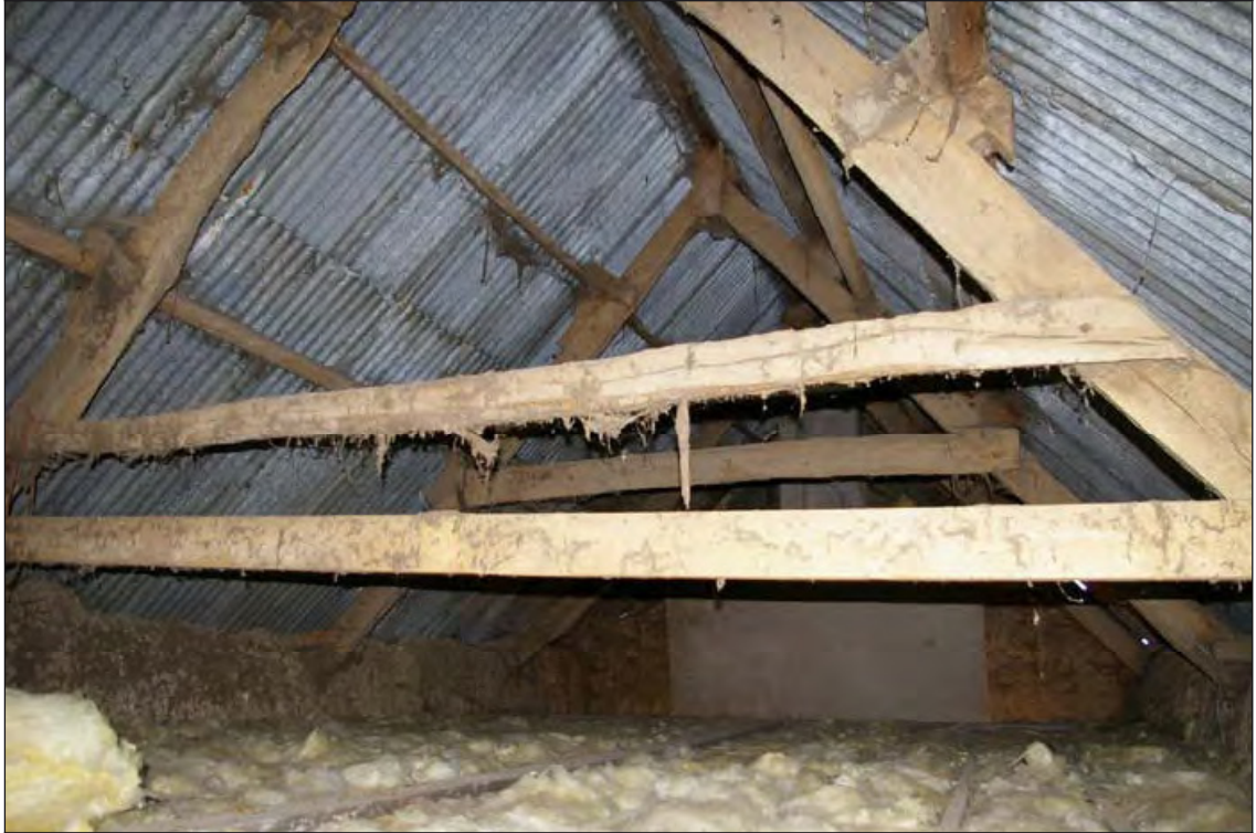
Figure 9: The roof structure of the threshing barn , viewed from the south-west.
