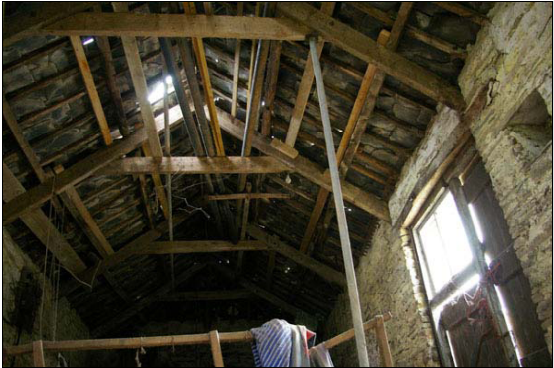
Figure 11: Roof structure, viewed from the east.
