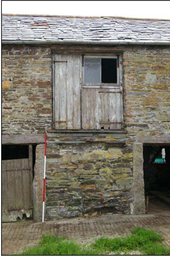
Figure 10: The central section of the north elevation (scale 2m).
