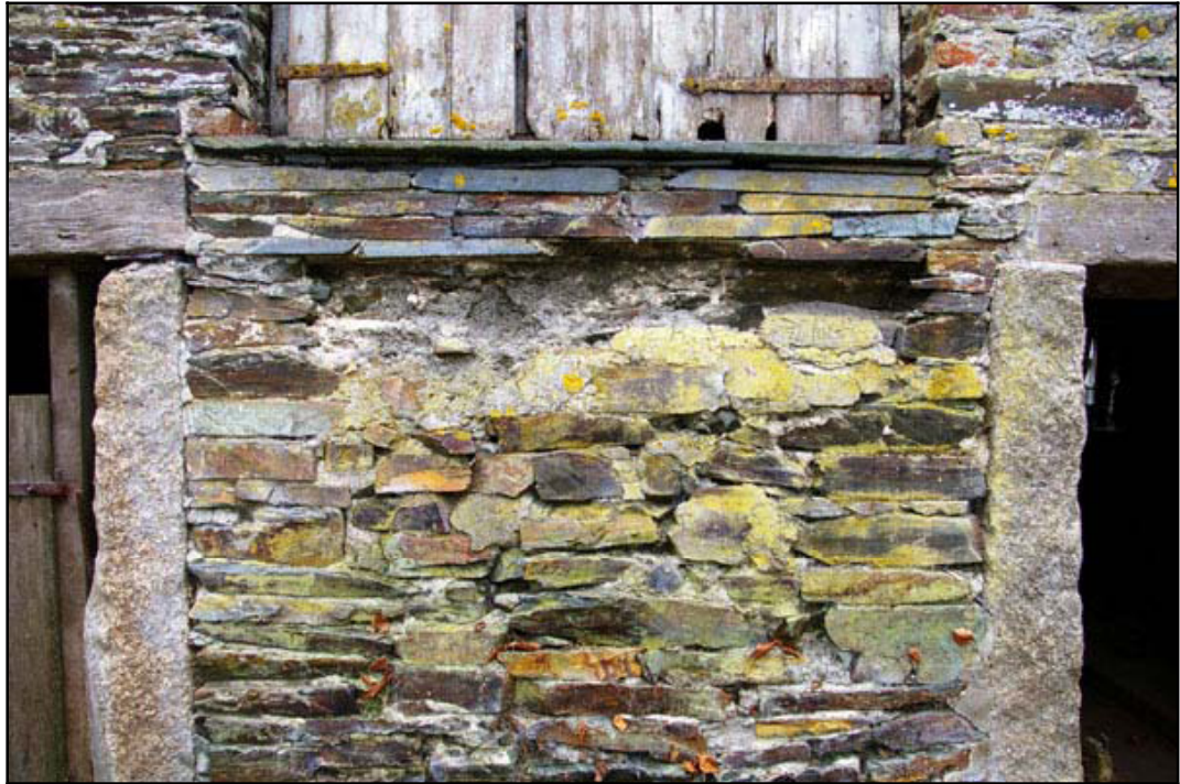
Figure 9: Granite posts flanking the ground floor openings in the north elevation.
