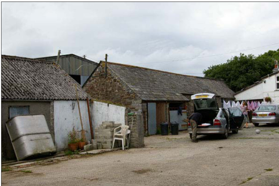
Figure 2: The farmyard, with the single-storey barns and farmhouse, viewed from the south-east.
