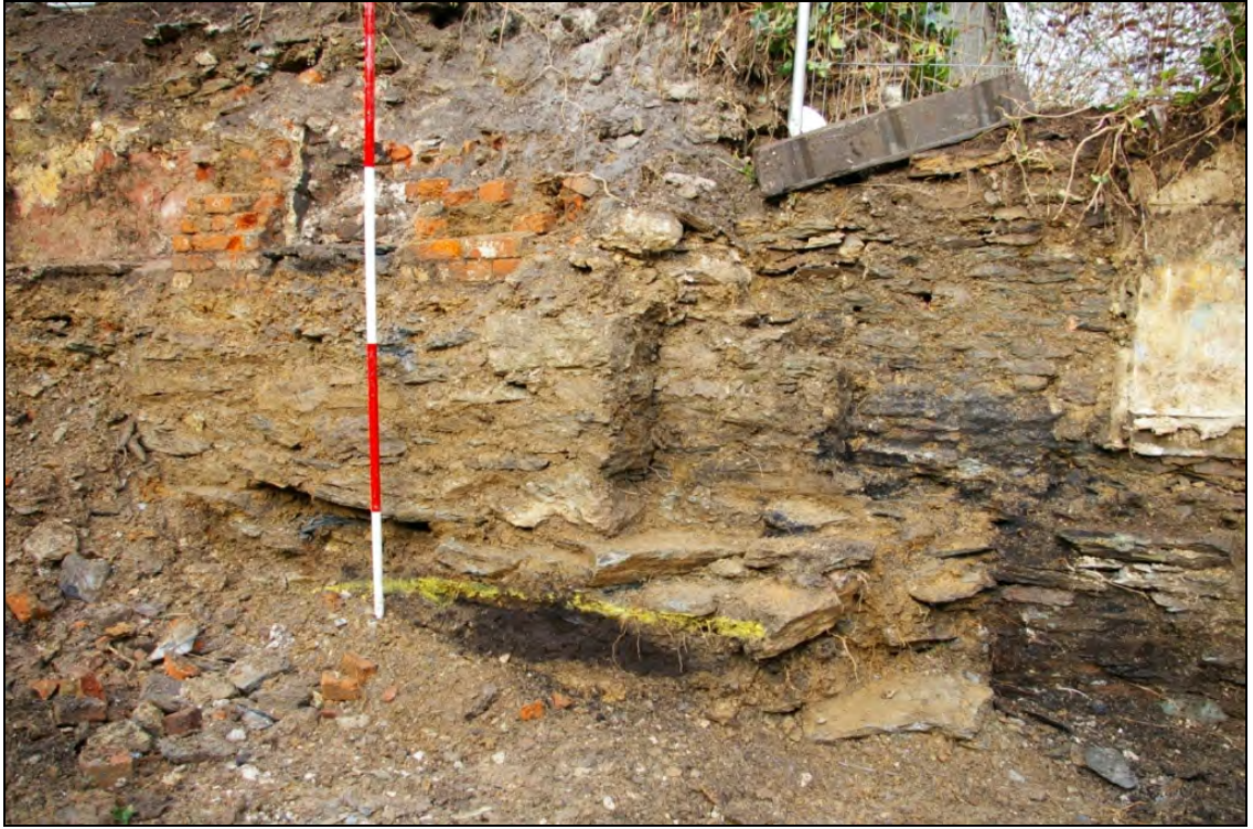
Figure 20: The dwarf wall in the north-east corner of Building 9, viewed from the east (2m scale).
