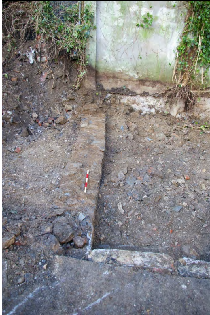
Figure 21: The east elevation of Building 10, viewed from the south-east with the modern storage building in the background (0.5m scale).
