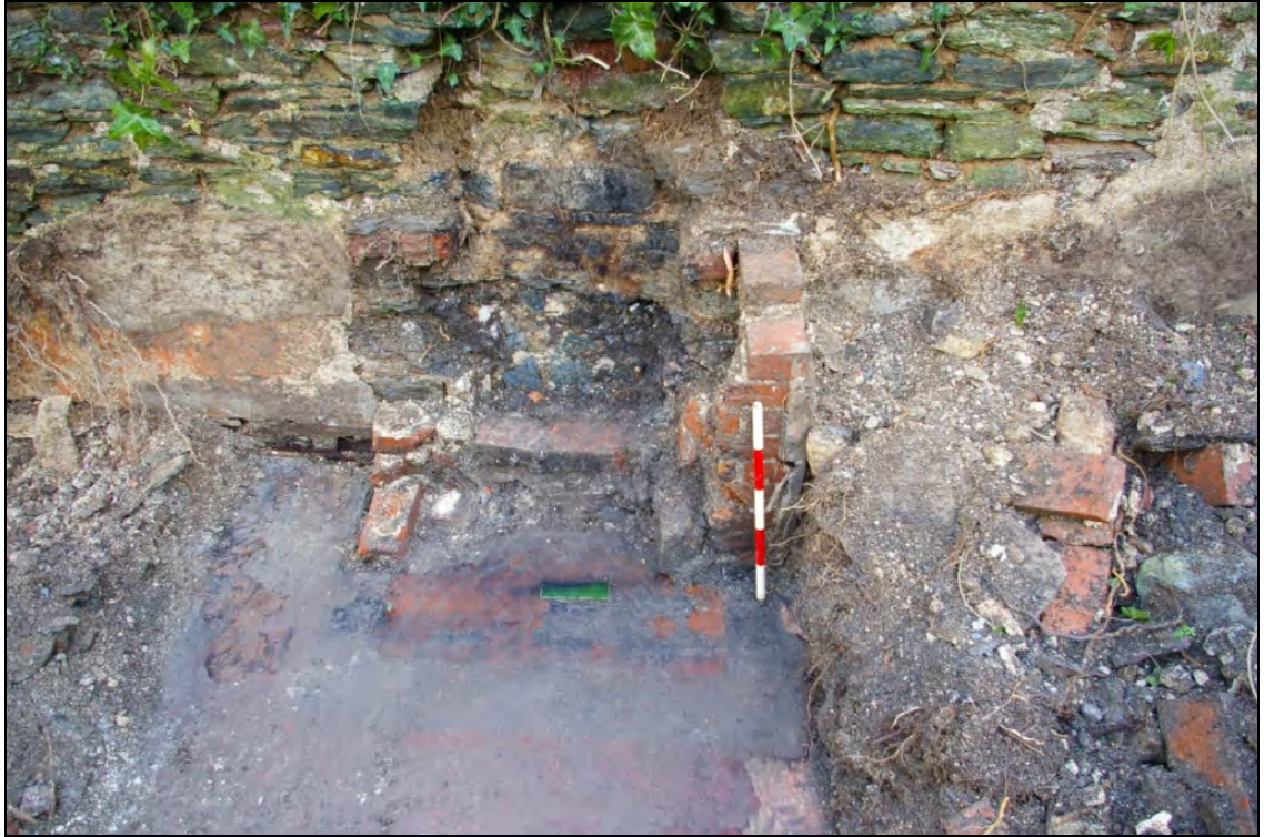
Figure 5: The fireplace inserted into the southern elevation of Building 2, viewed from the north-east (0.5m scale).
