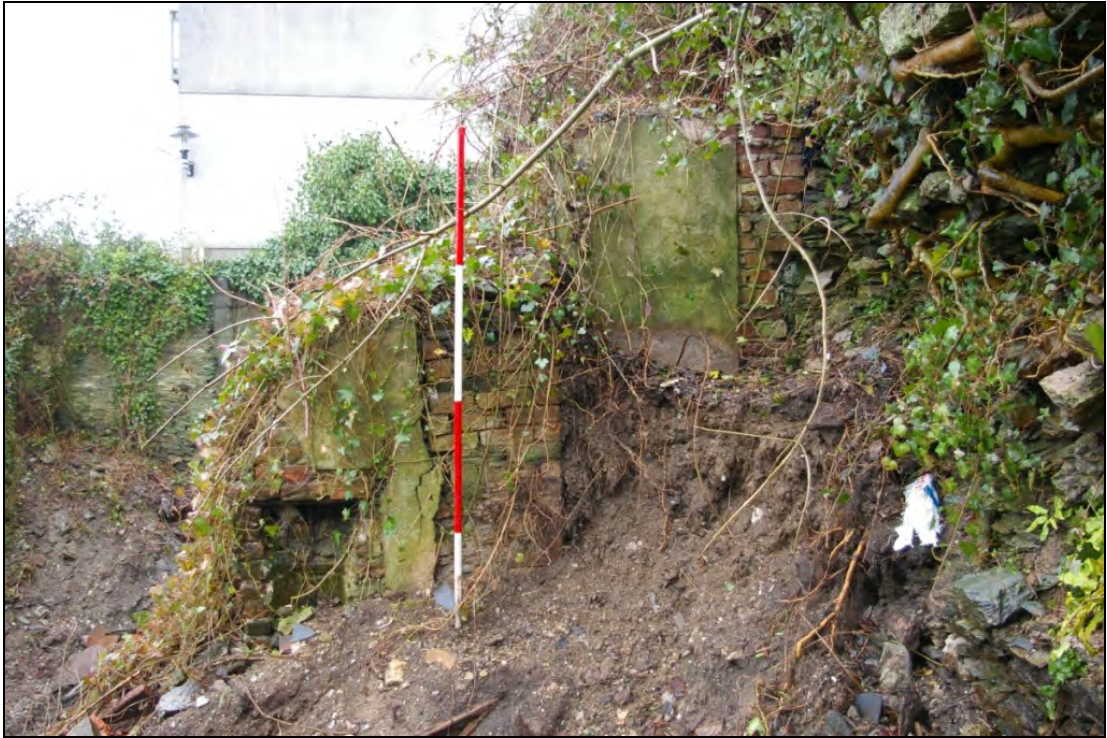
Figure 15: North face of Elevation 6, viewed from inside Building 7 (2m scale).
