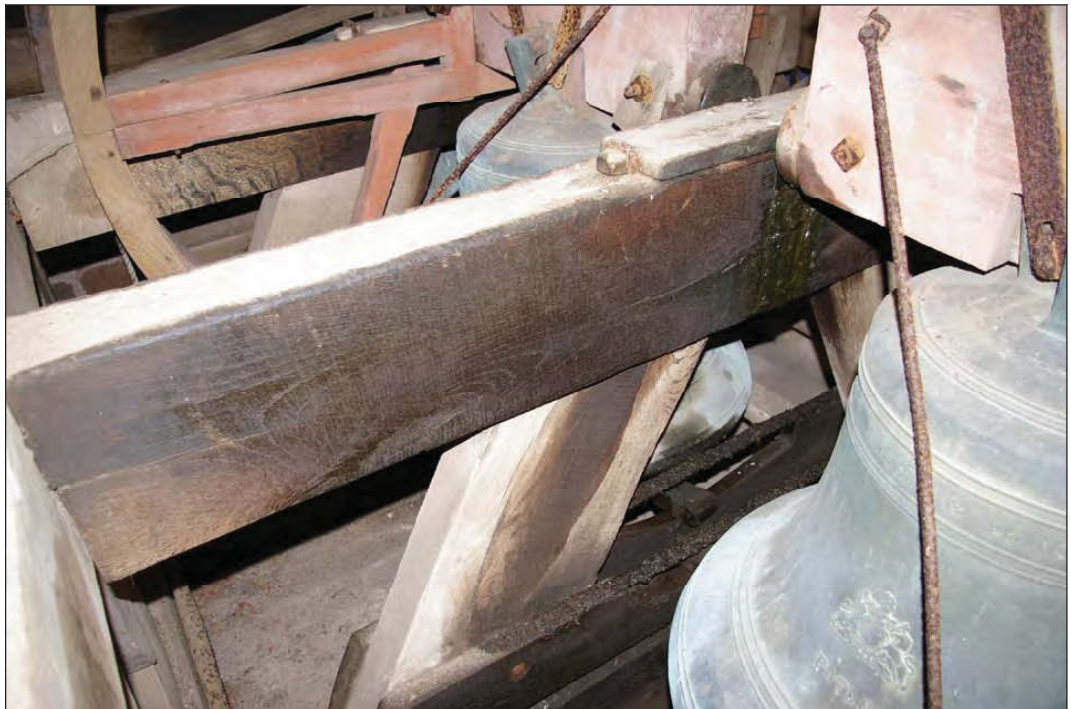
Figure 8: Detail of the truss on the north side of bellpit 3.
