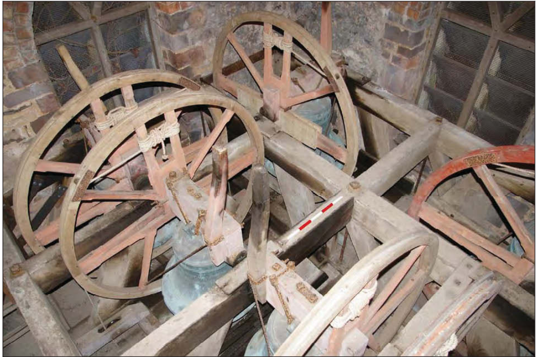
Figure 13: The bell frame, viewed from the north-east (scale 0.5m).
