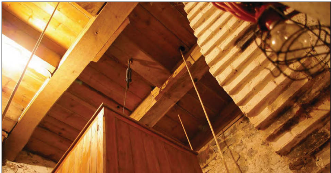
Figure 7: The floor of the belfry, viewed from below and the north-east.
