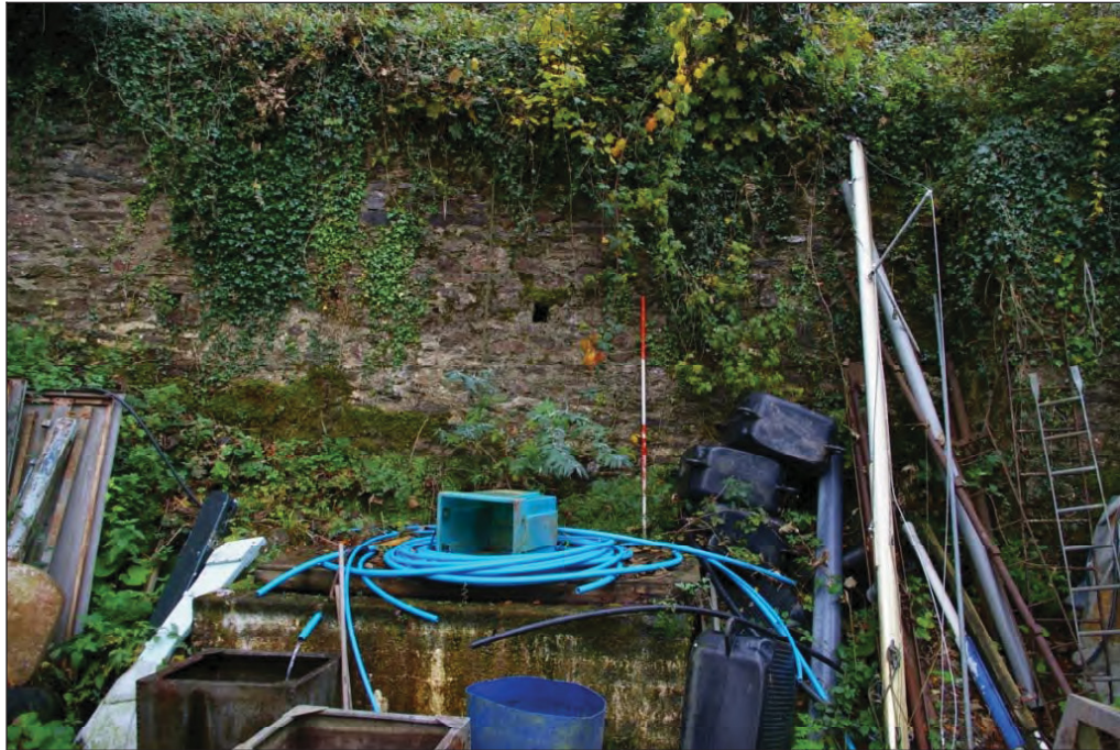
Figure 13: The surviving southern wall of the former cottages (2m scale).
