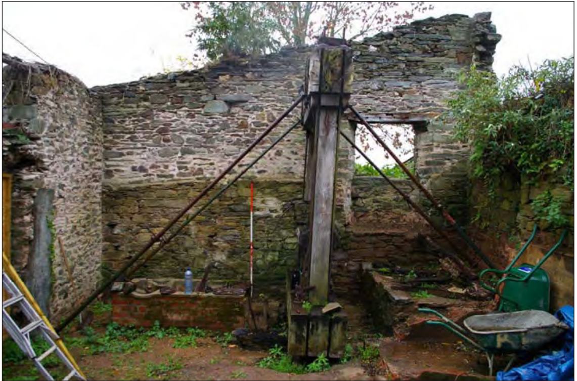
Figure 10: The eastern half of the interior, viewed from the west. The contrast between the Phase 1 and Phase 2 build is clearly visible (scale 2m).
