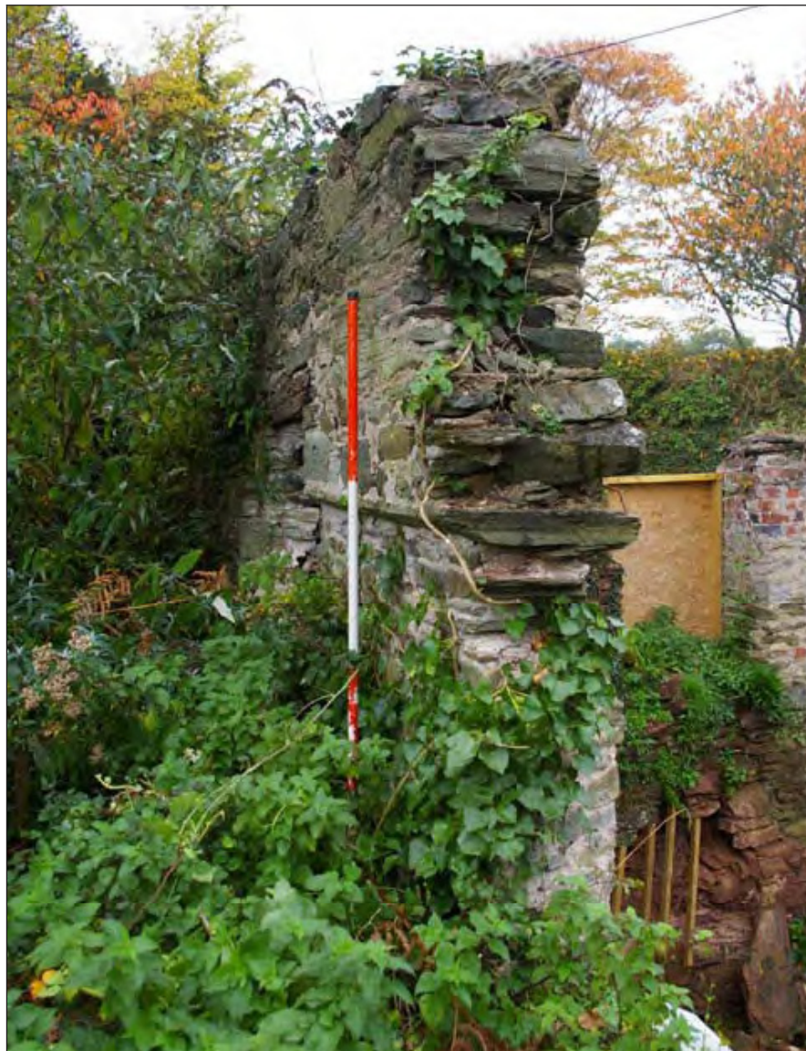
Figure 9: Surviving splay of window (W5) and projecting chamfered string course, viewed from the east (scale 2m).
