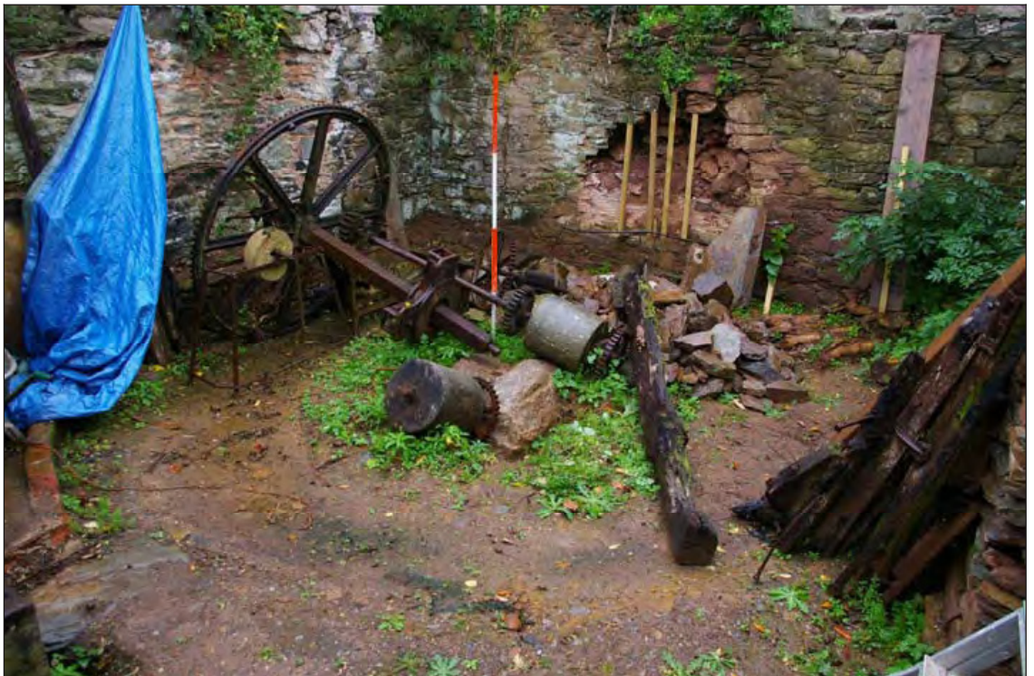
Figure 11: The western half of the interior, viewed from the north-east. The groove worn into the floor around the horse engine is clearly visible (scale 2m).
