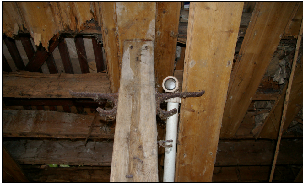
Figure 9: The hooks to the front of the dividing partition within B2.
