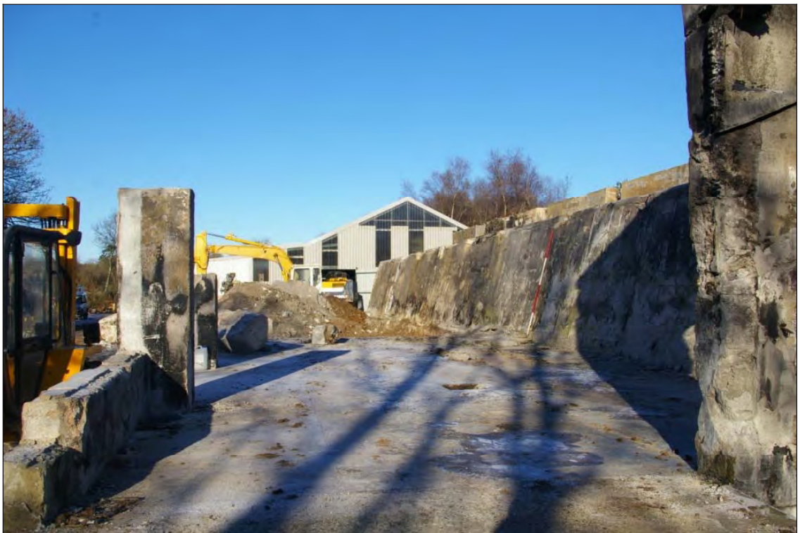
Figure 11: Phase 2 linhay, viewed from the south-east (Scale: 2m).
