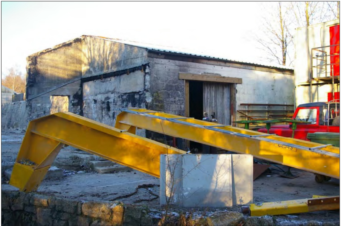
Figure 15: Phase 2 furnace house, viewed from the south (Scale: 2m).
