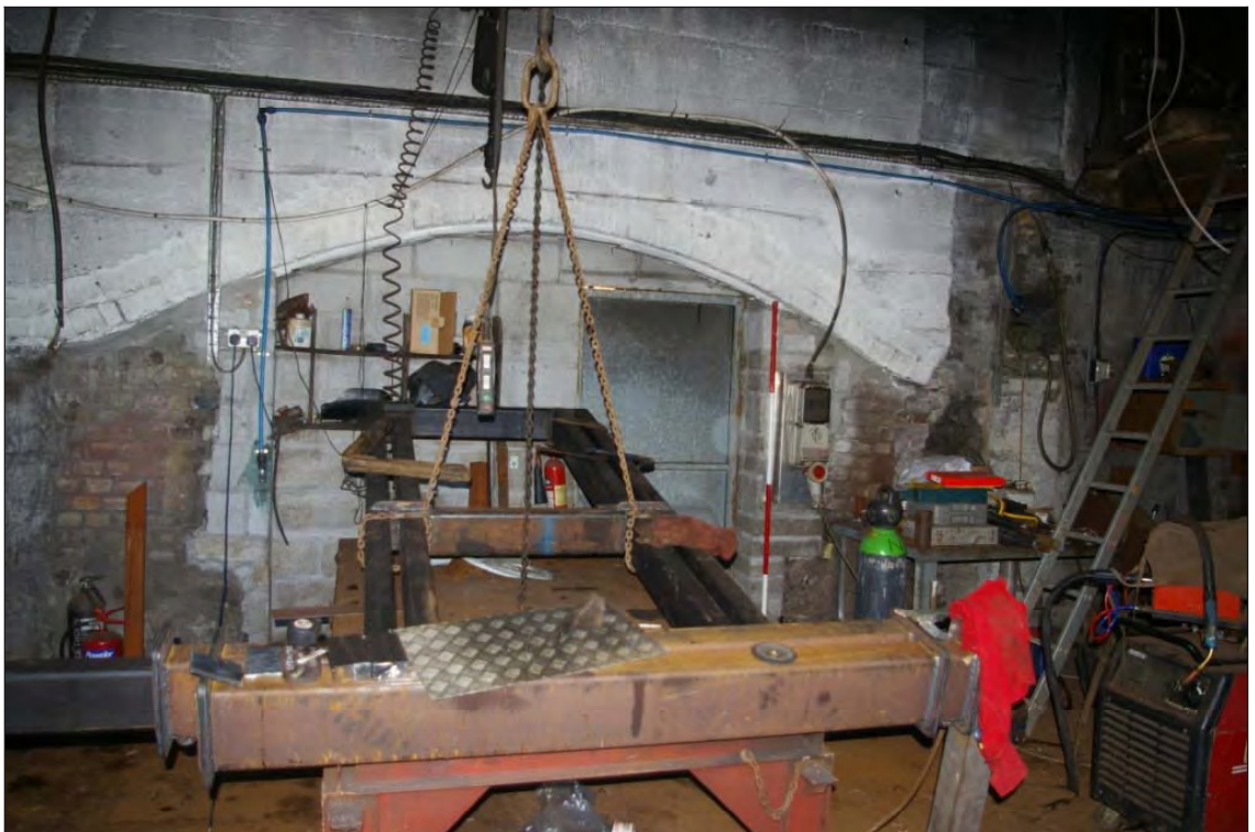
Figure 16: Archway through the north-western wall of the furnace house, viewed from the south (Scale:2m).
