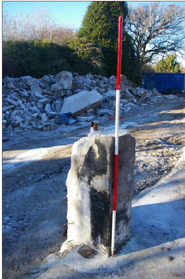
Figure 12: Concrete pillar on the south-western side of Phase 2 linhay, viewed from the south-east (Scale: 2m).
