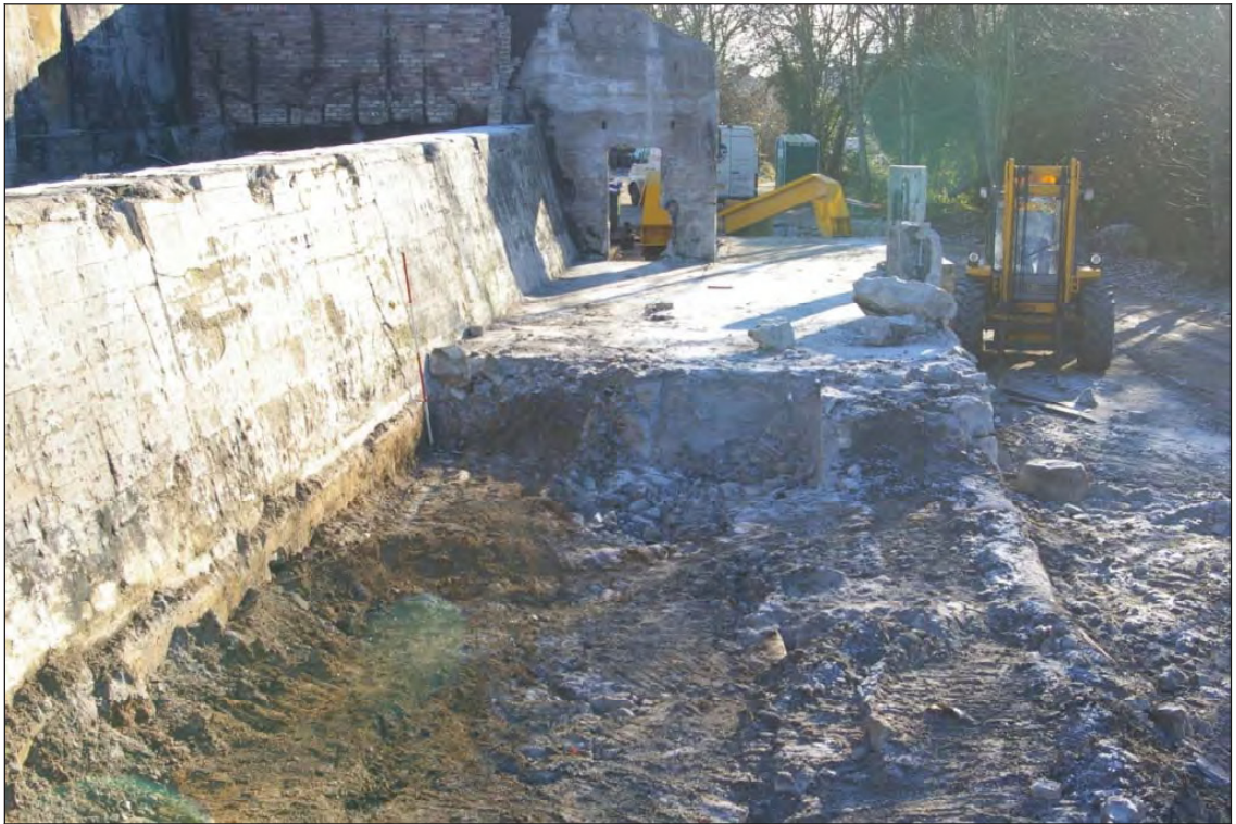
Figure 10: Phase 2 linhay, viewed from the north west, the three compartment construction is clearly visible (Scale: 2m).
