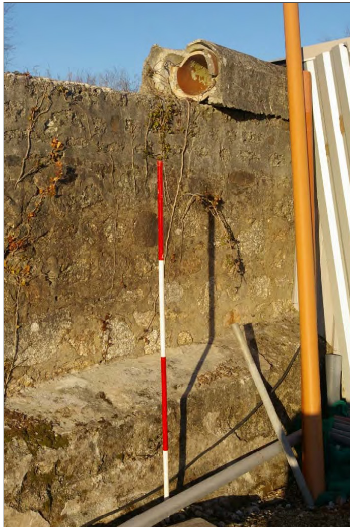
Figure 3: Clay slurry pipe on the wall between settling tanks 6 and 7 (see Fig. 2), viewed from the south-east (Scale: 2m).
