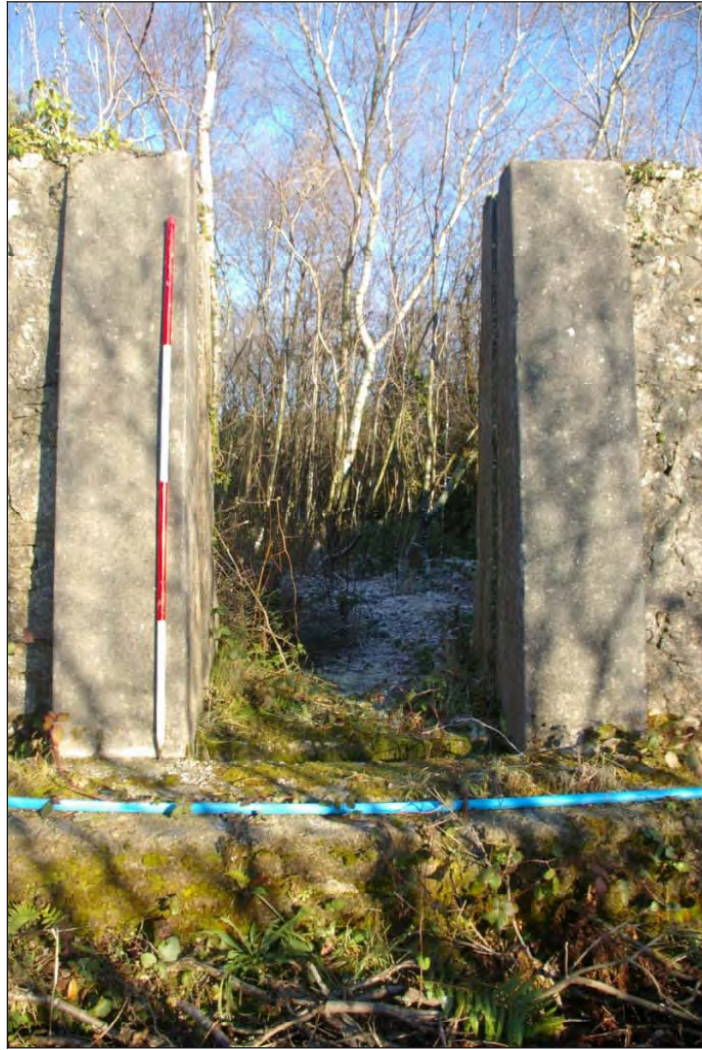
Figure 4: Entrance to settling tank 3 (see Fig. 2), viewed from the south-west (Scale: 2m).
