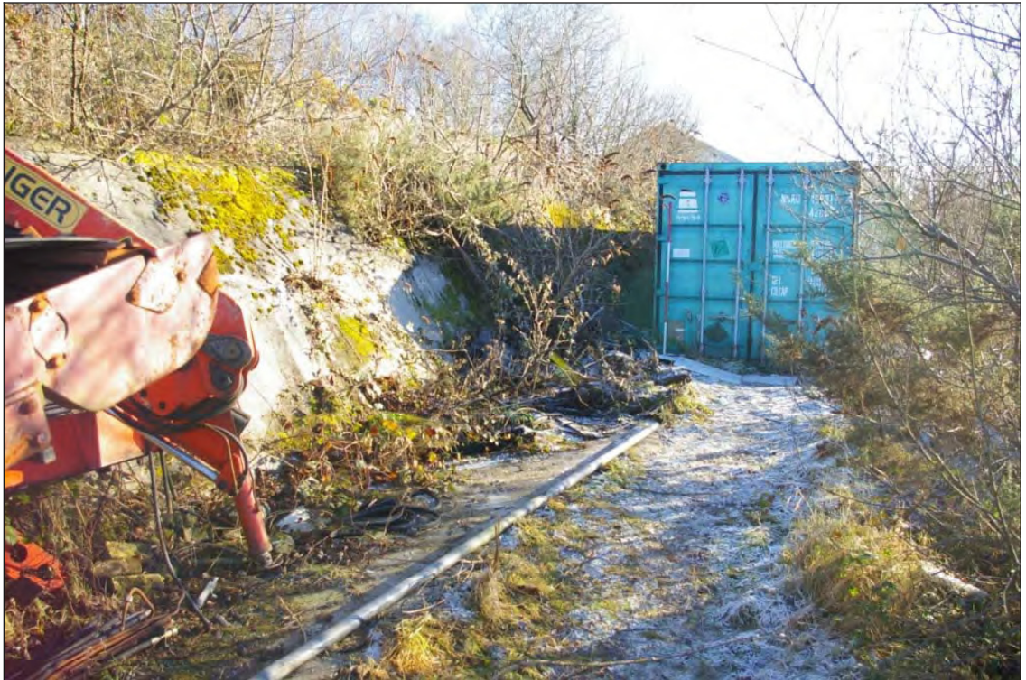
Figure 7: Phase 1 linhay, viewed from the north-west (Scale 2m).
