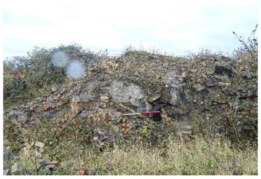
Figure 19: Side of Blast Furnace base showing tuyere inlet for blast
