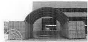
Figure 1 - Shipping Container Car Port
