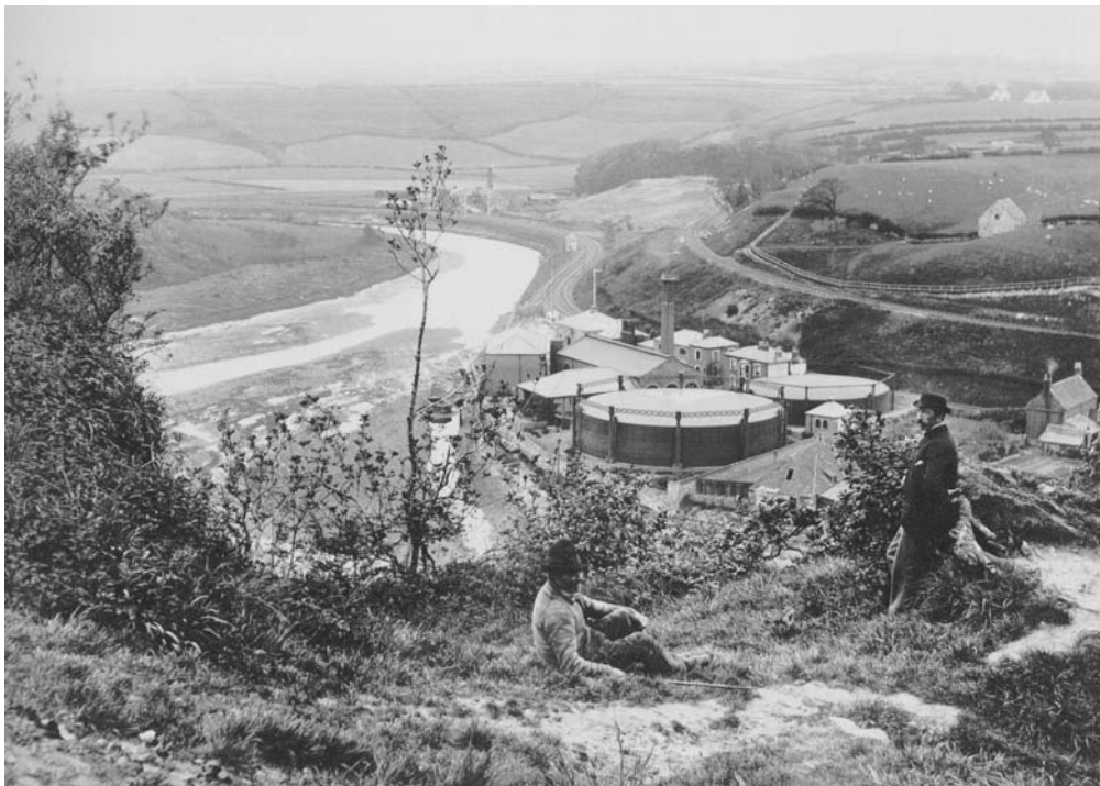
Figure 9.6. Gas works, River Esk (© Sutcliffe Gallery ( www.sutcliffe-gallery.co.uk ))
