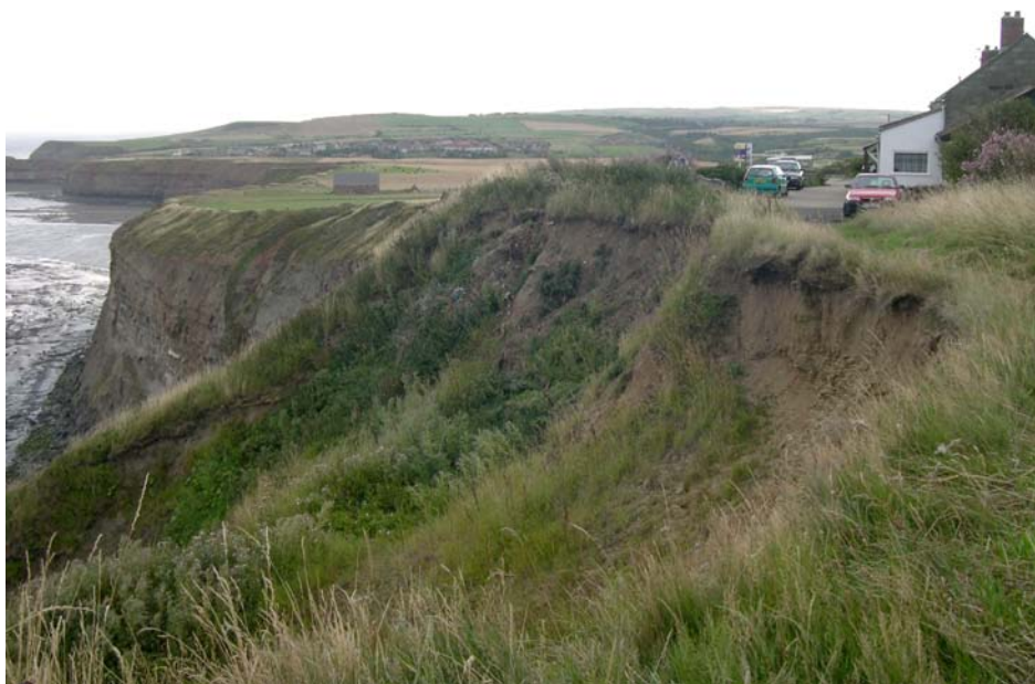
Figure 9.50. Cliff erosion at Boulby
