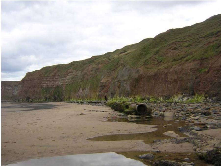
Figure 9.13. Disused sewage pipeline on the foreshore at Saltburn
