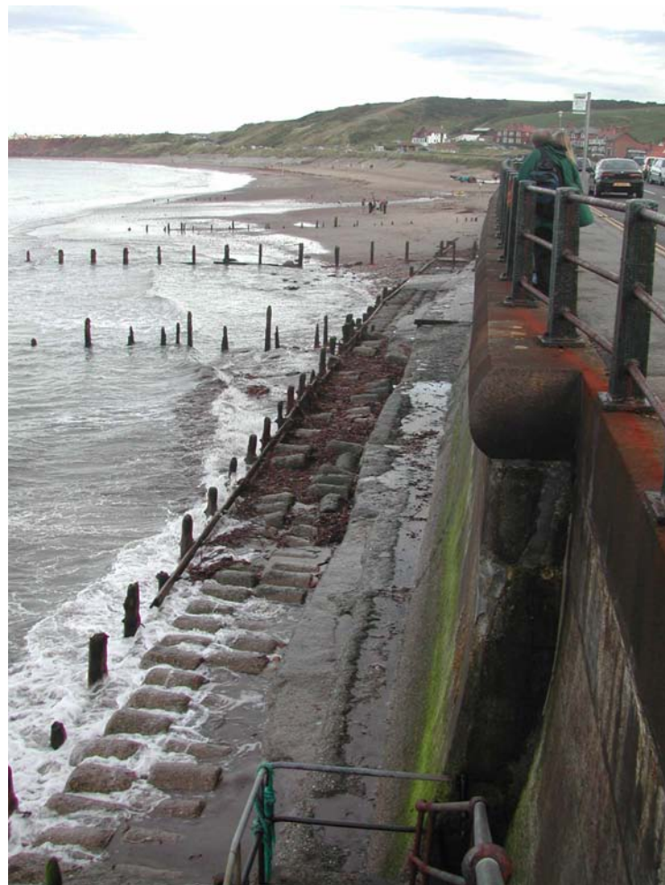
Figure 9.68. Anti-tank defences now incorporated into the sea wall at Sandsend
