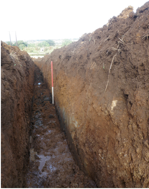
Plate 10 – Section 8, looking northwest
