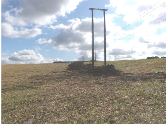
Plate 1 – View looking southeast along the cable route
