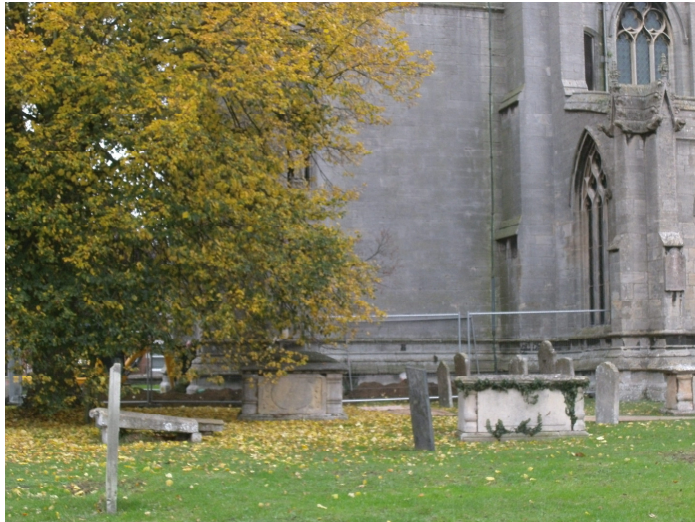
Plate 1 – General view of the west end of St Andrew's church showing the area of works, looking northeast
