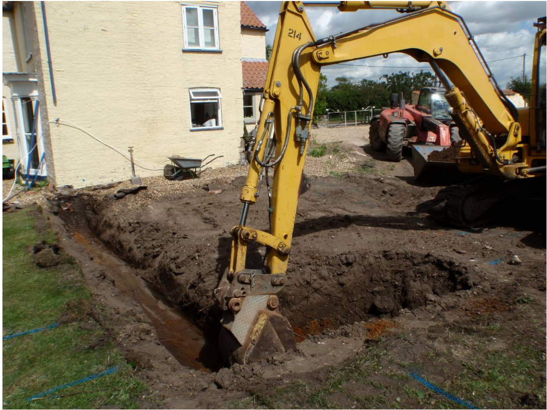
Plate 5. Excavating the house extension footings looking north
