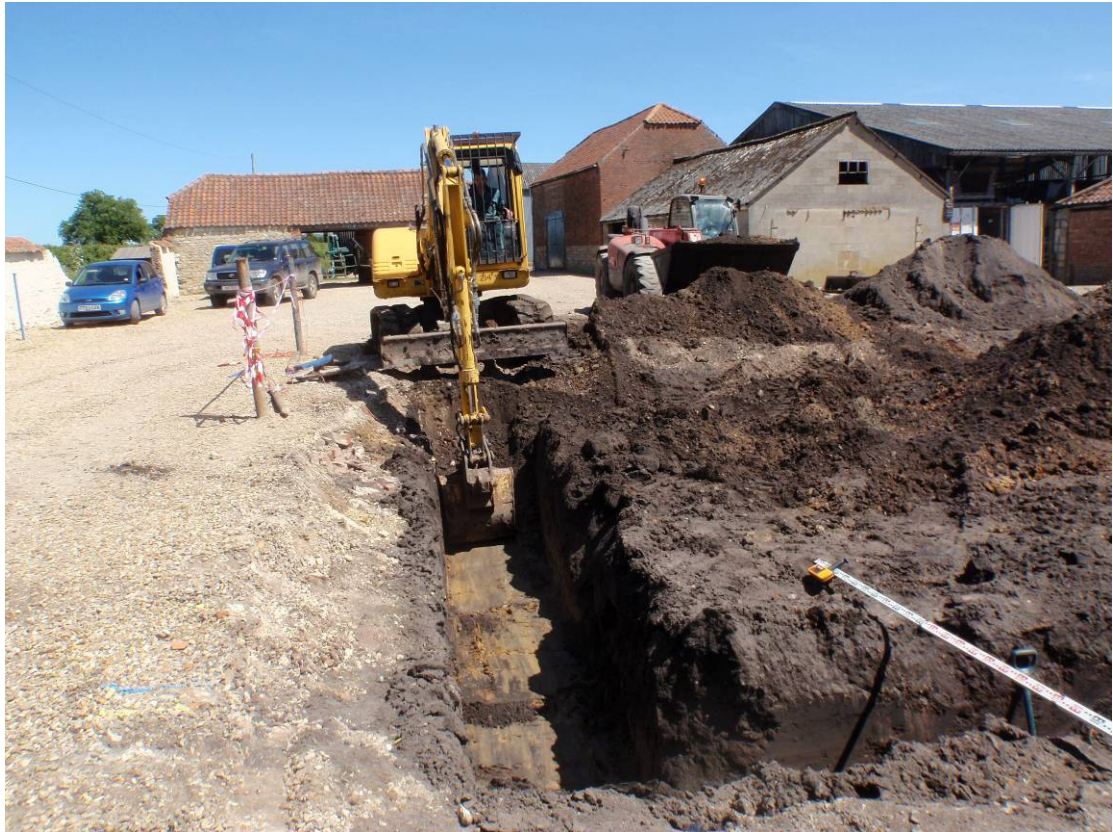
Plate 1. Excavating the barn footings looking east
