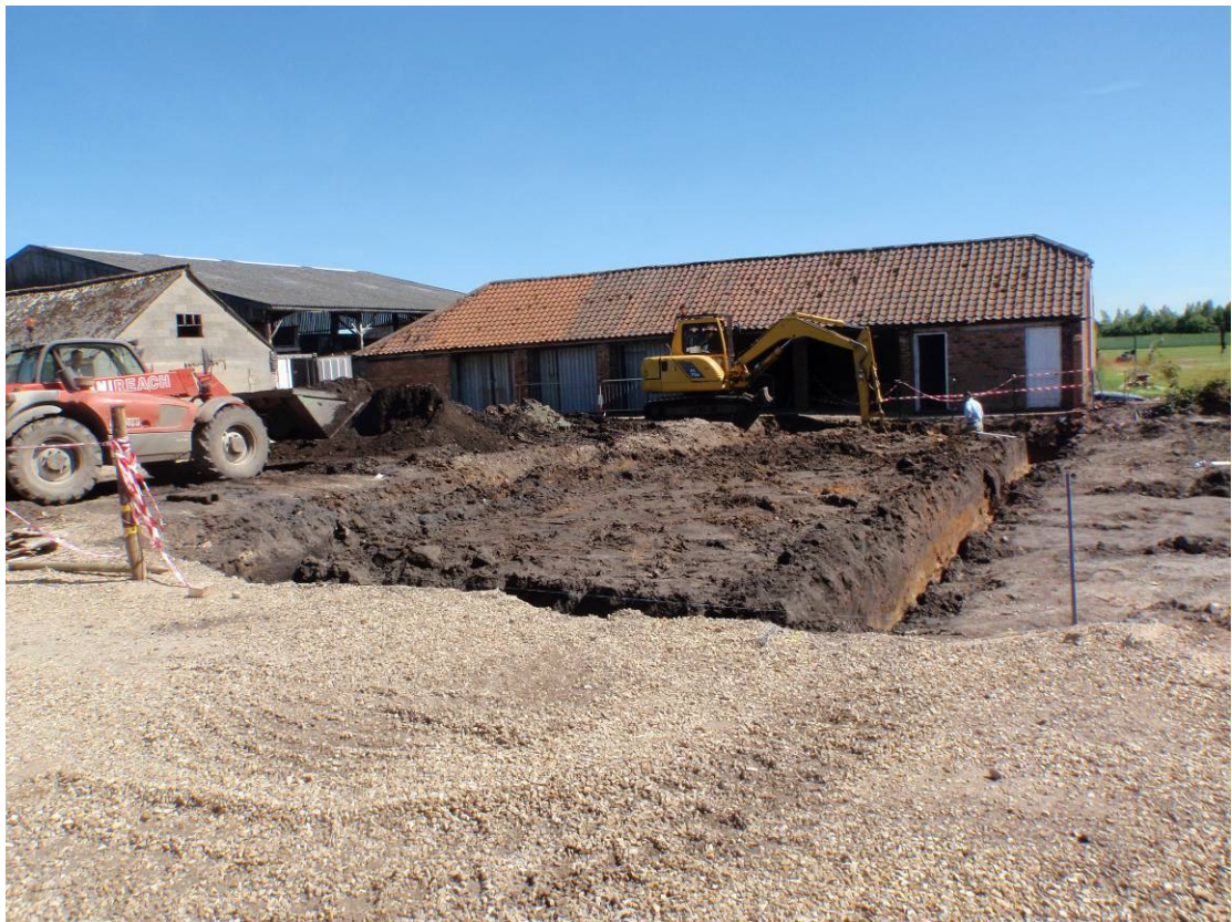
Plate 4. Completed barn footings looking south
