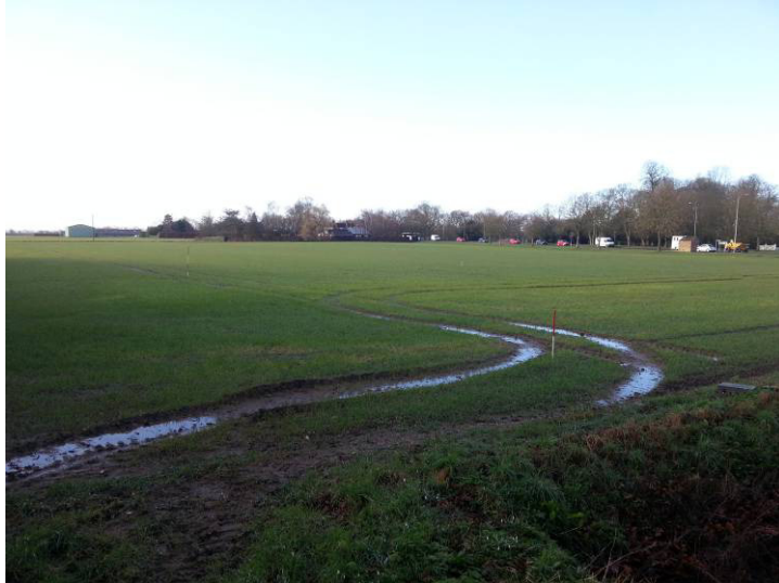
Plate 1 – General view of site
