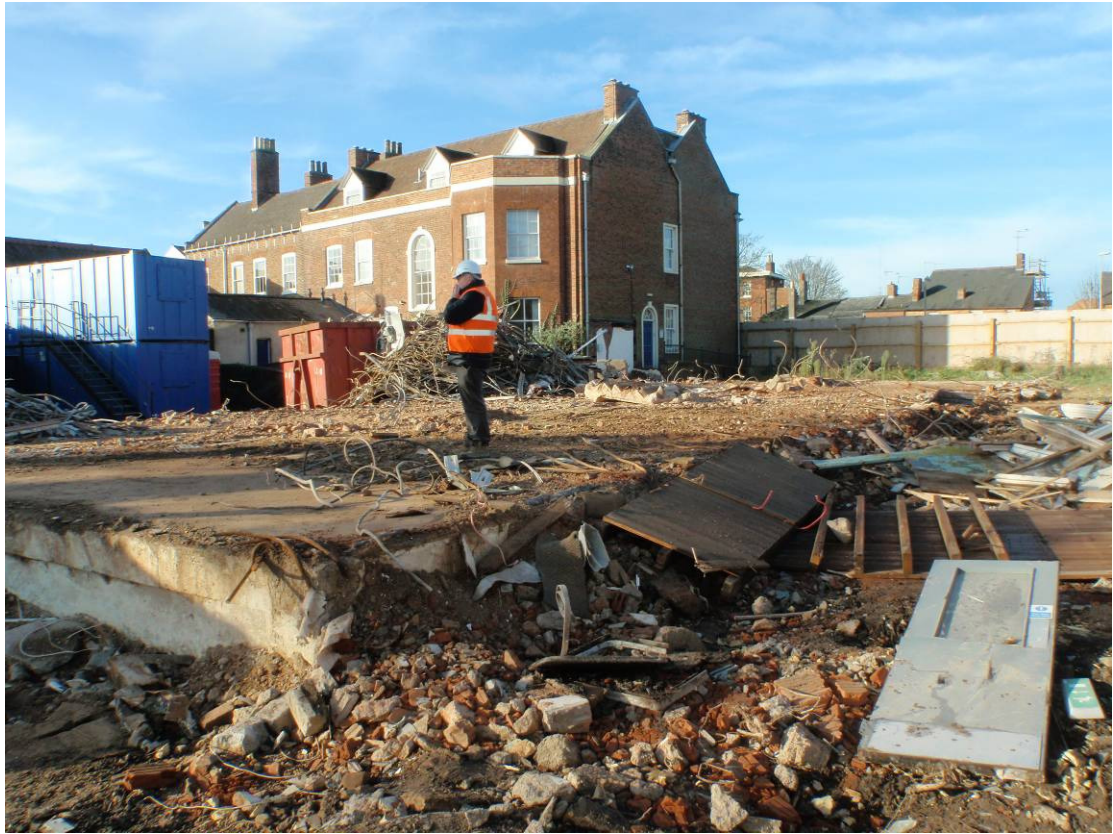
Plate 1. Pre-machining view of site looking northwest
