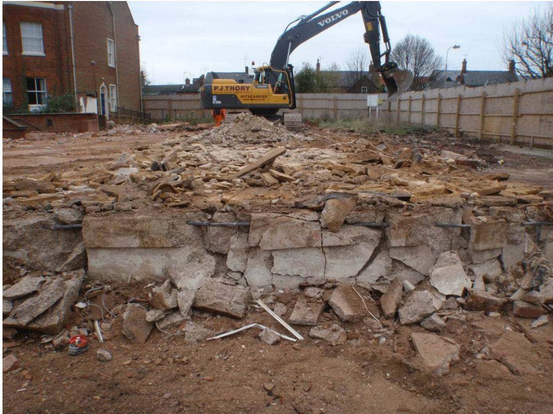
Plate 3. Breaking the thick reinforced concrete looking northwest
