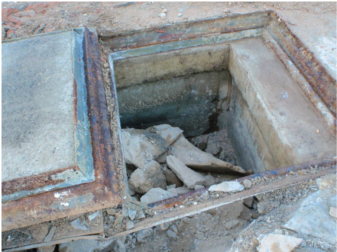
Plate 2. View showing thickness of concrete slab in side of manhole
