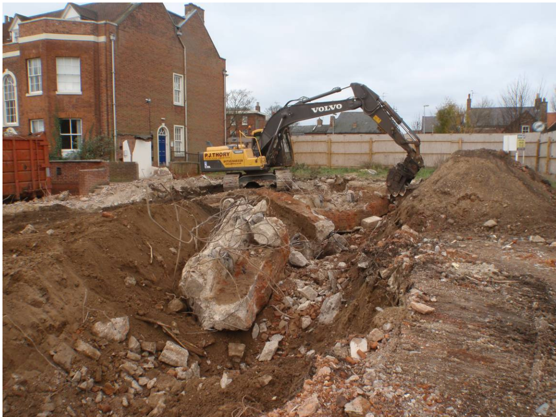
Plate 4. Removing concrete foundations looking northwest
